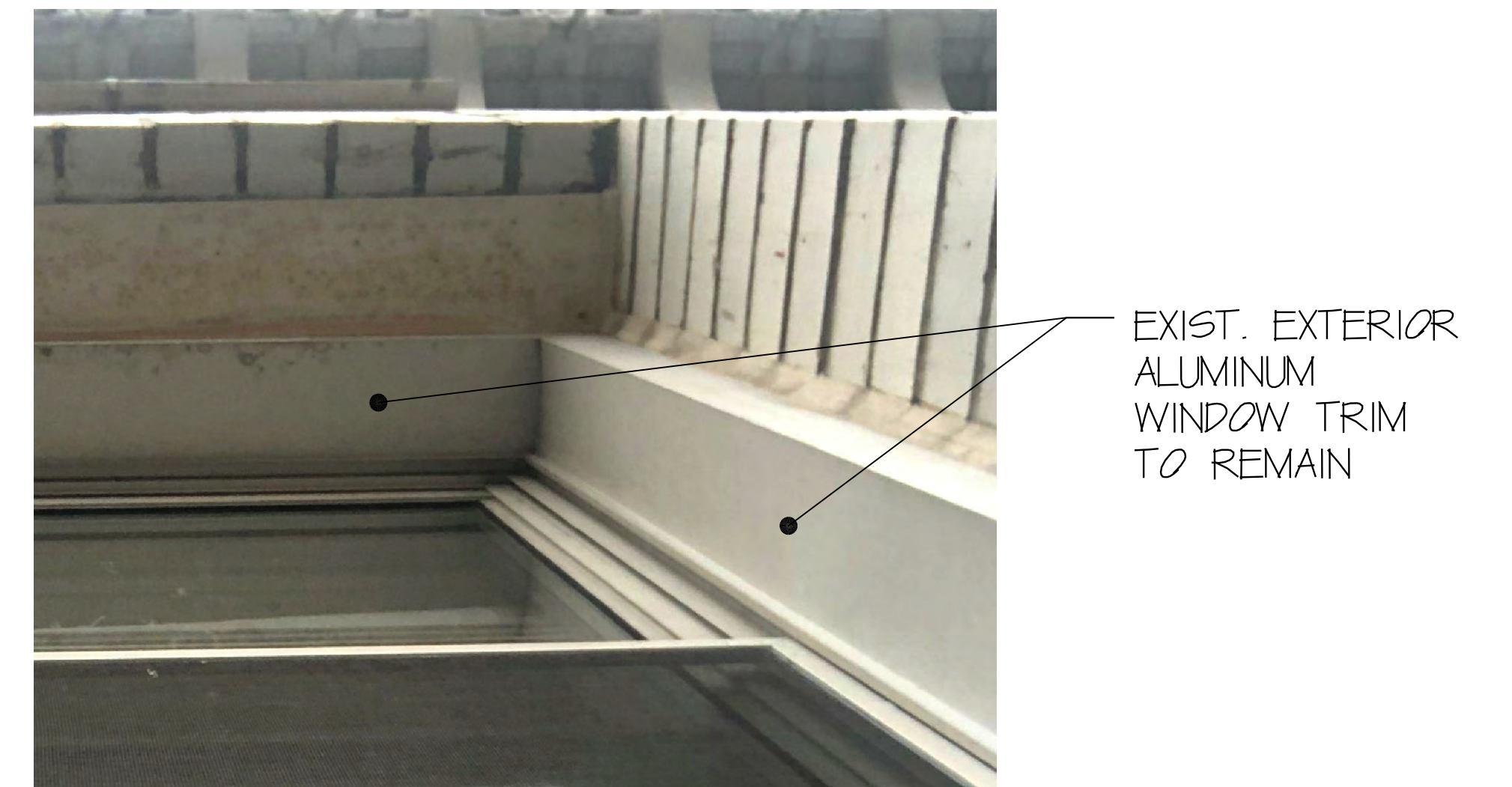
PHOTO OF EXISTING WINDOW HEAD CONDITION ( TYPICAL FOR ALL WINDOWS )
