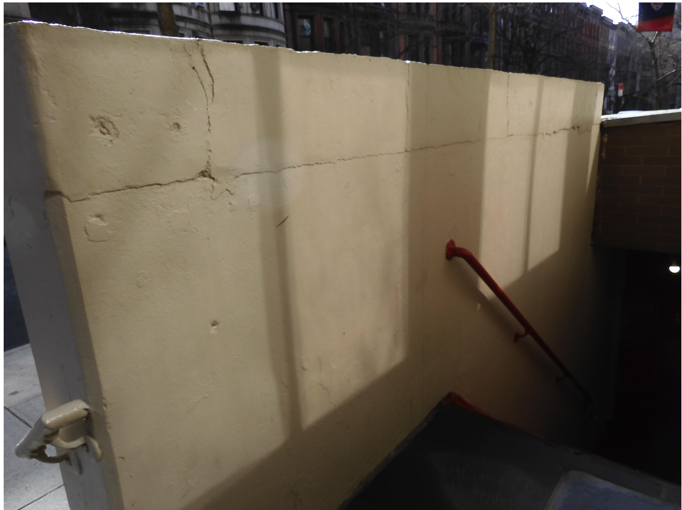
DETERIORATING CONCRETE WALL
