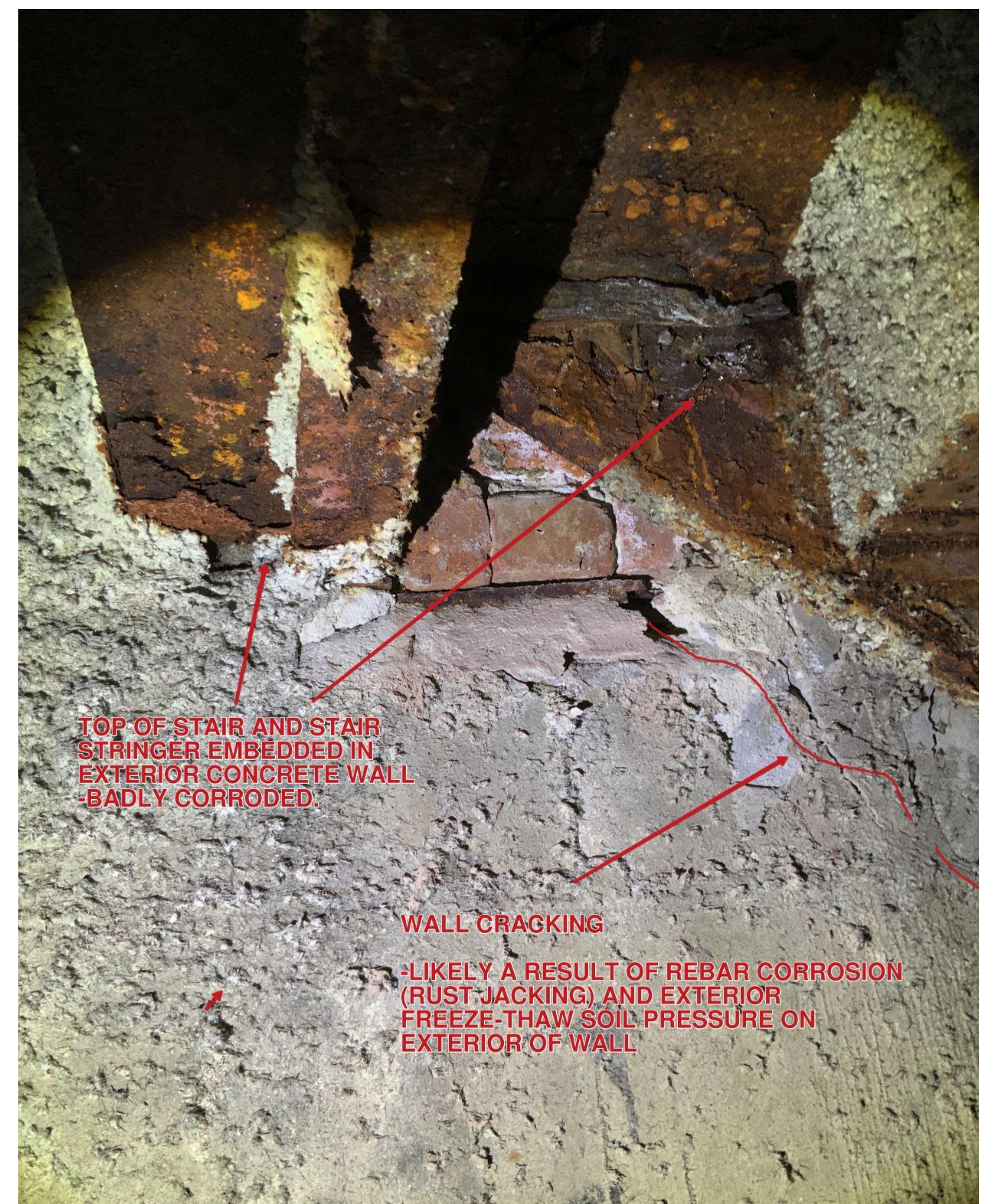
LANDING BEAM & STAIR CONDITION
