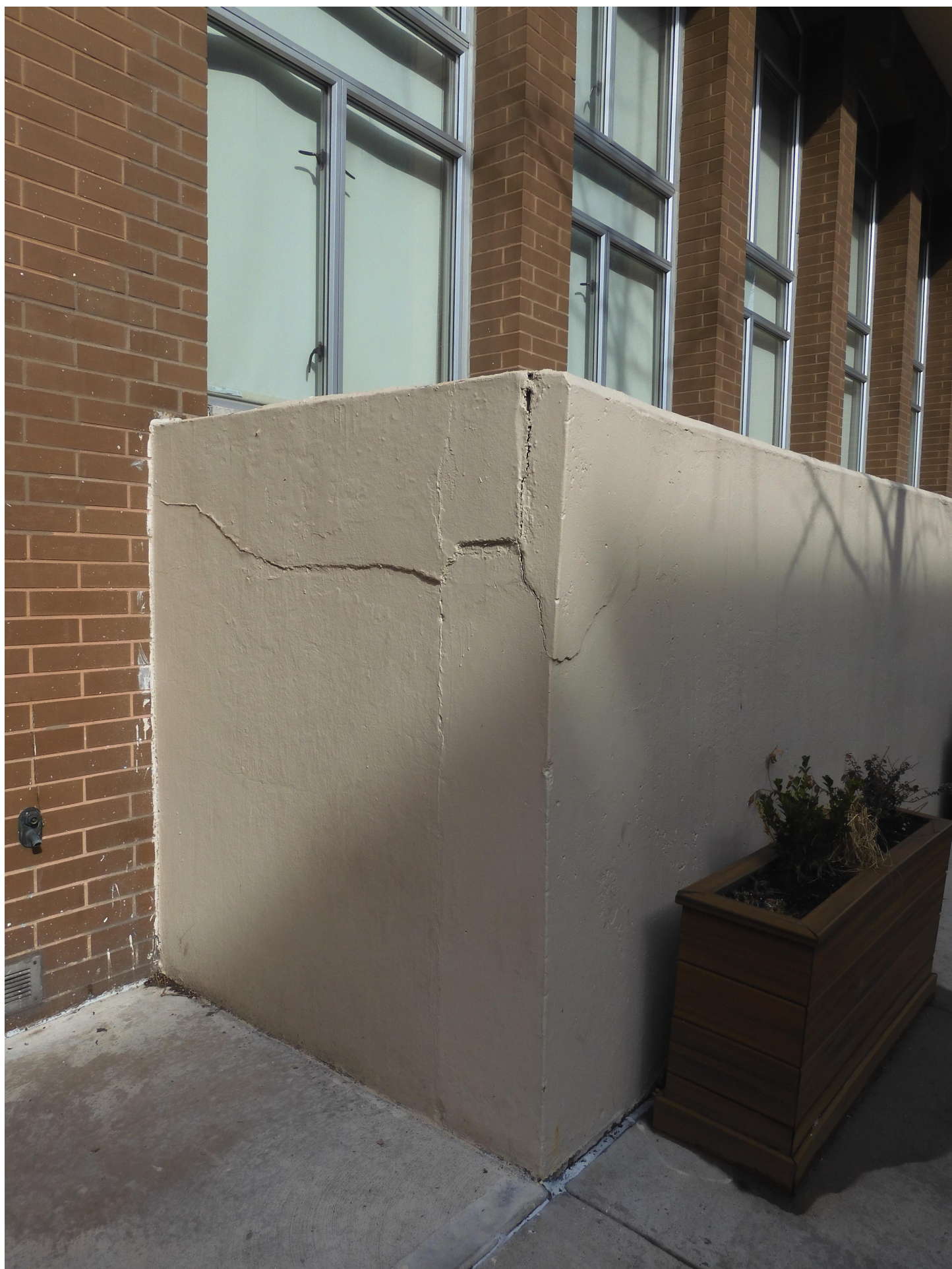
SPALLED CONCRETE WALL
