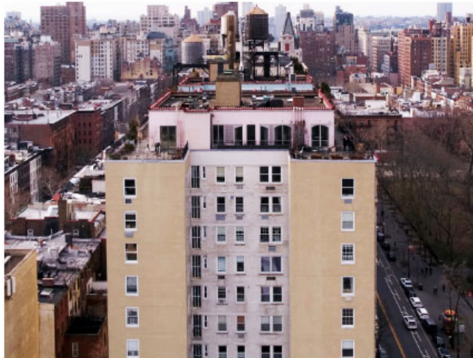
6th 77th street North Facade, Painted Brick
