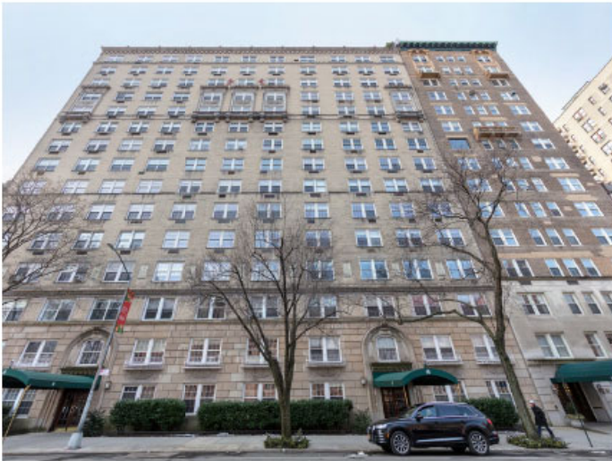
6th 77th street North Facade, Brick
