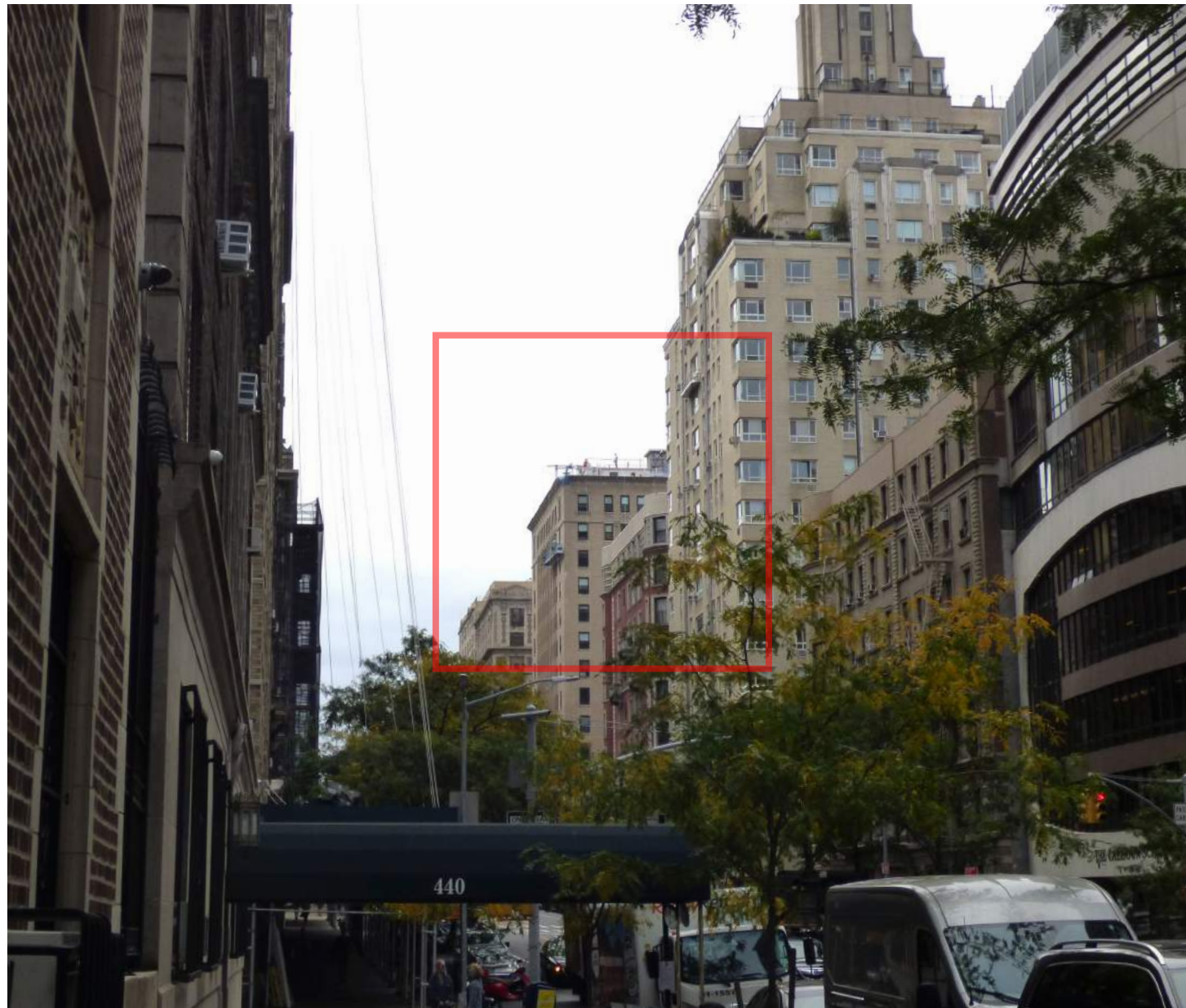
VIEW FROM 81ST ST (EXISTING)
