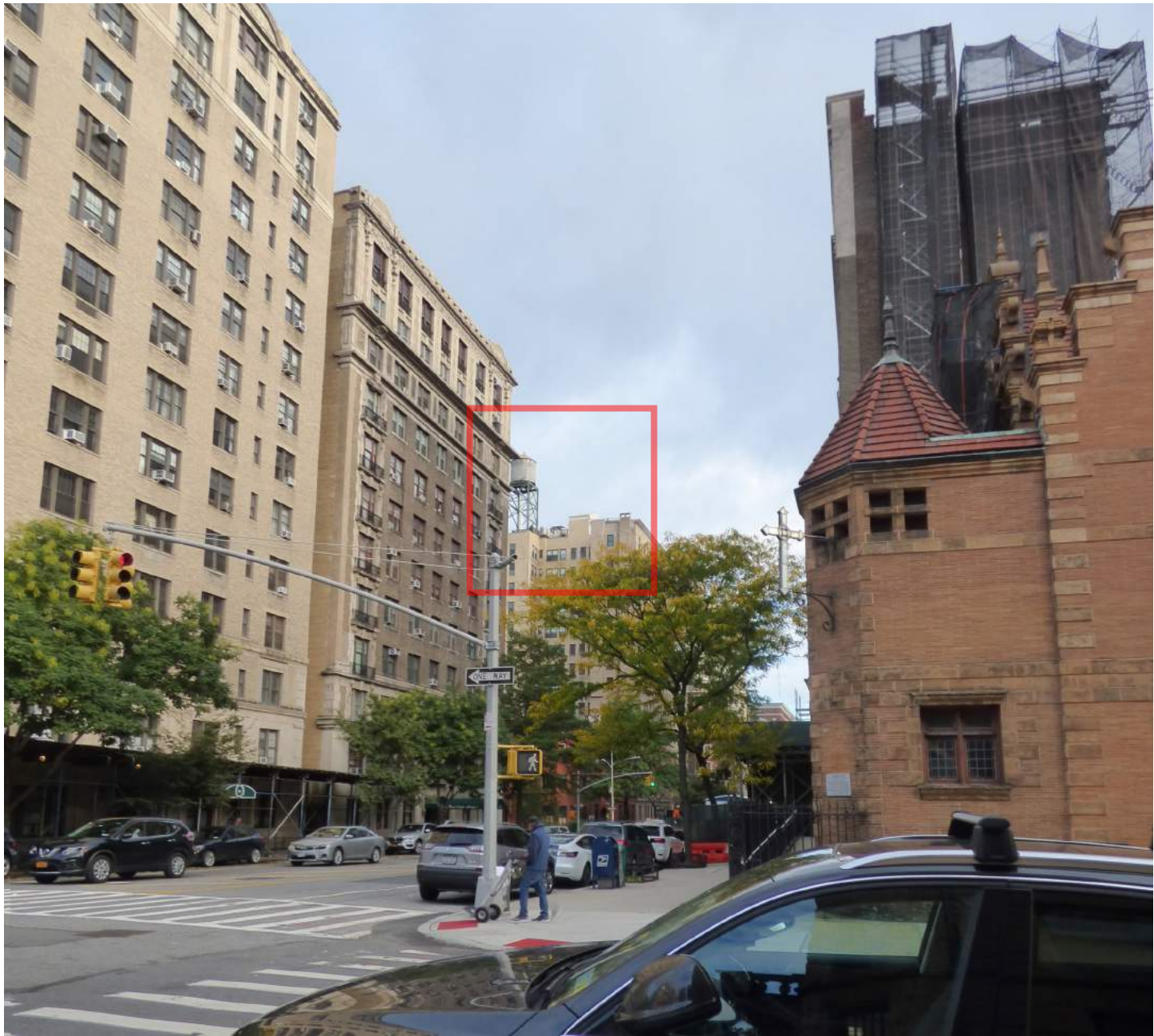
VIEW FROM 77TH ST (EXISTING)
