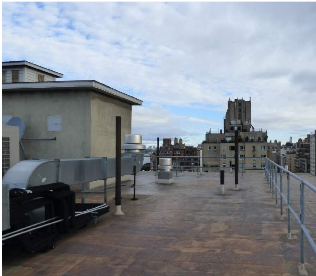
(G) EXISTING ELEVATOR BULKHEAD EAST FACADE
