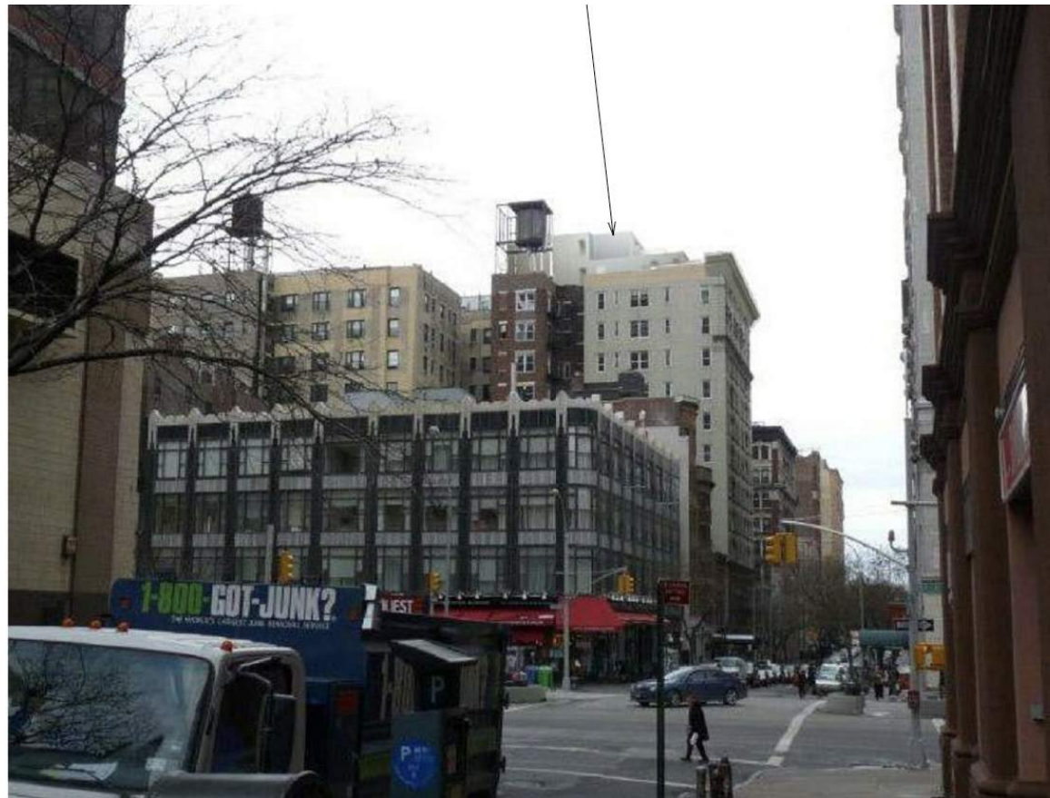
498 WEST END AVENUE (Riverside-West End Avenue HD Extension)
