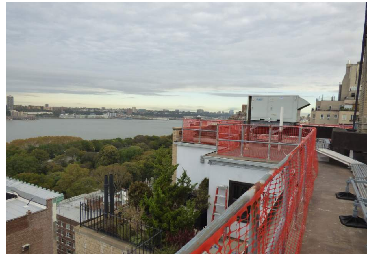
VIEW ALONG THE WEST ELEVATION OF THE MOCKUP, LOOKING NORTH.
