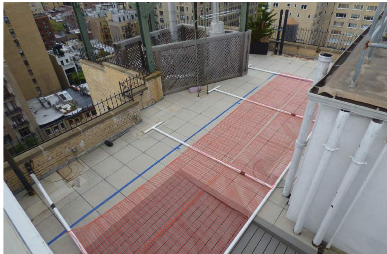
VIEW OF THE PENTHOUSE EXTENSION MOCKUP AT THE SOUTH ELEVATION OF THE BUILDING; THE PVC PIPING AND NETTING STOOD UPRIGHT AND WAS HELD IN PLACE AT THE BLUE LINE, MARKING THE SOUTHERNMOST EDGE OF THE EXTENSION.
