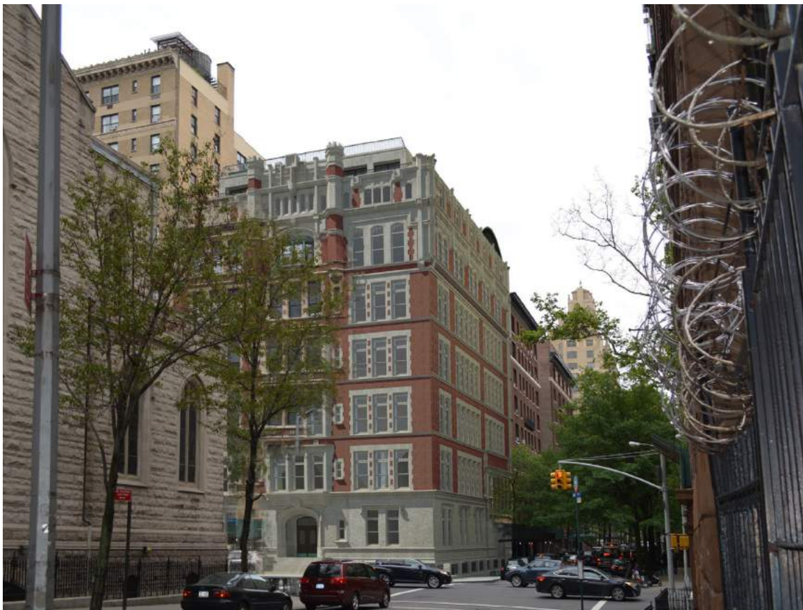
555 WEST END AVENUE (Riverside-West End Avenue HD Extension)
