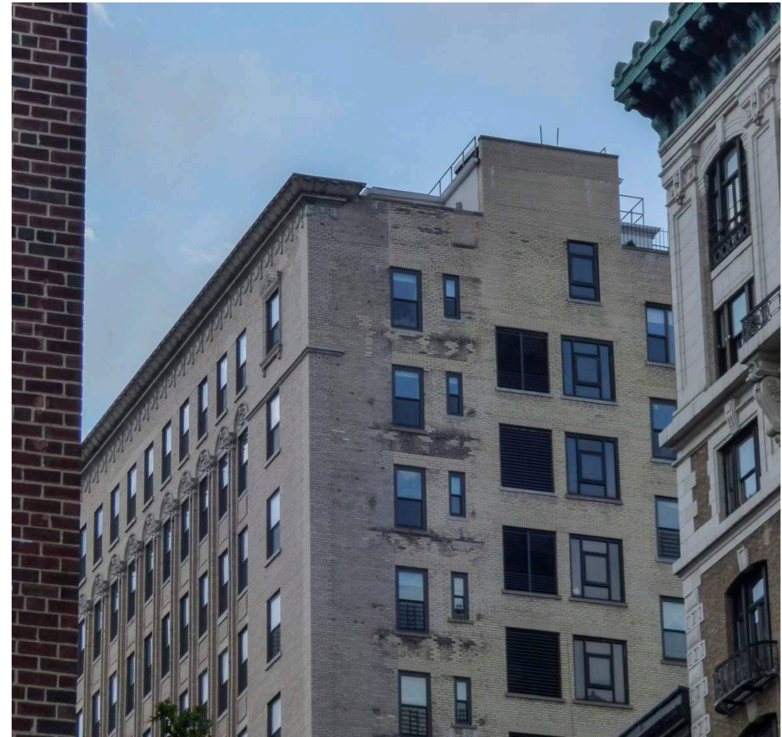
DETAIL VIEW OF THE WEST FACADE
