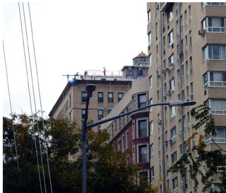
VIEW FROM 81ST ST (EXISTING)
