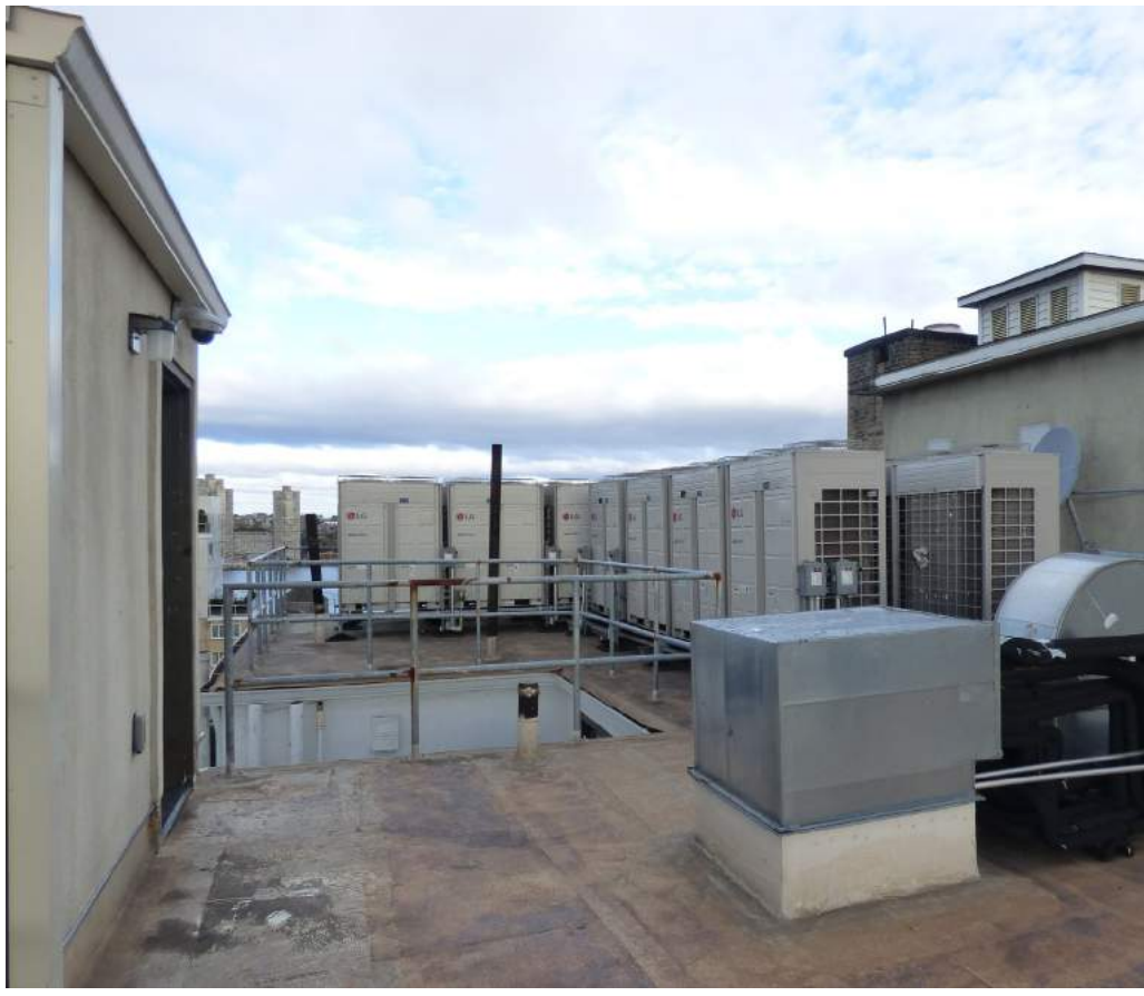
(H) EXISTING ELEVATOR BULKHEAD SOUTH FACADE
