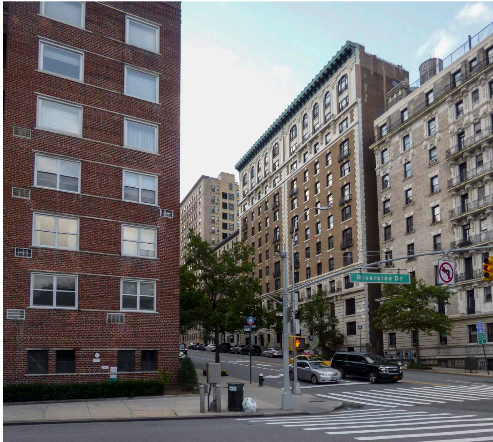
VIEW LOOKING EAST FROM RIVERSIDE PARK
