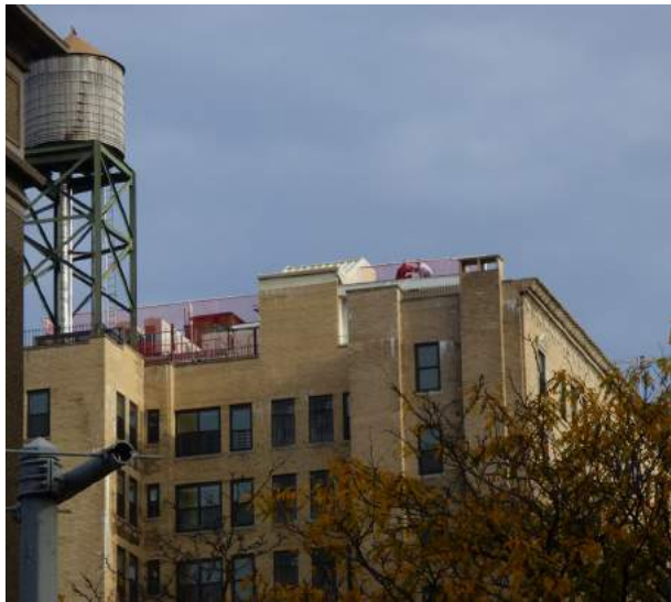
VIEW FROM 77TH ST (EXISTING)
