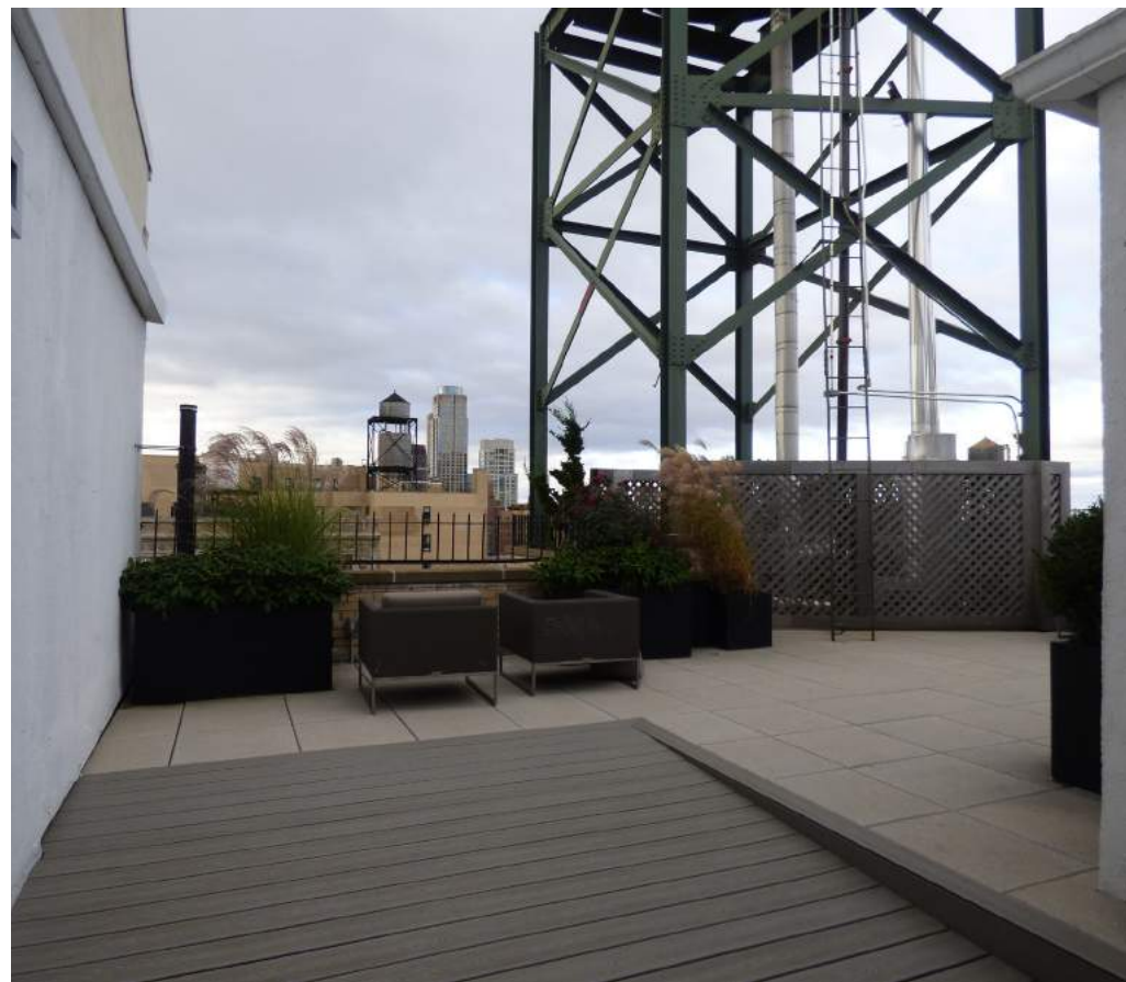
(A) EXISTING FACADE - SOUTH VIEW
