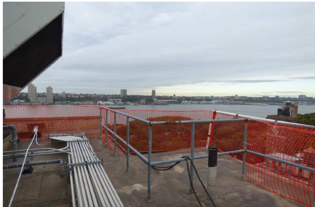
VIEW OF THE NORTHWEST CORNER OF THE MOCKUP,
