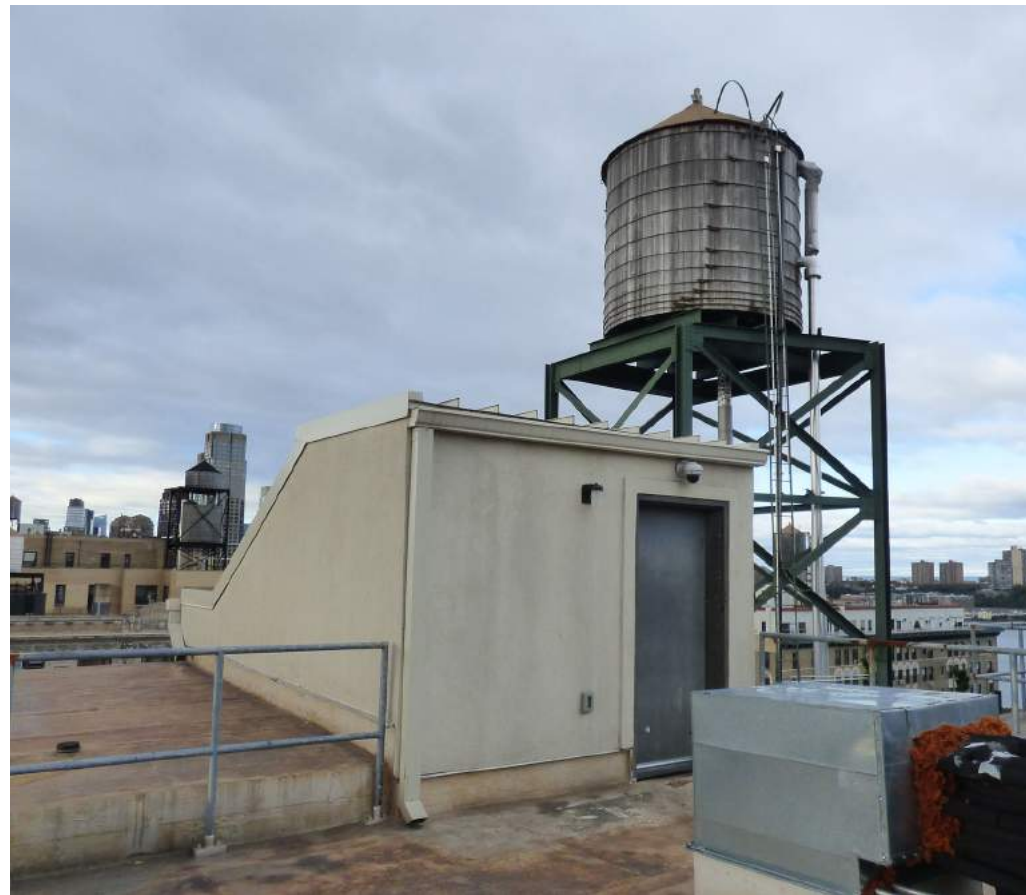
(F) EXISTING STAIR BULKHEAD FACADE
