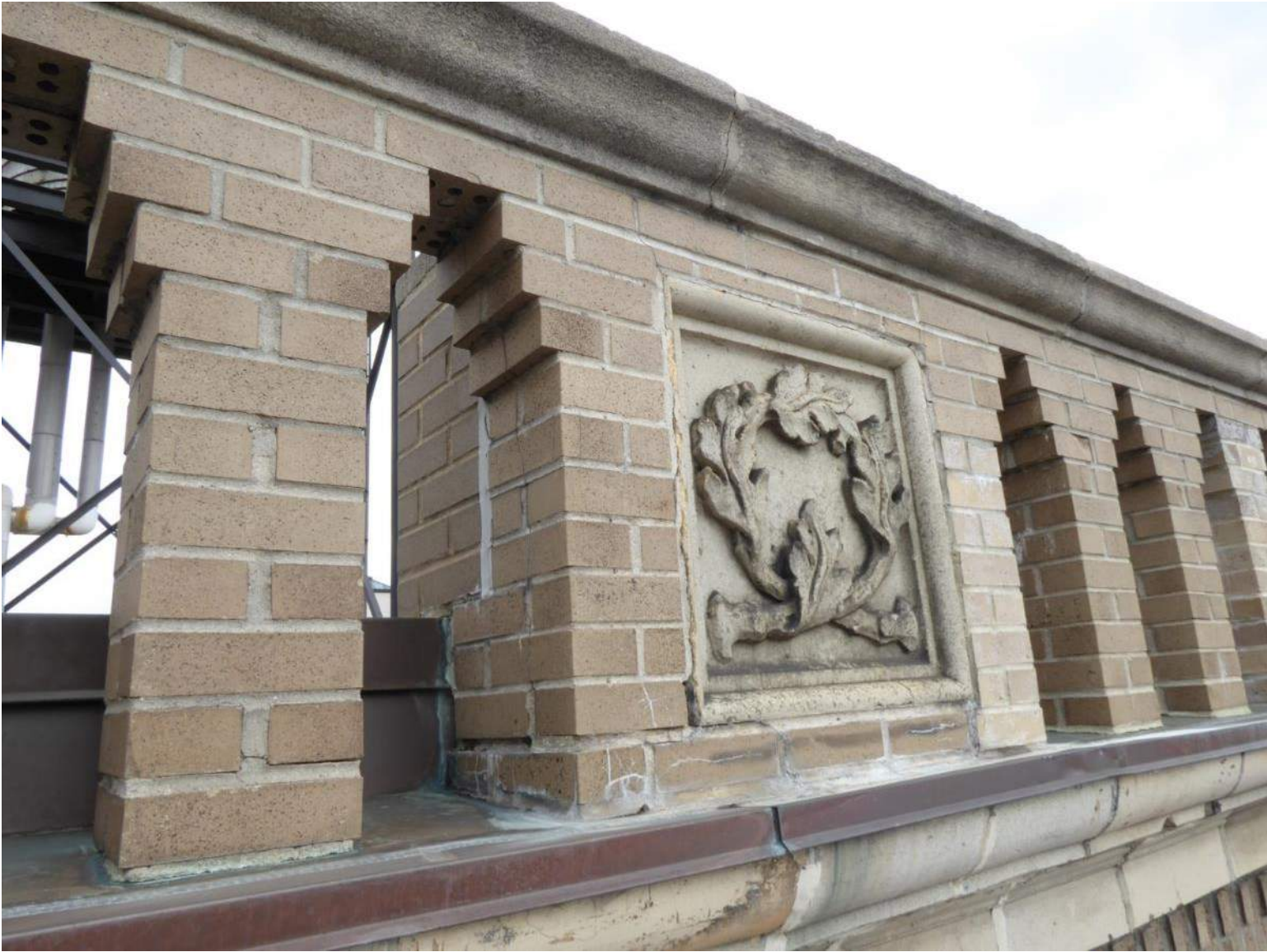
Balustrade pier deterioration (location along 89 th Street side)
