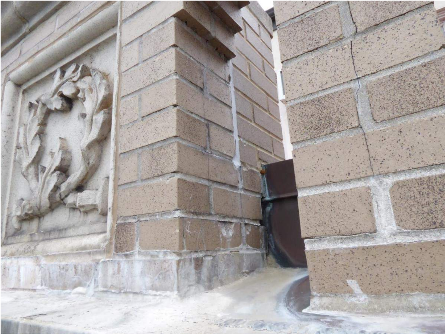
Balustrade pier deterioration (location along Riverside Drive)
