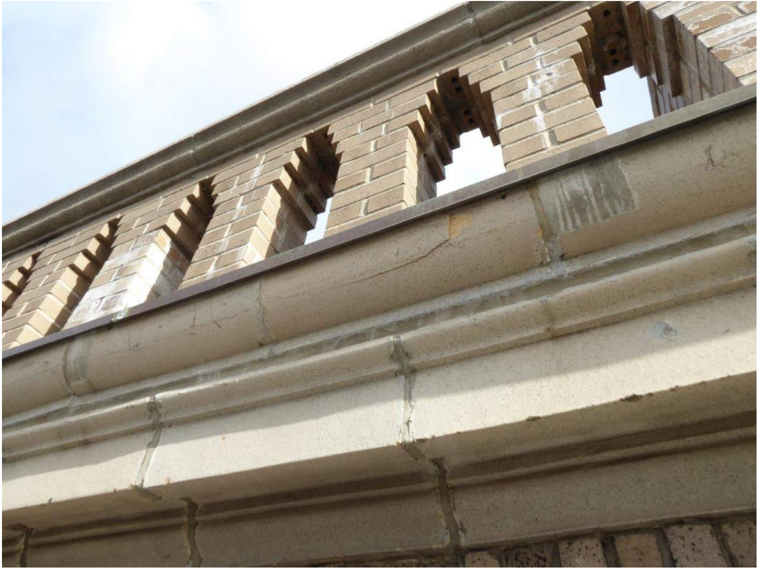
Balustrade and cornice deterioration (additional location along 89 th Street)
