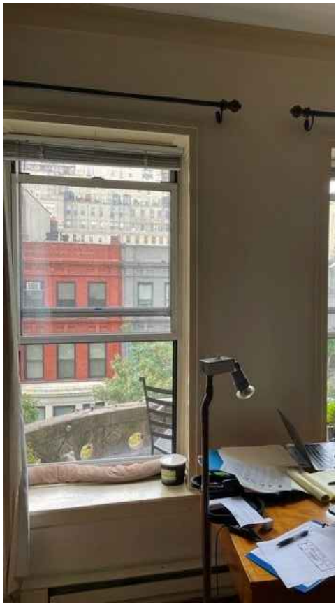
Existing Condition - Interior View
