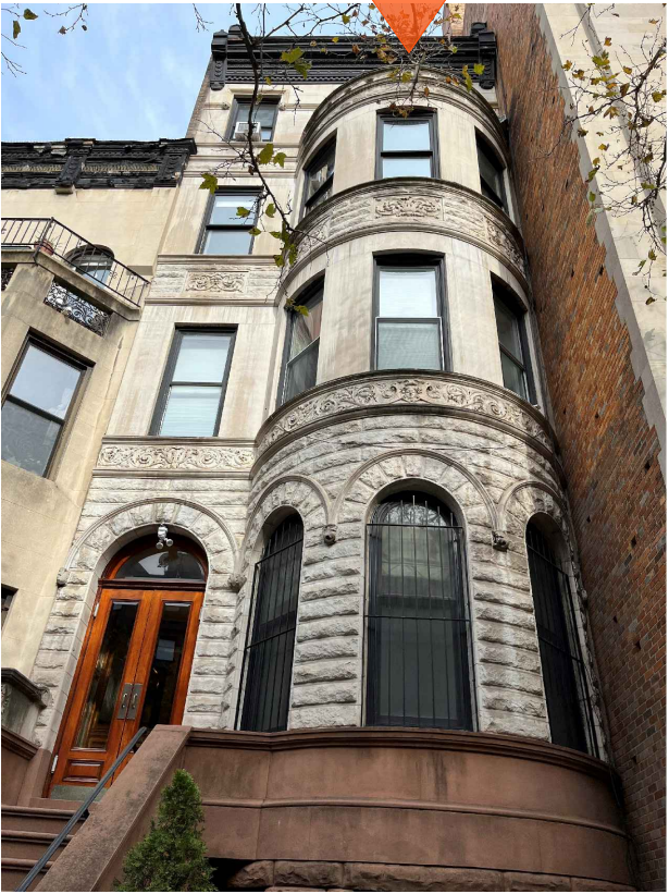
From sidewalk directly in front of building
