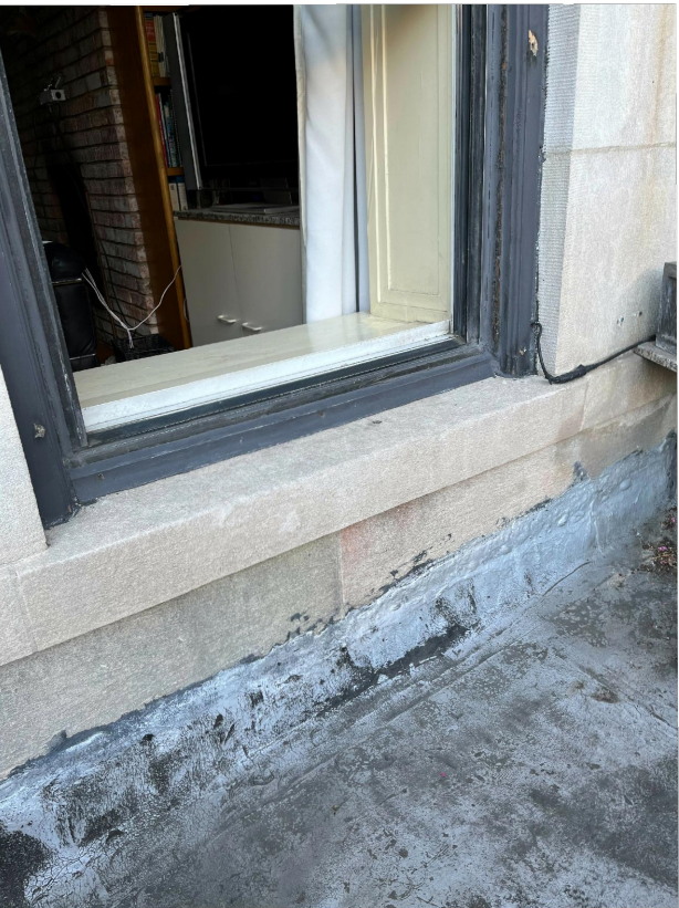
Existing exterior sill
