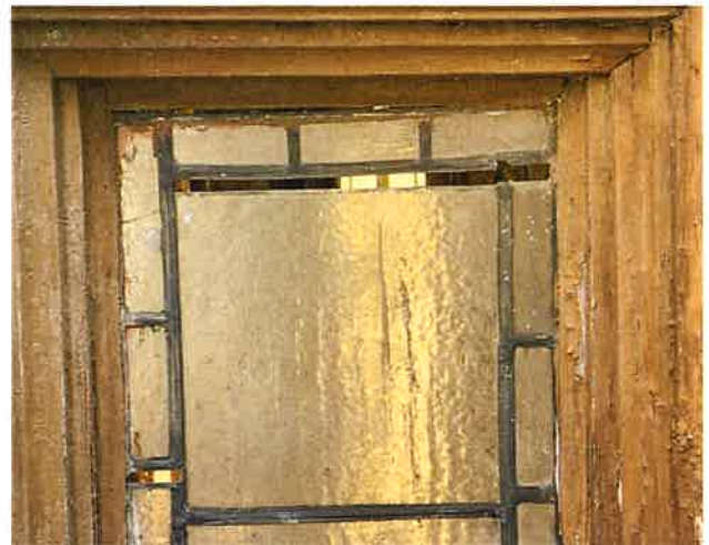
South Tower – Deteriorated Leaded Window
