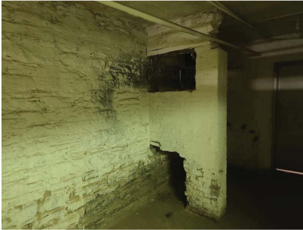
PHOTO 9: VOIDS IN BEARING WALL AT CELLAR
