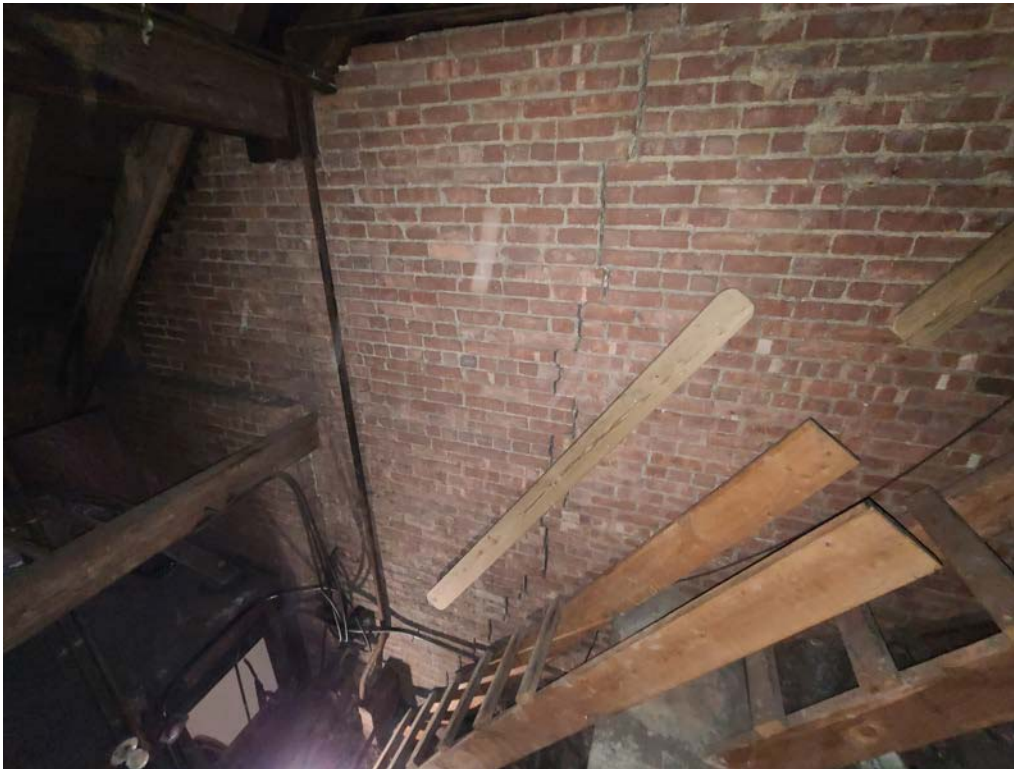
PHOTO 6: WIDE CRACK AT BRICK BEARING WALL EAST OF SANCTUARY
