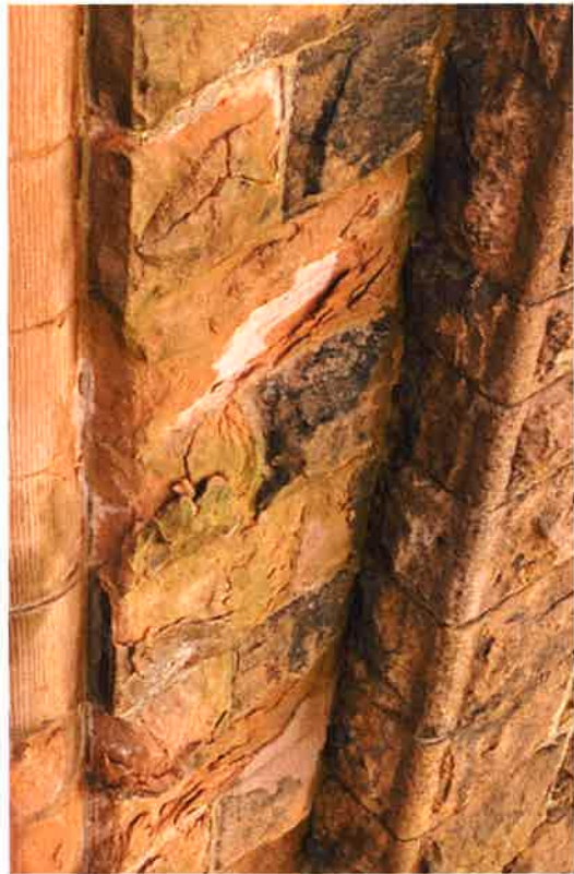
North Tower – Spalled Stones
