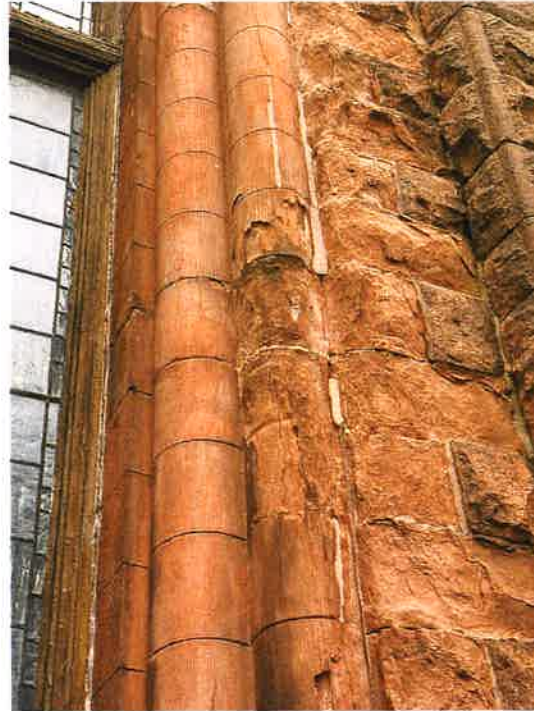
East Tower – Spalled Stones
