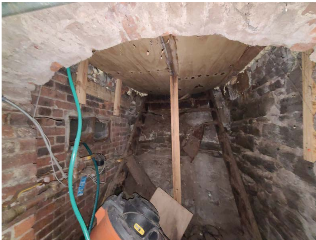
PHOTO 8: INADEQUATE SIDEWALK VAULT COVER SUPPORT
