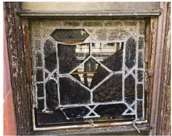
West Church – Spalled stone at window. West Church – Stained glass window compromised.
