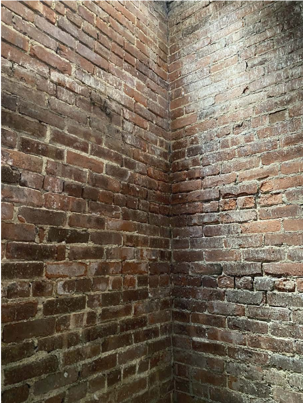
PHOTO 11: BELL TOWER BRICK REQUIRES POINTING
