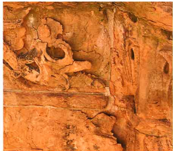
West Tower- Spalled and Deteriorated Stone
