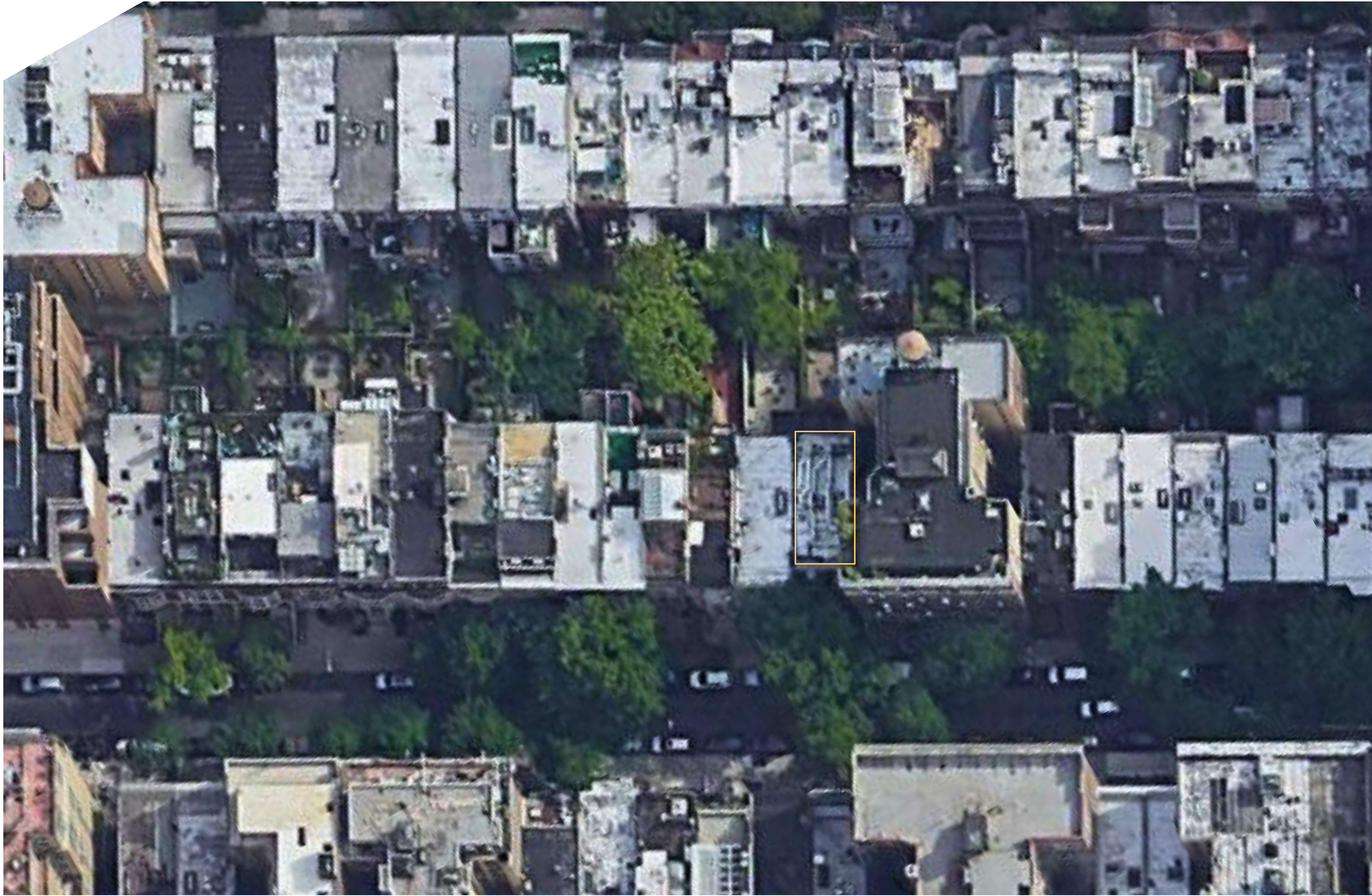
1 BLOCK AERIAL OF EXISTING ROOF TOPS
