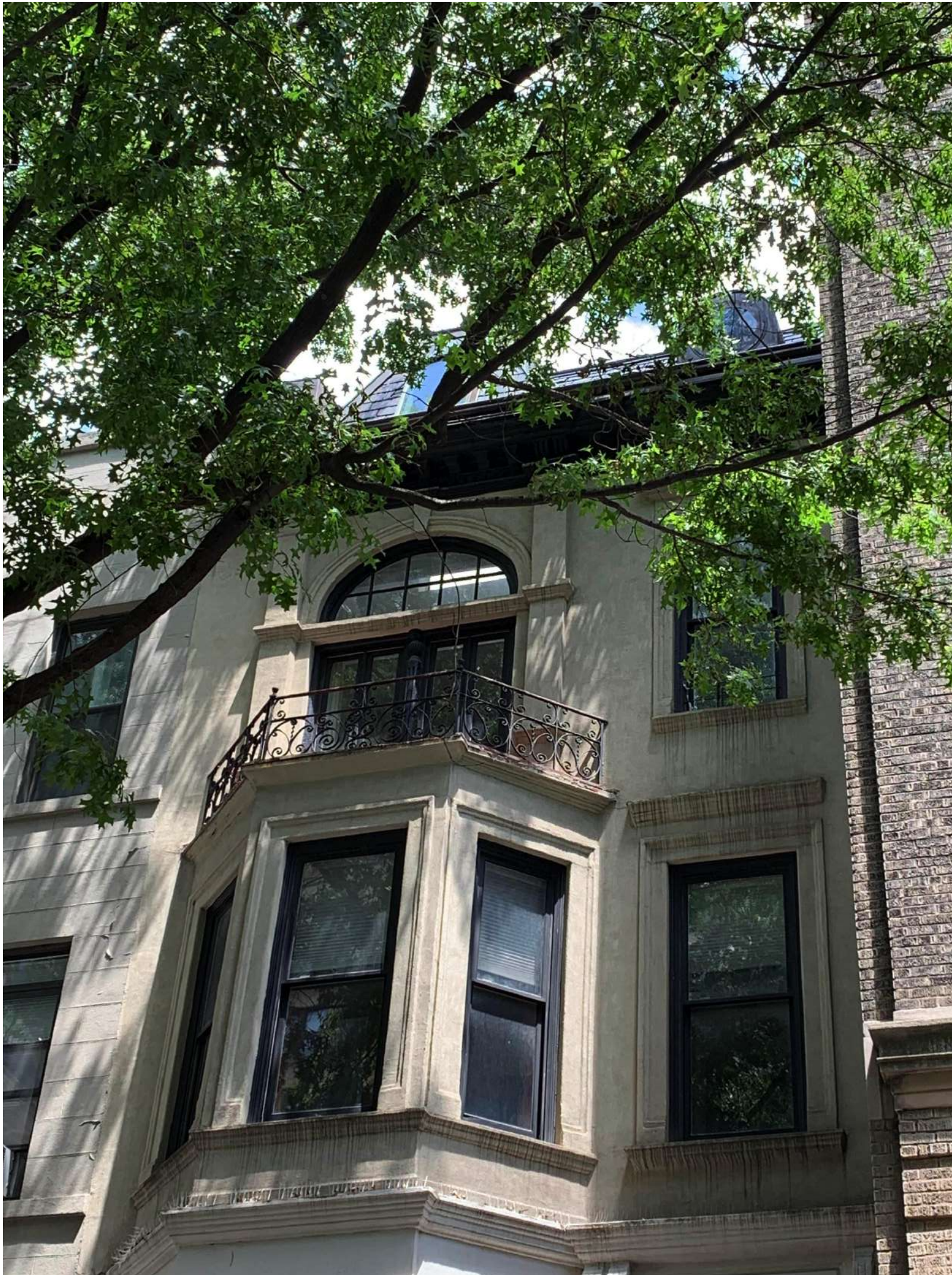
THIRD FLOOR DOOR AND TRANSOM
