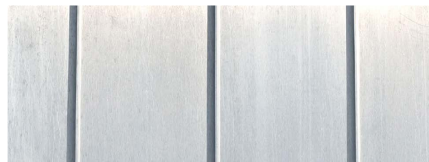
Pre-weathered zink "Mansard Roof" to match existing gutter
