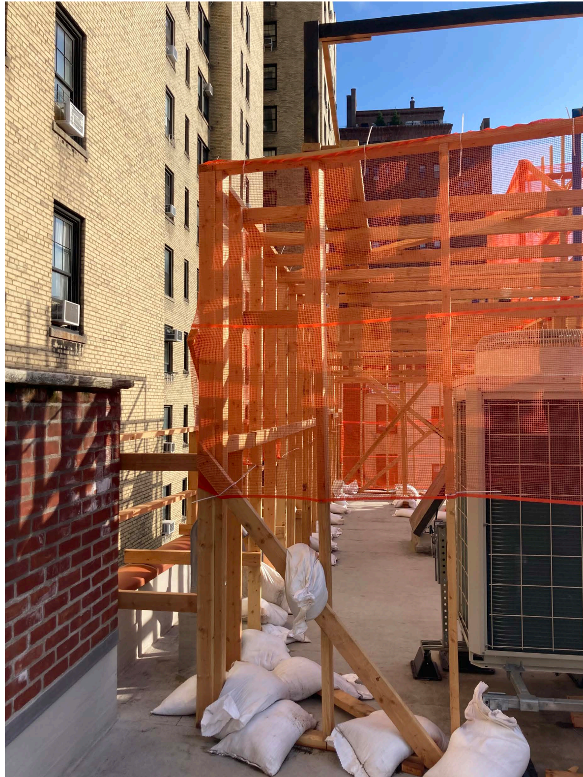
North-East Corner: Showing proposed additional story, guardrail, & raised parapet heights
