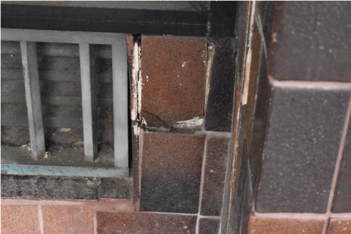
Cracked Tiles Delaminating From Substrate
