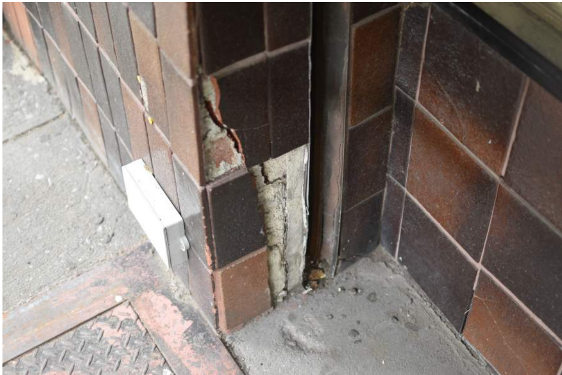
Cracked and Delaminated Tiles
