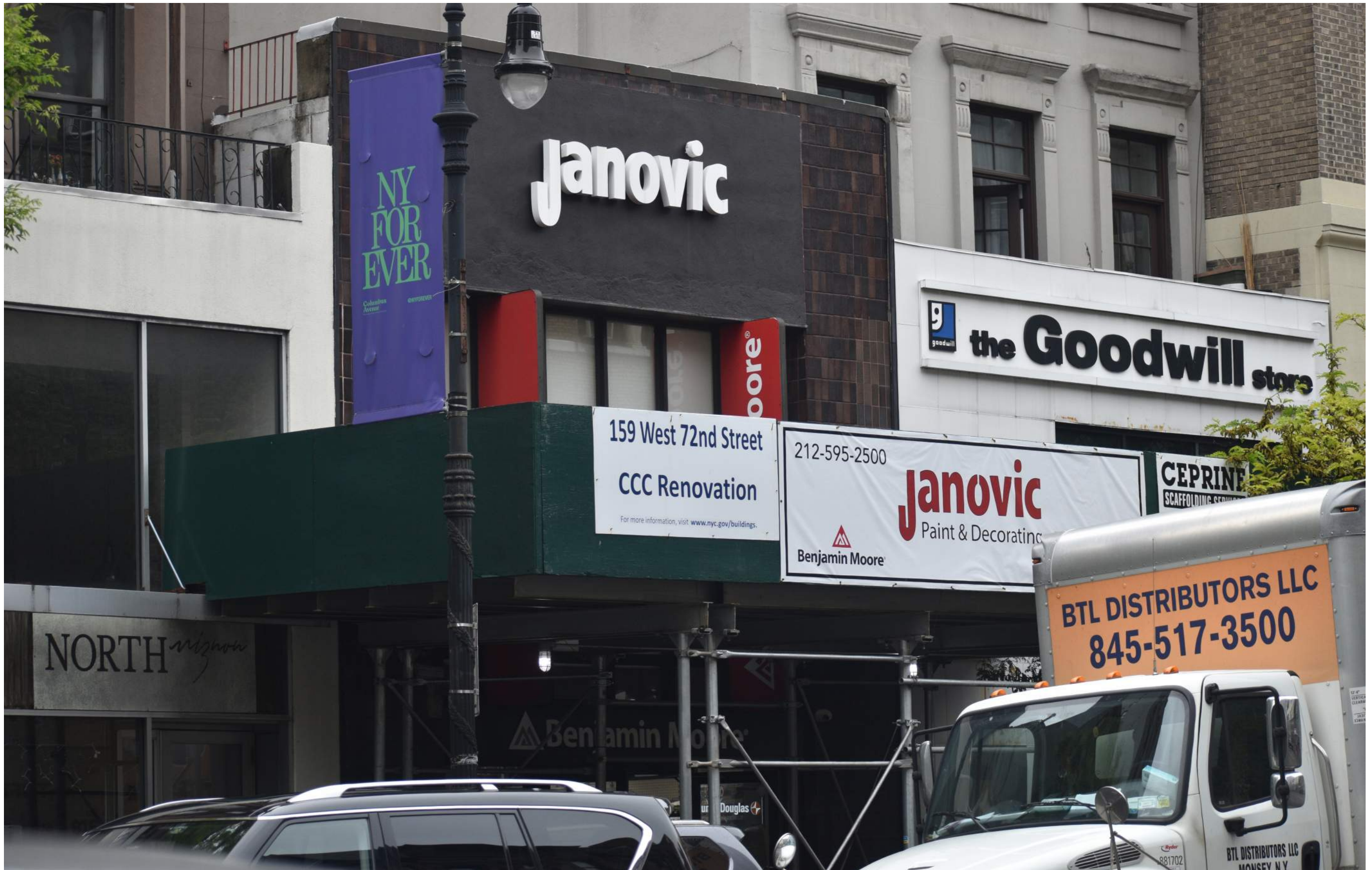
Erected Sidewalk Shed For Public Safety
