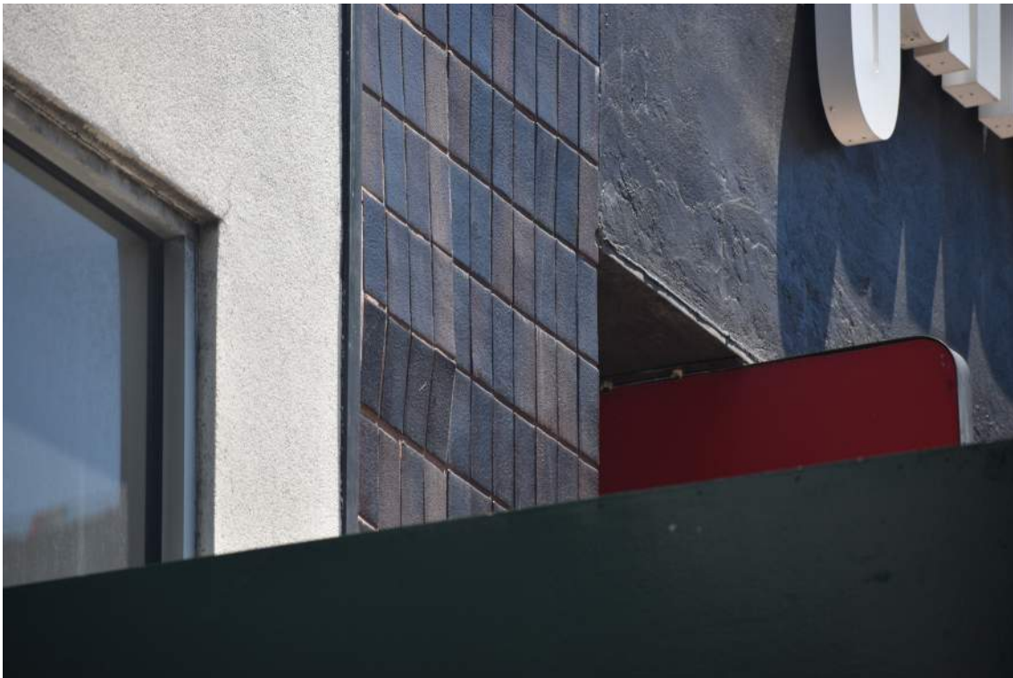
Bulging Tiles Delaminating From Substrate
