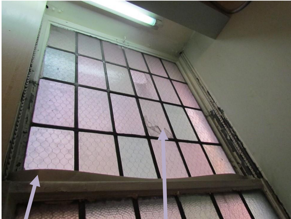
TEMPORARY INSULATION, GAPS PRESENT
