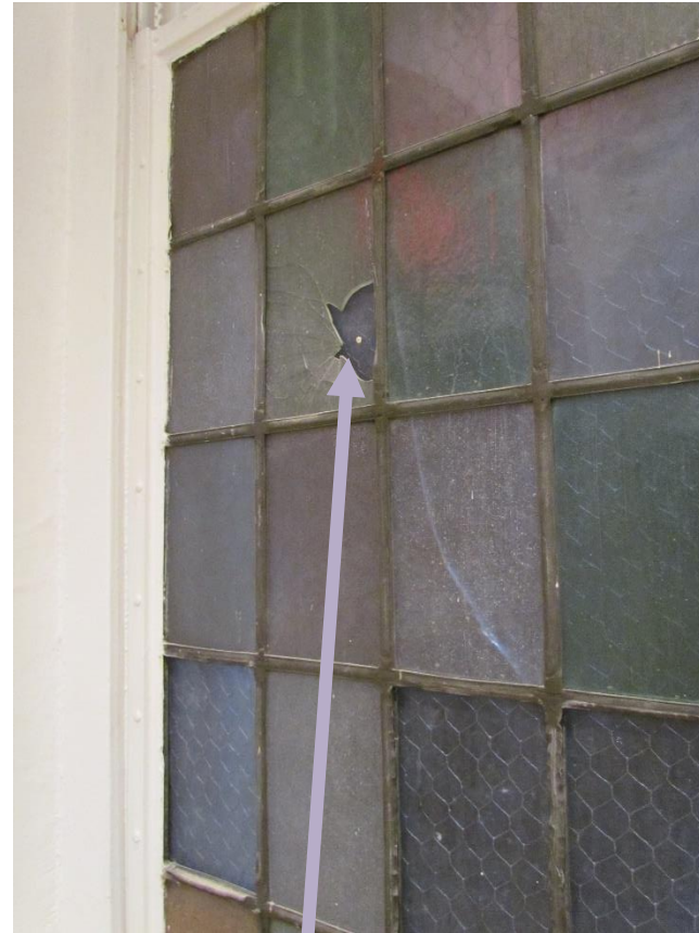
CRACKED GLAZING
