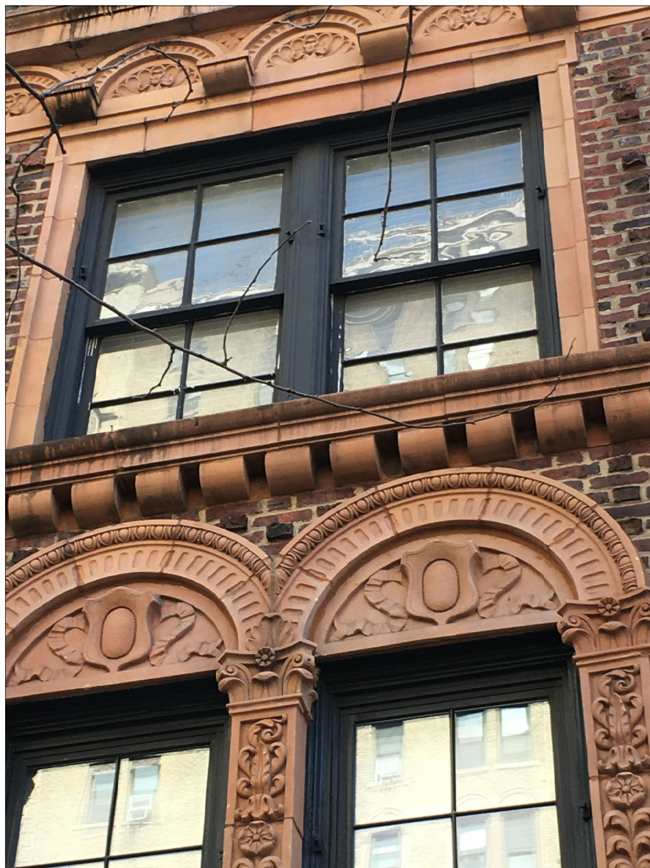
2 EXISTING DOUBLE HUNG WINDOW, TYP @ BUILDING SCALE: NONE
