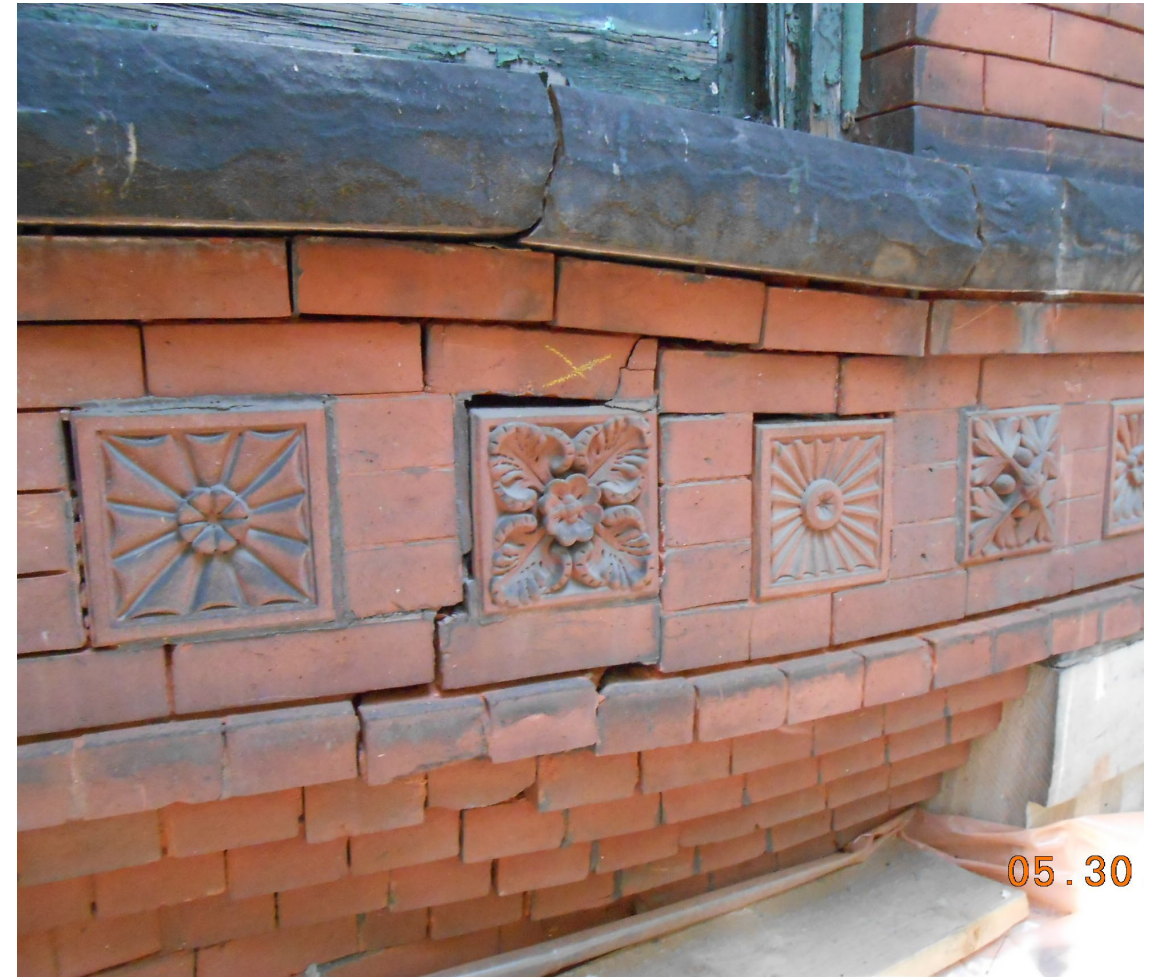
233 West 75 th Street (Projecting bow window. masonry severely displaced vertically and horizontally from settlement of the facades) Photos taken 2012
