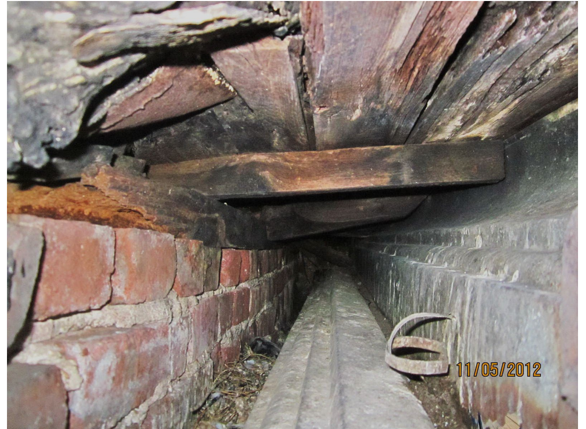
233 West 75 th Street (Severe deterioration at Mansard Roof and underlying brick masonry)
