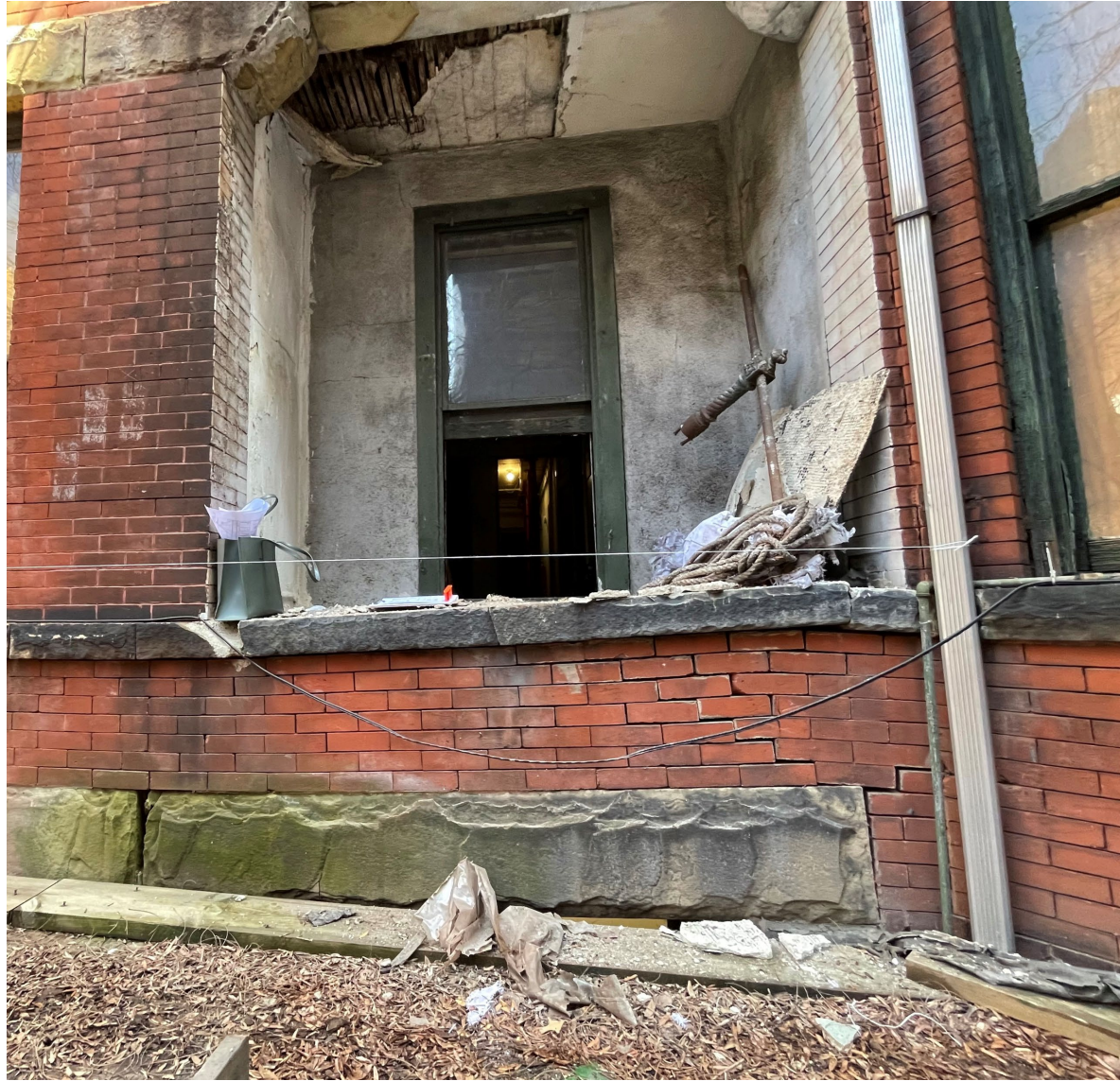
231 West 74 th Street (Lintel above main Entrance severely deformed from façade settlement) 2022
