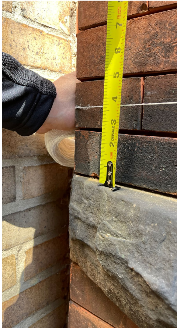
String Level indicates that portion of building adjacent to party wall between (2) buildings has settled close to 3 inches relative to West end of 233 and East end of 231.) Photos taken 2022
