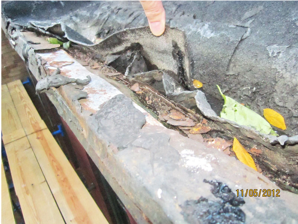
233 West 75 th Street (Severe deterioration at Mansard Roof and underlying brick masonry)
