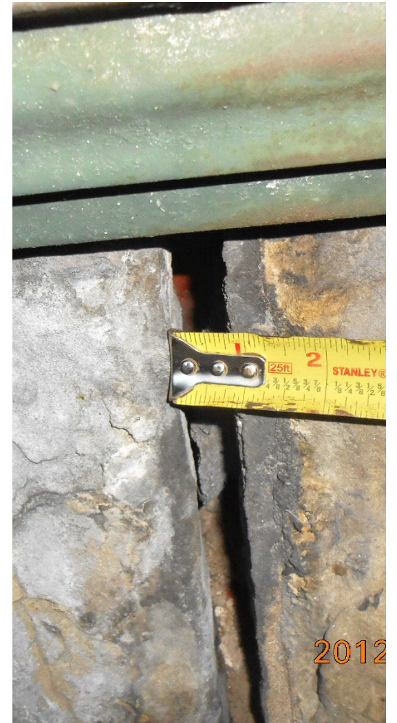
231 / 233 West 75 th Street (Differential Façade Settlement visible at misaligned gutters and mortar joint widths ) Photos Taken 2012
