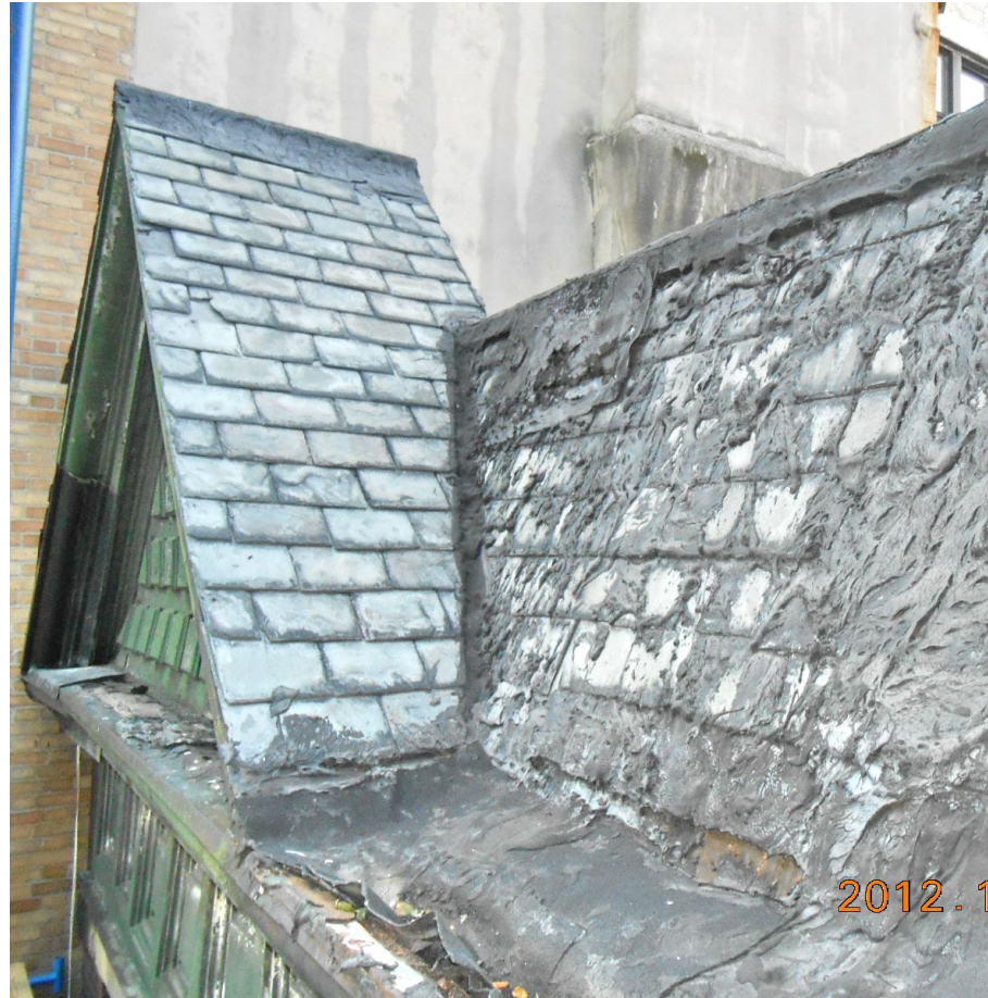
233 West 75 th Street (Severe deterioration of Mansard and Gable Roofs and Integral gutter) Photos taken 2012
