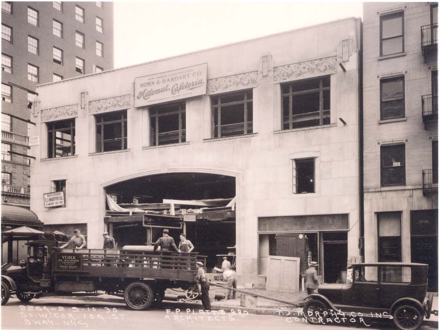
Horn & Hardart Automat-Cafeteria Building, under construction (1930)
