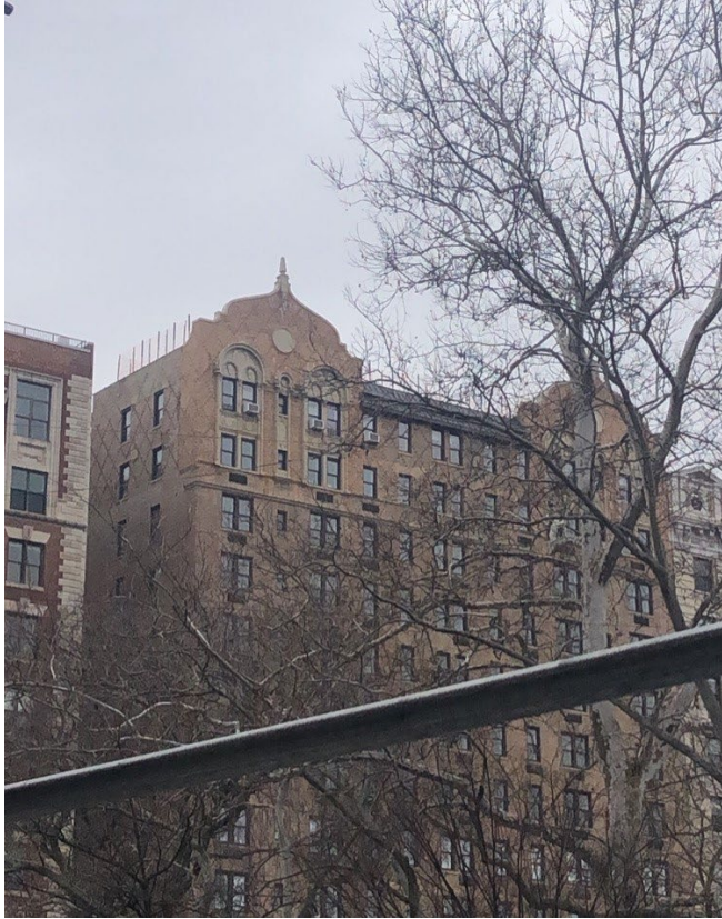
View from Columbus Avenue showing visibility impacts on the decorative arch.
