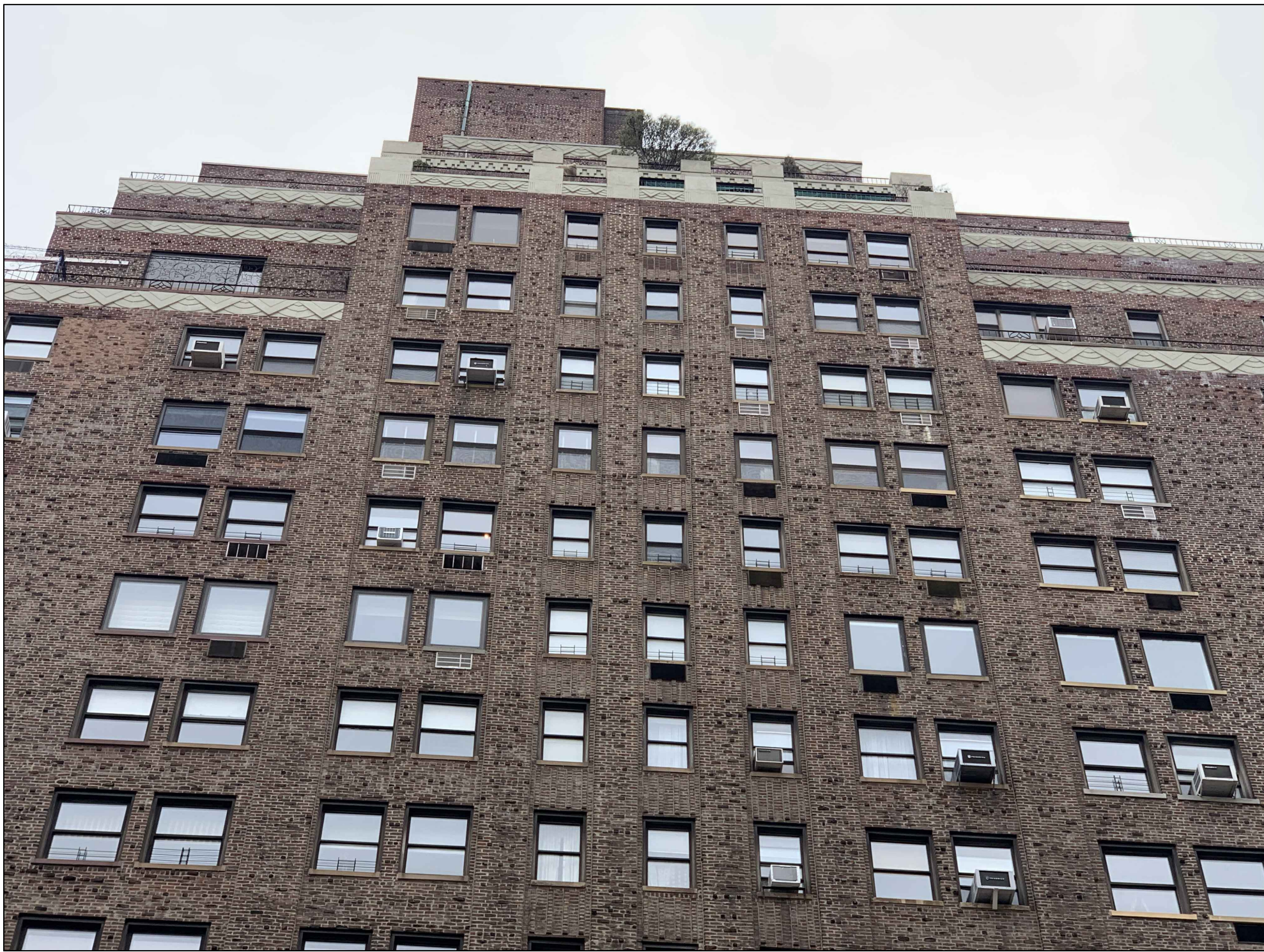
Close-up View from West 79th Street Majority of windows are one-over-one aluminum double hungs with bronze exteriors
