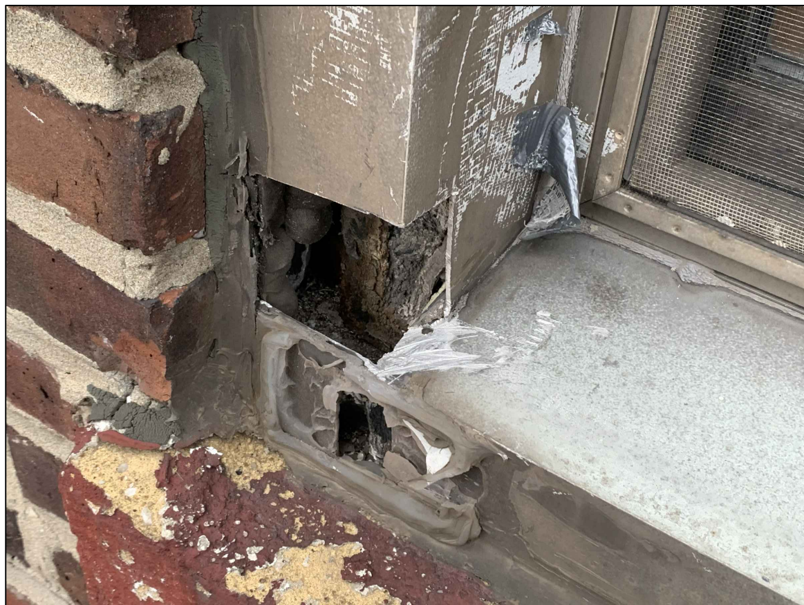
Probe completed to show that no historic brickmold casing exists under aluminum panning.
