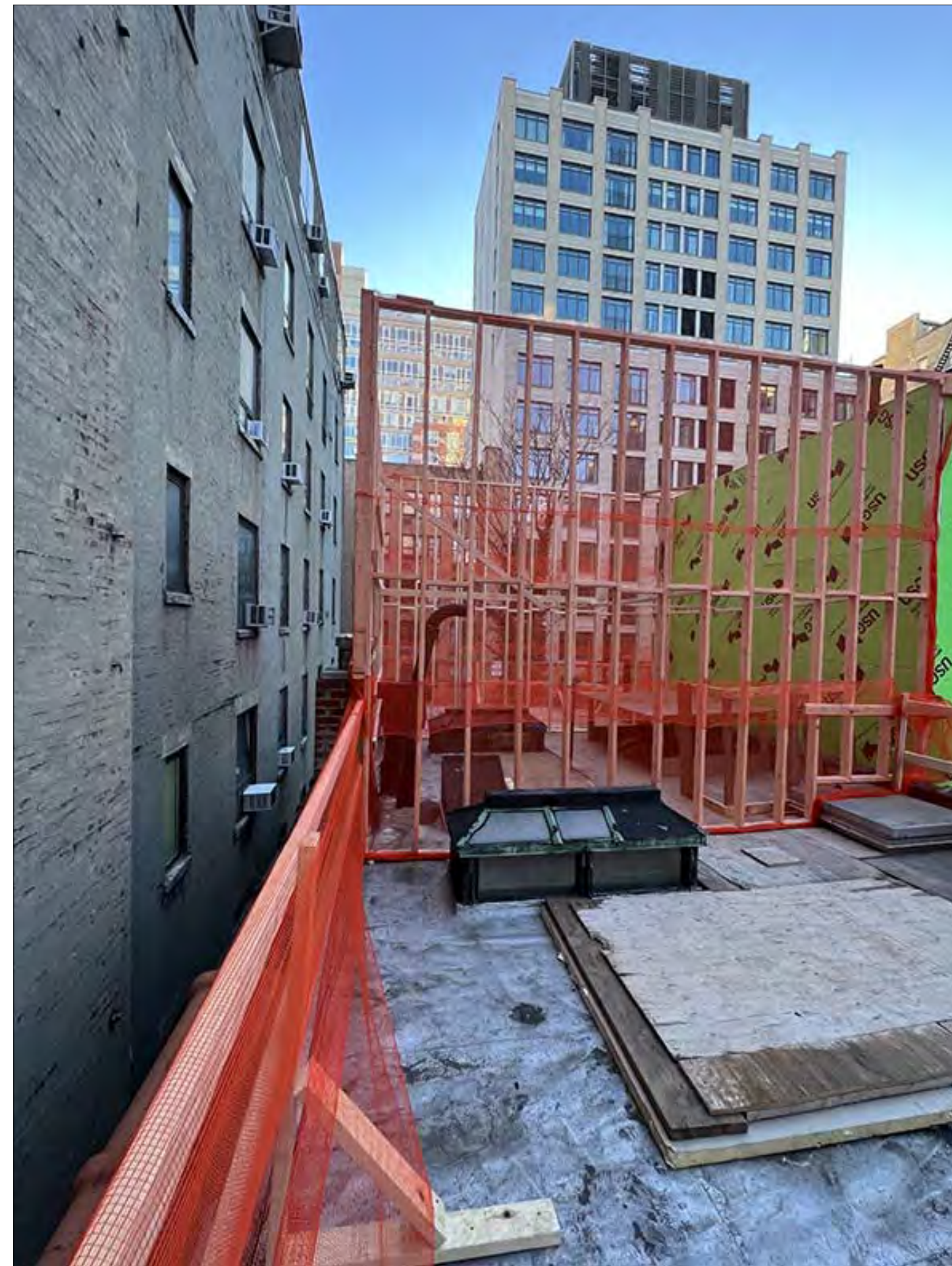
ROOF- LOOKING SOUTH WEST
