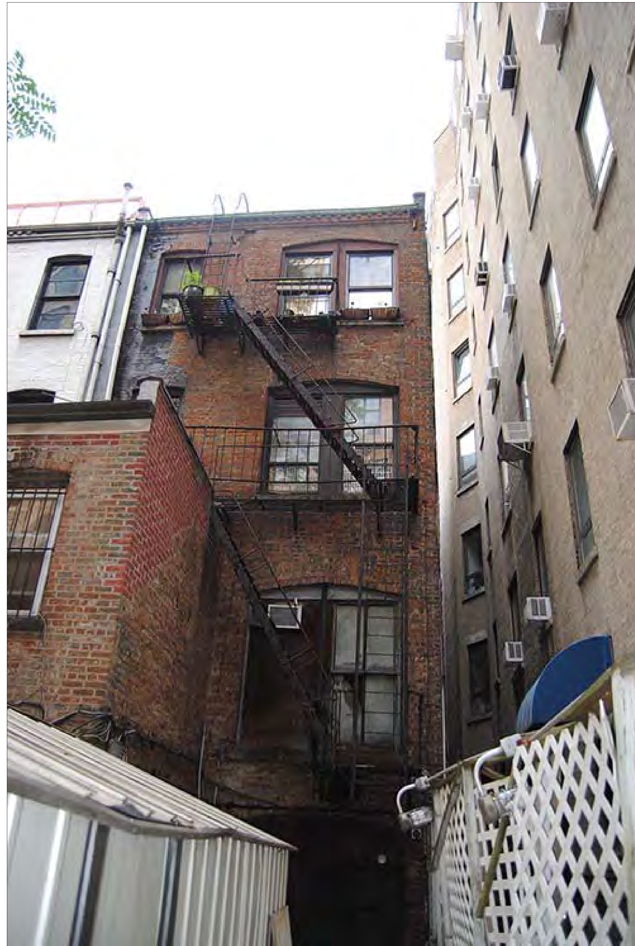
EXISTING SOUTH FACADE
