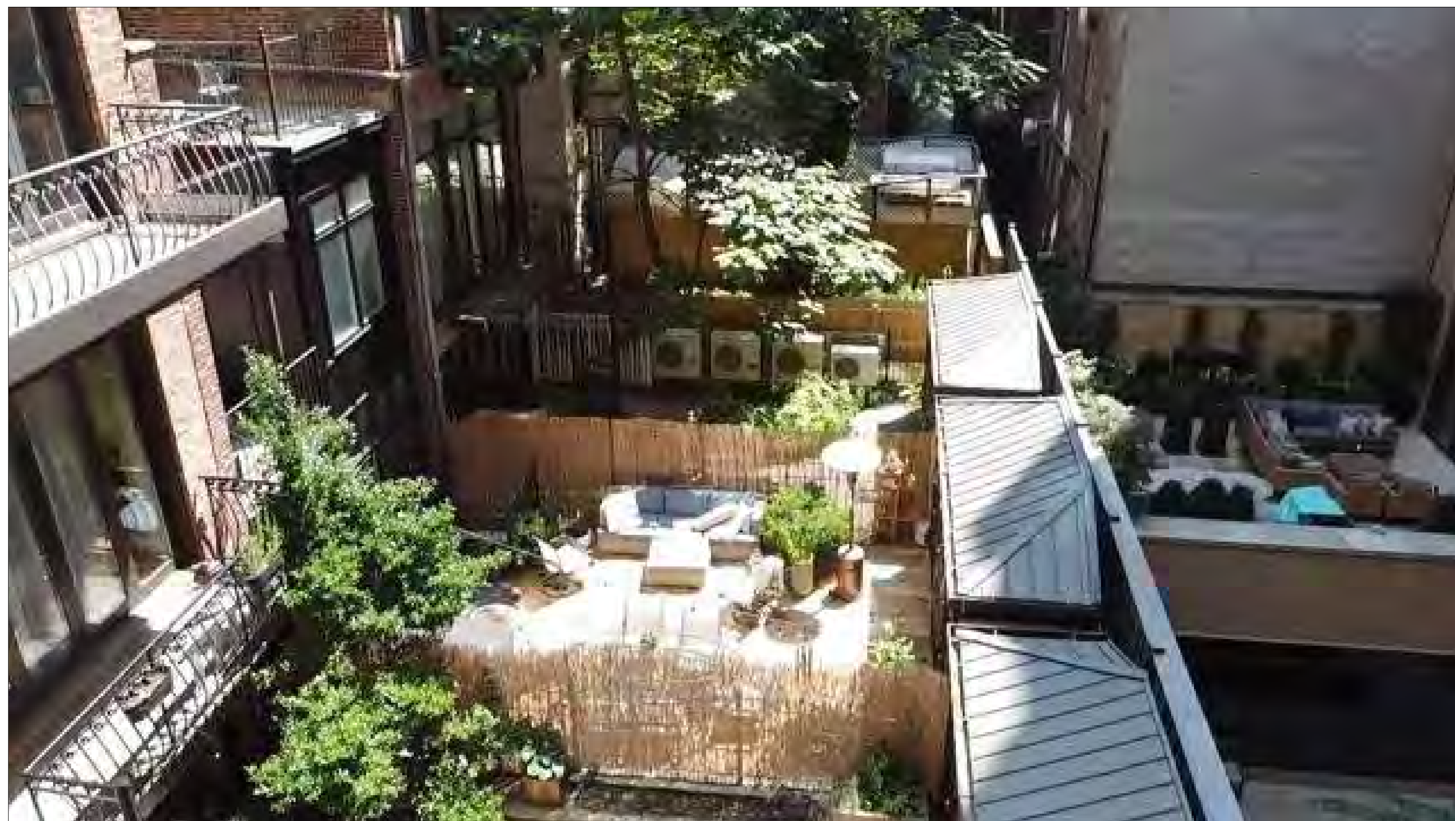
INTERIOR BLOCK LOOKING EAST
