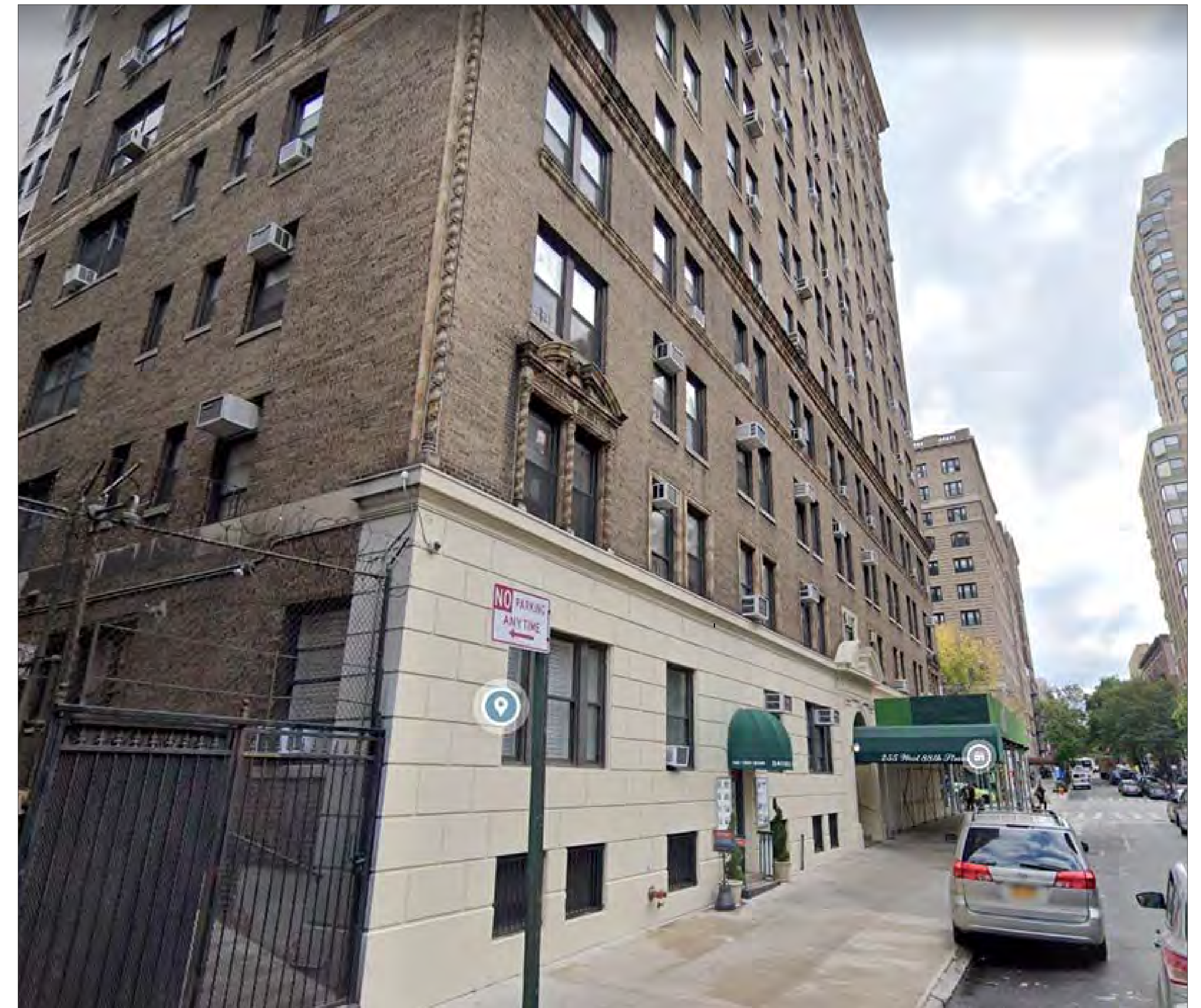
NORTH SIDE OF WEST 88TH STREET, LOOKING EAST
