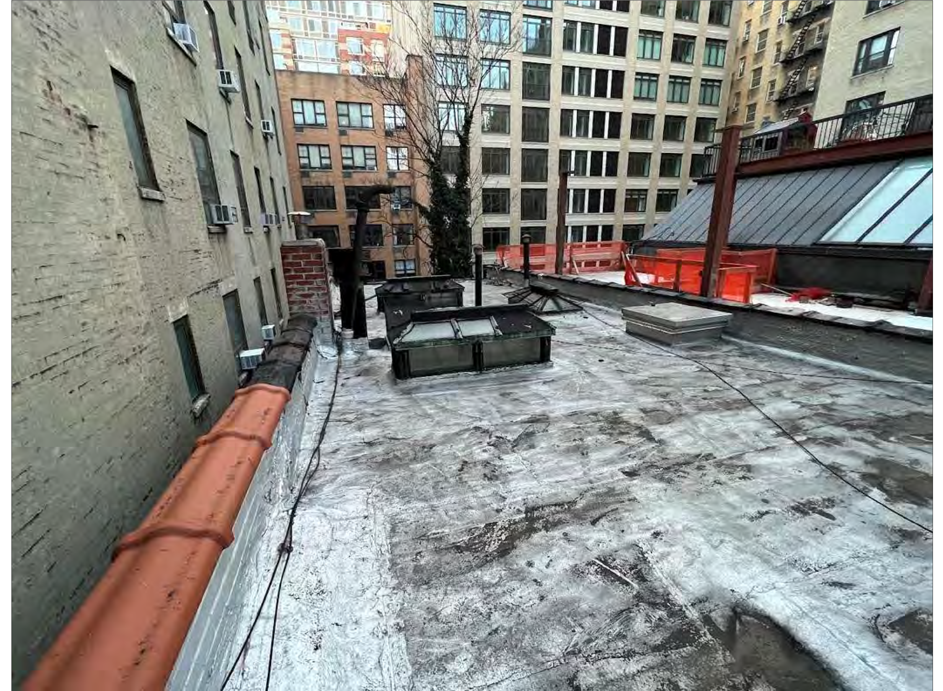
EXISTING ROOF, LOOKING SOUTH
