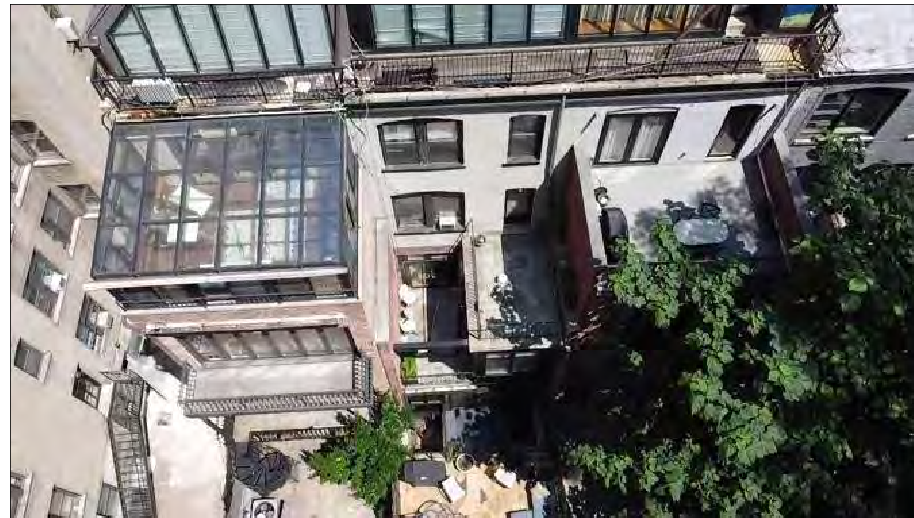
EXISTING REAR ADDITIONS AT ROWHOUSES TO THE WEST
