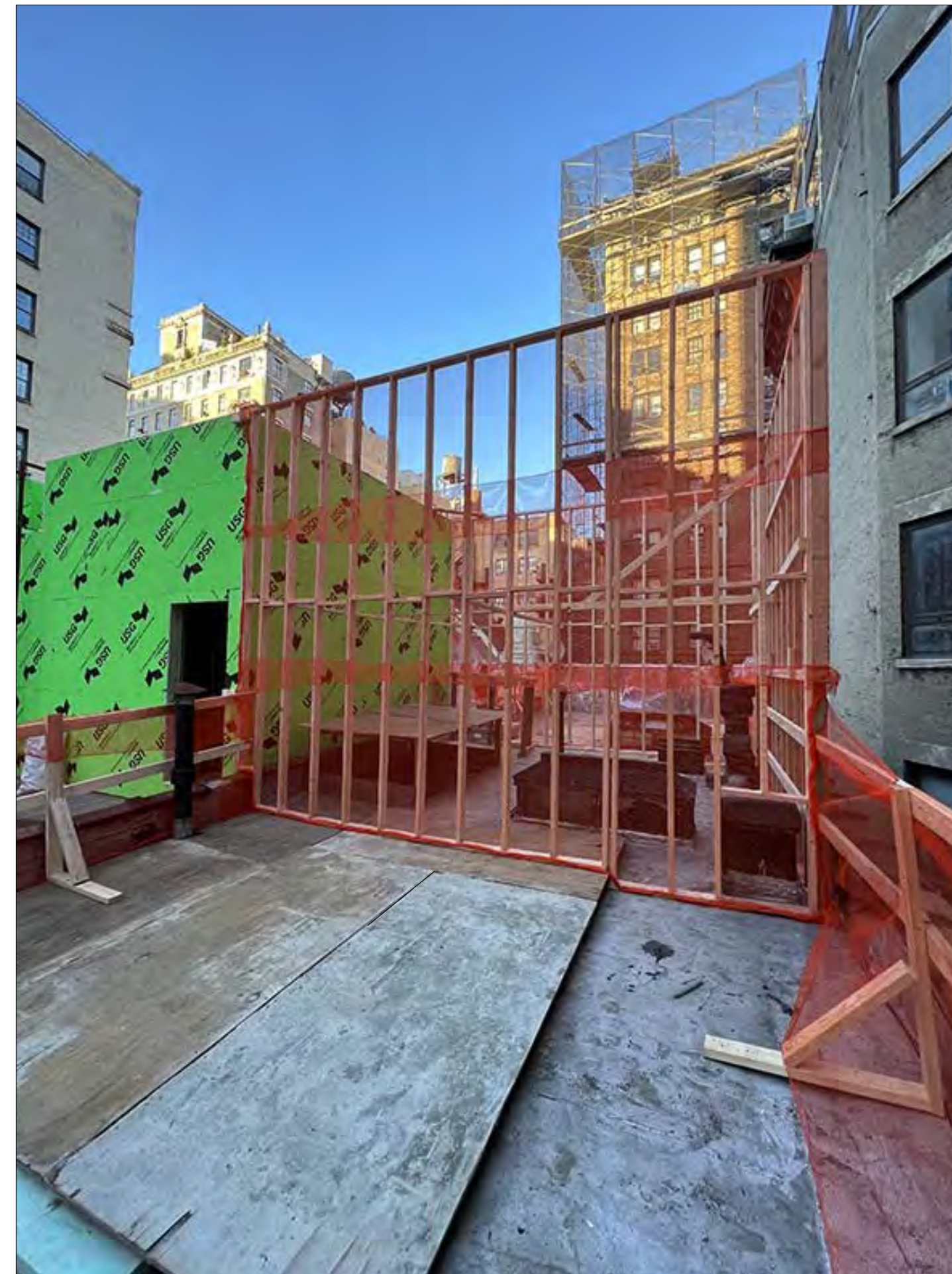
ROOF-LOOKING NORTH WEST
