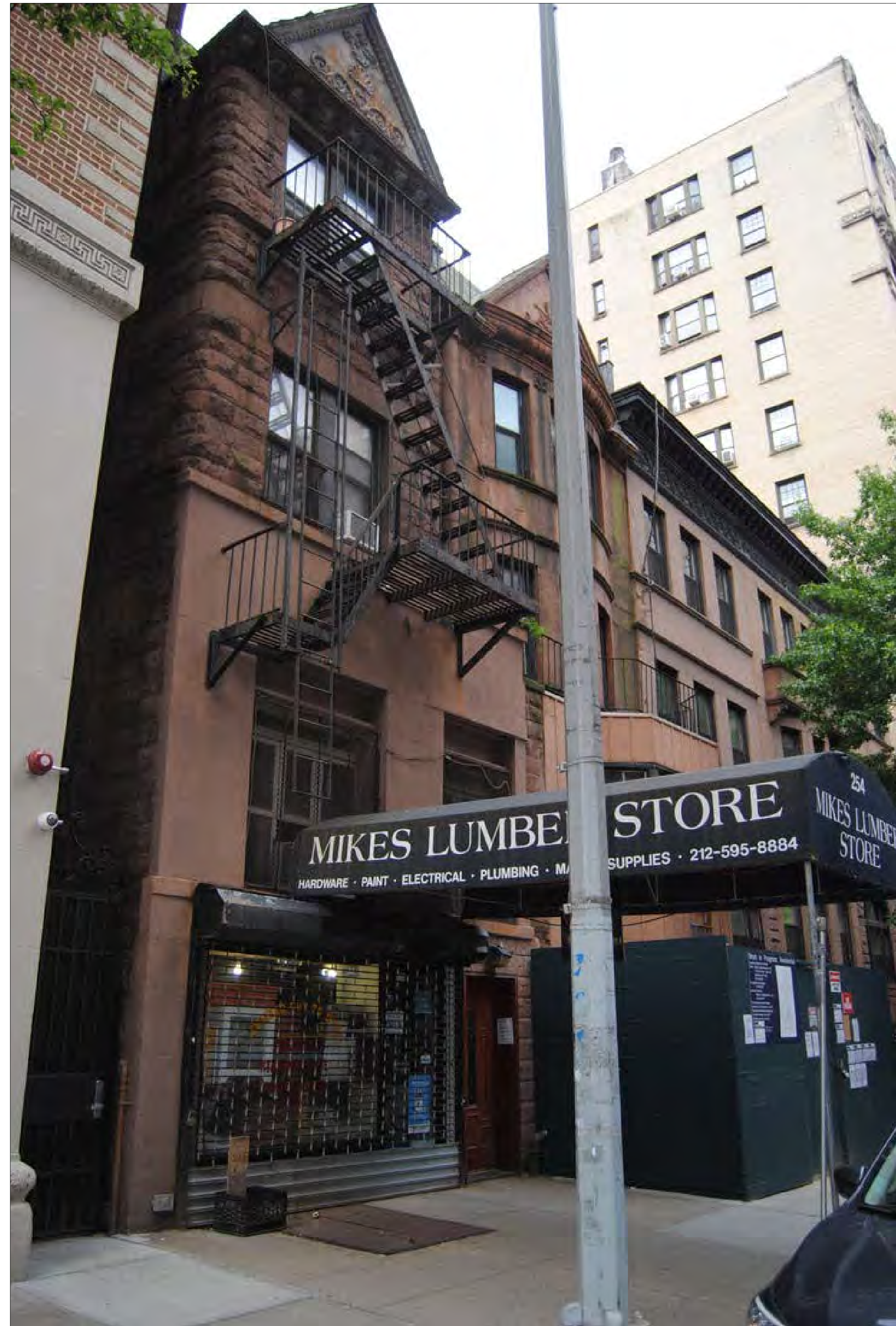
NORTH FACADE LOOKING S.W
