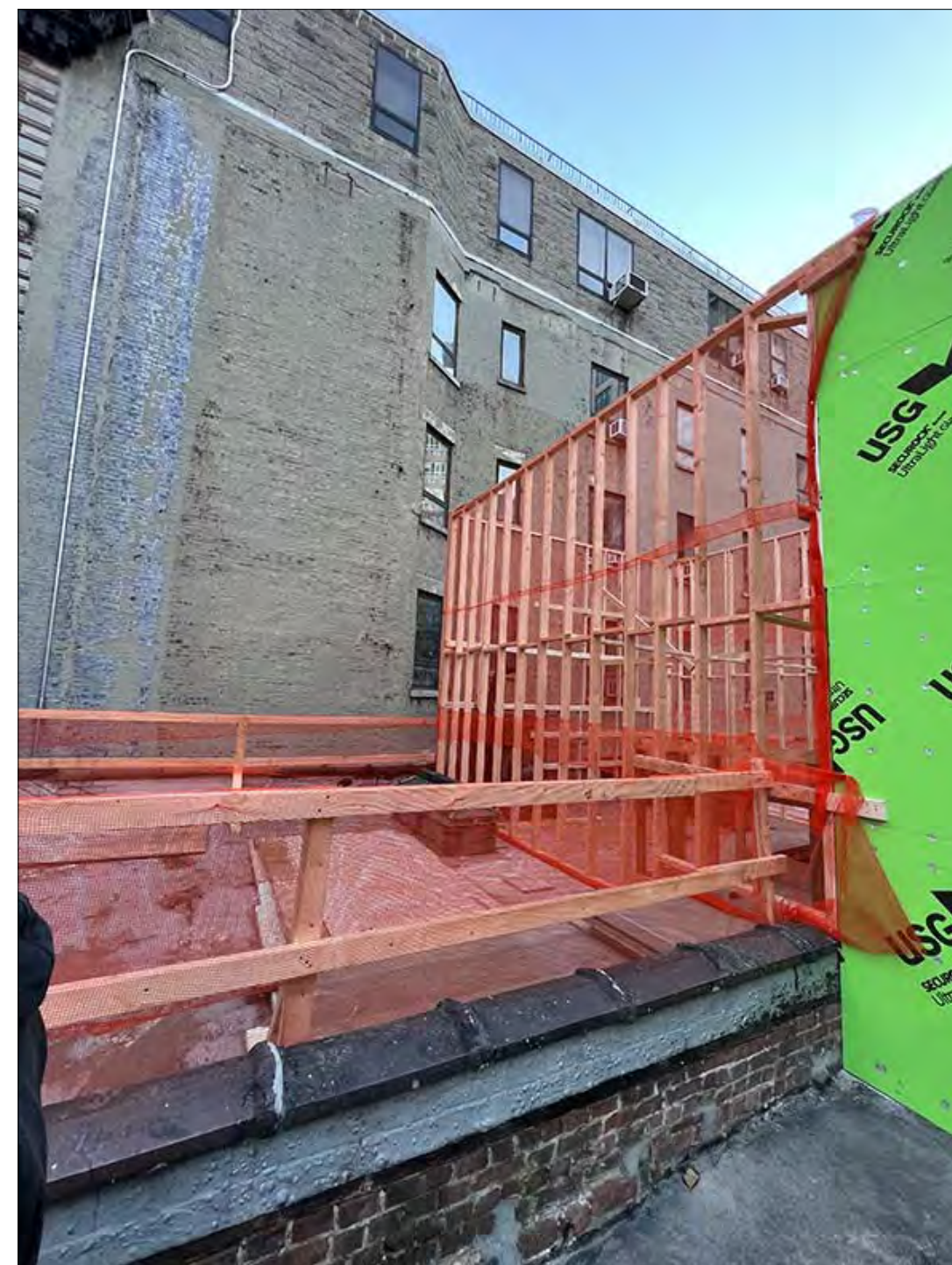
ROOF- LOOKING SOUTH EAST
