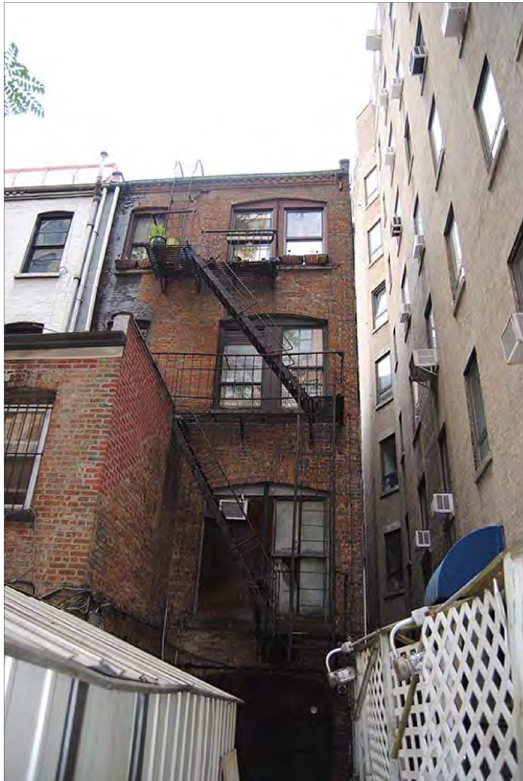
EXISTING SOUTH FACADE
