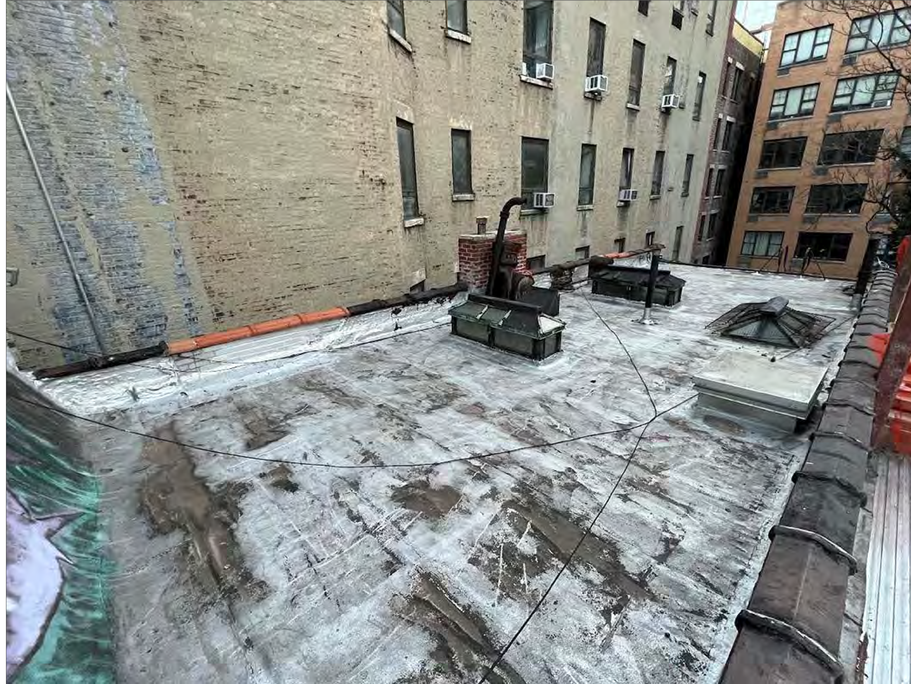
EXISTING ROOF, LOOKING SOUTH
