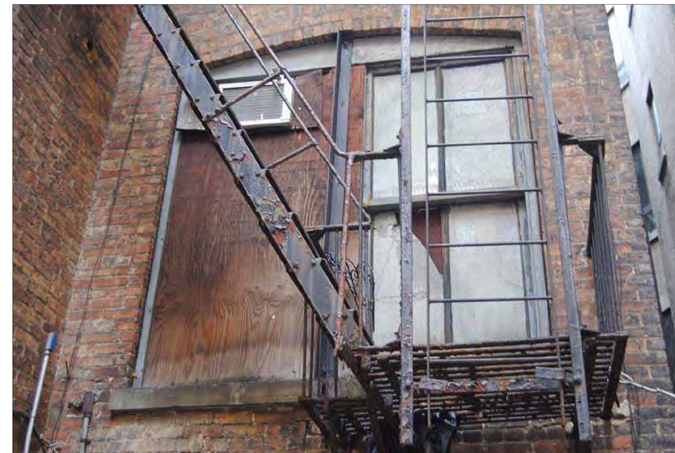
EXISTING ARCHED WINDOW
