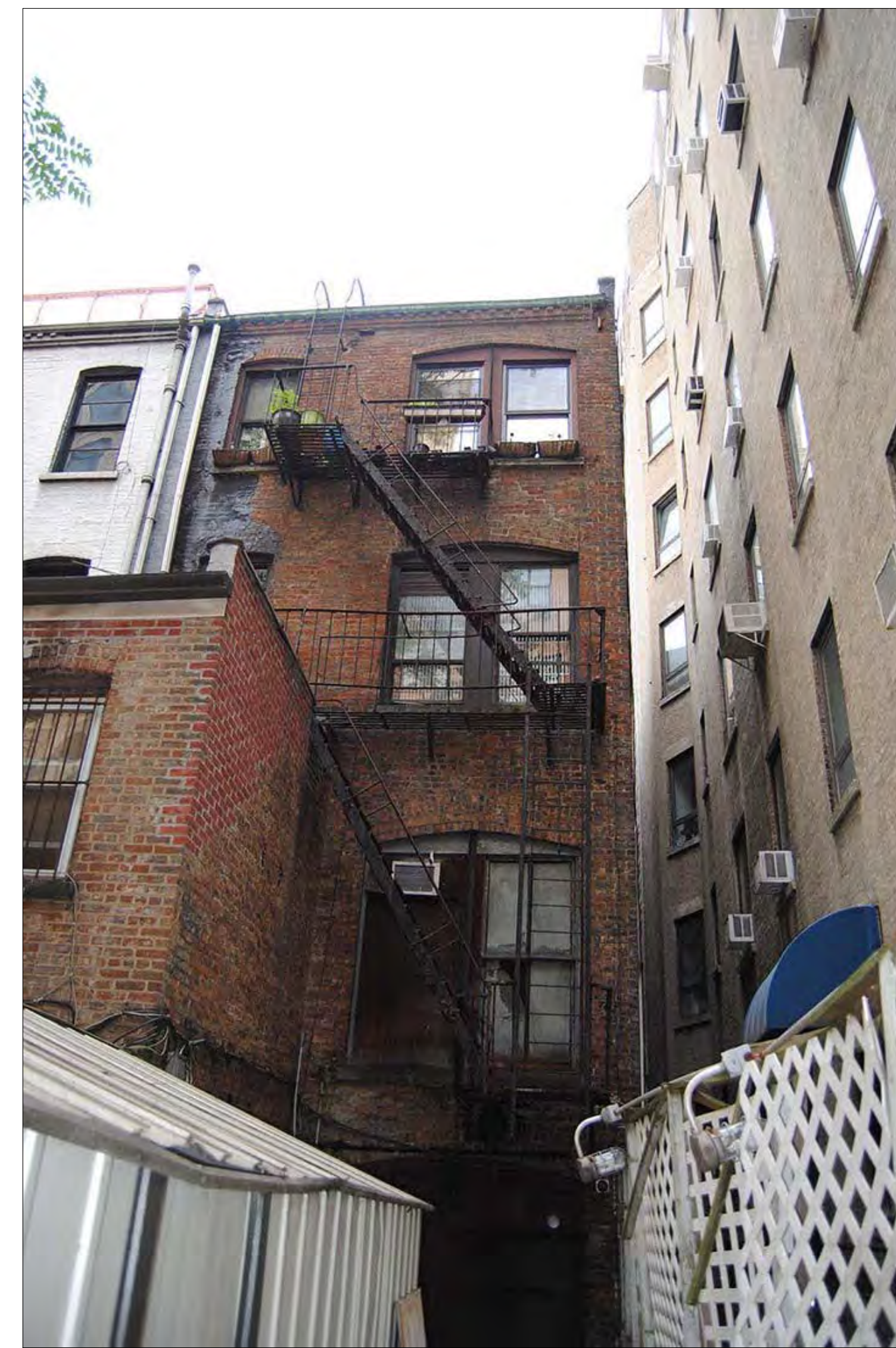
EXISTING SOUTH FACADE
