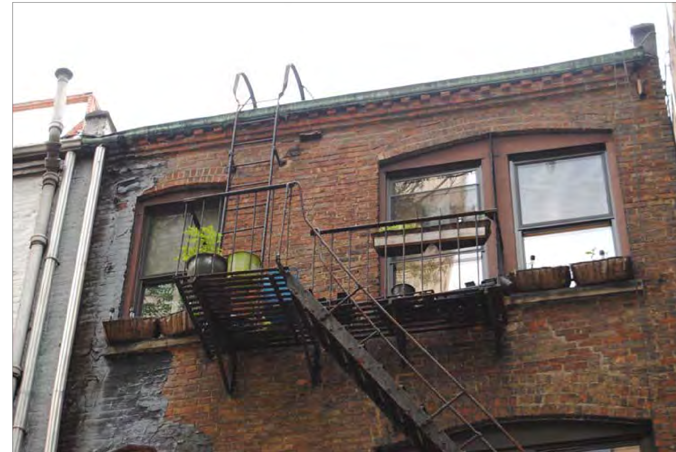
EXISTING BRICK CORBEL
