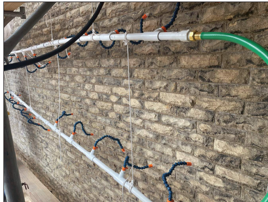
Figure 2. Cleaning mockup after completion.
