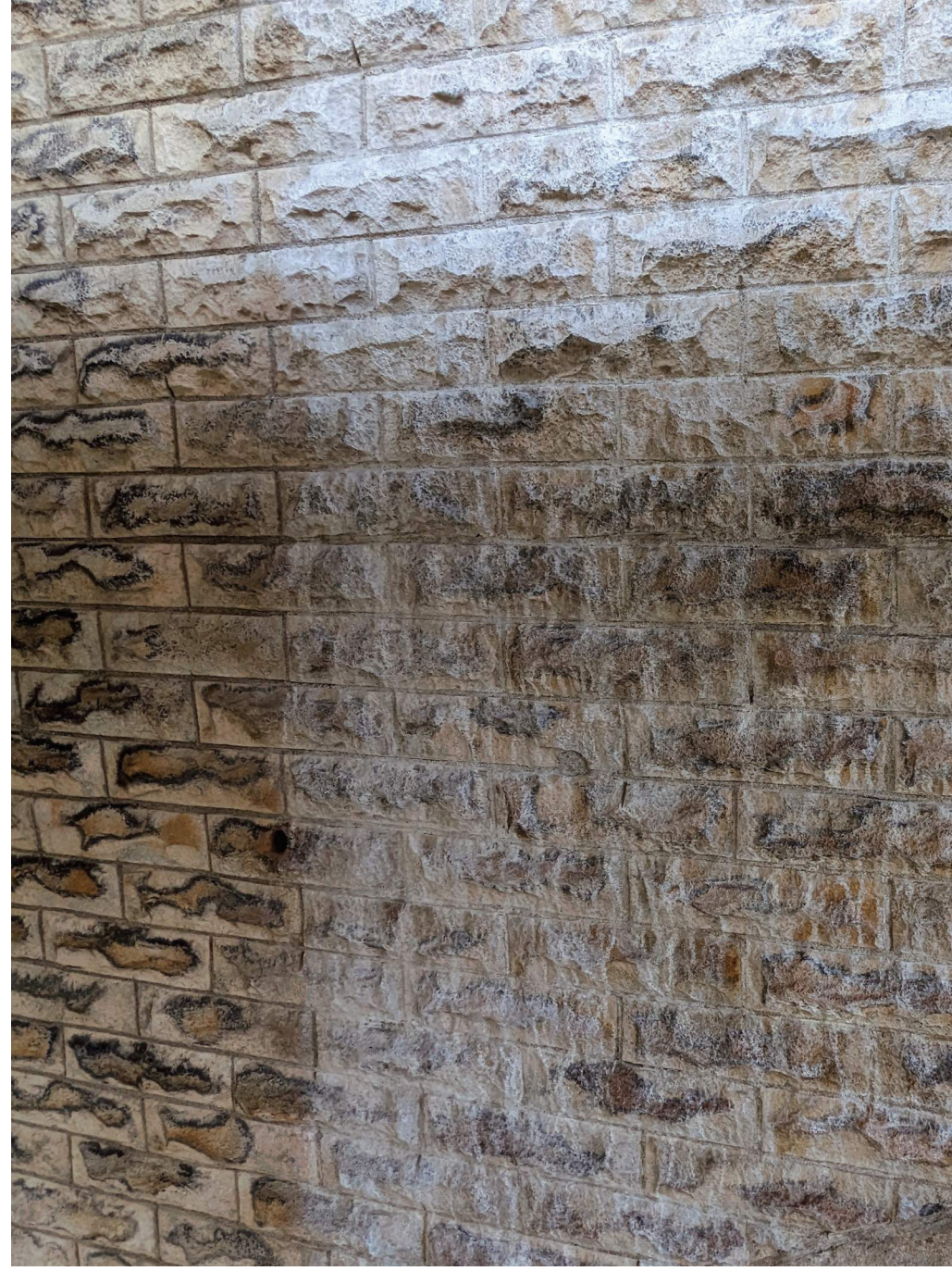
PHOTOS DATED 04/12/2023 SHOWING GYPSUM, LIME, AND COPPER DEPOSITS THROUGHOUT MAIN (NORTH) FACADE
