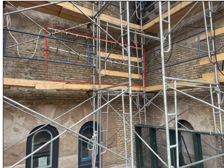
Figure 1. Cleaning mockup (indicated) after completion, from 20' away.
