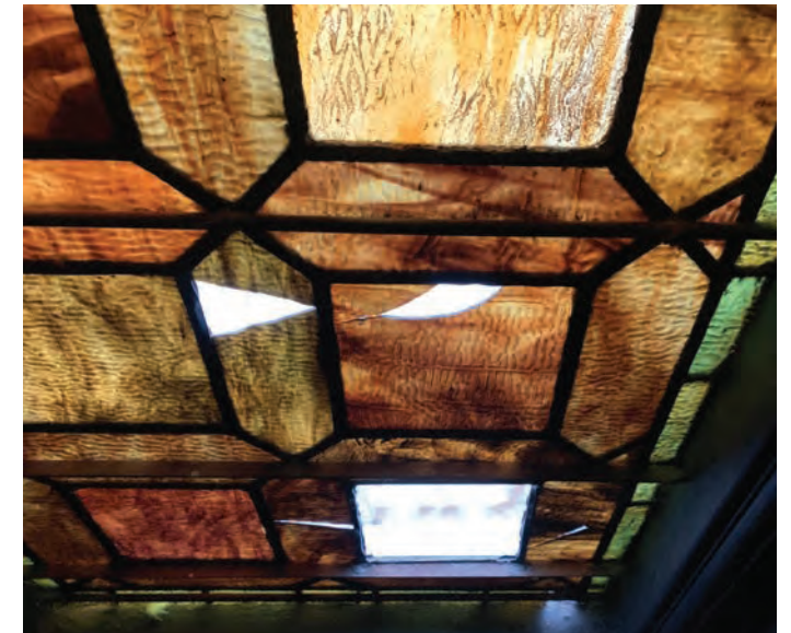
Detail illustrating several lost and unstable glass pieces in window S 13.
