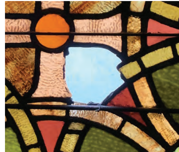
Detail from window S 12 where a piece of glass and the surrounding matrix have been lost. The pieces are unstable.
