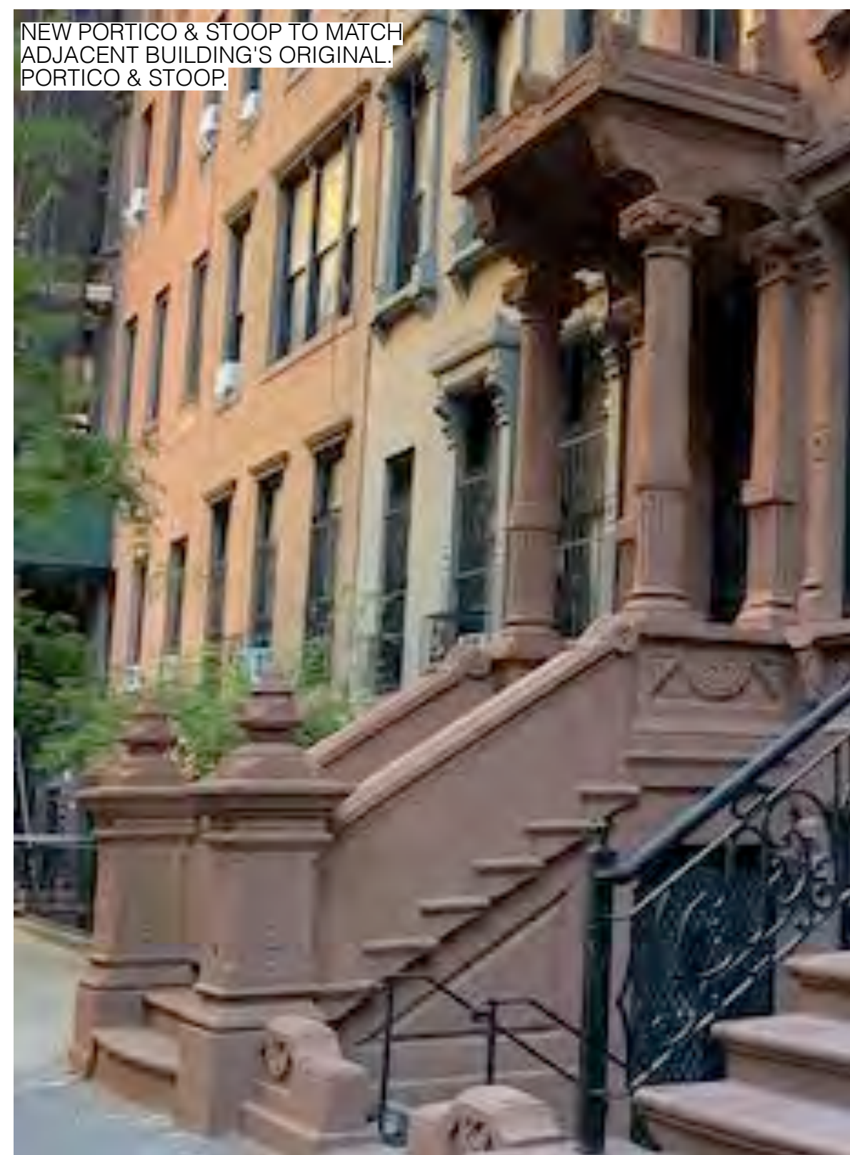
3 CURRENT PHOTO 152 WEST 73RD ST PORITICO LOOKING EAST Scale: NTS
