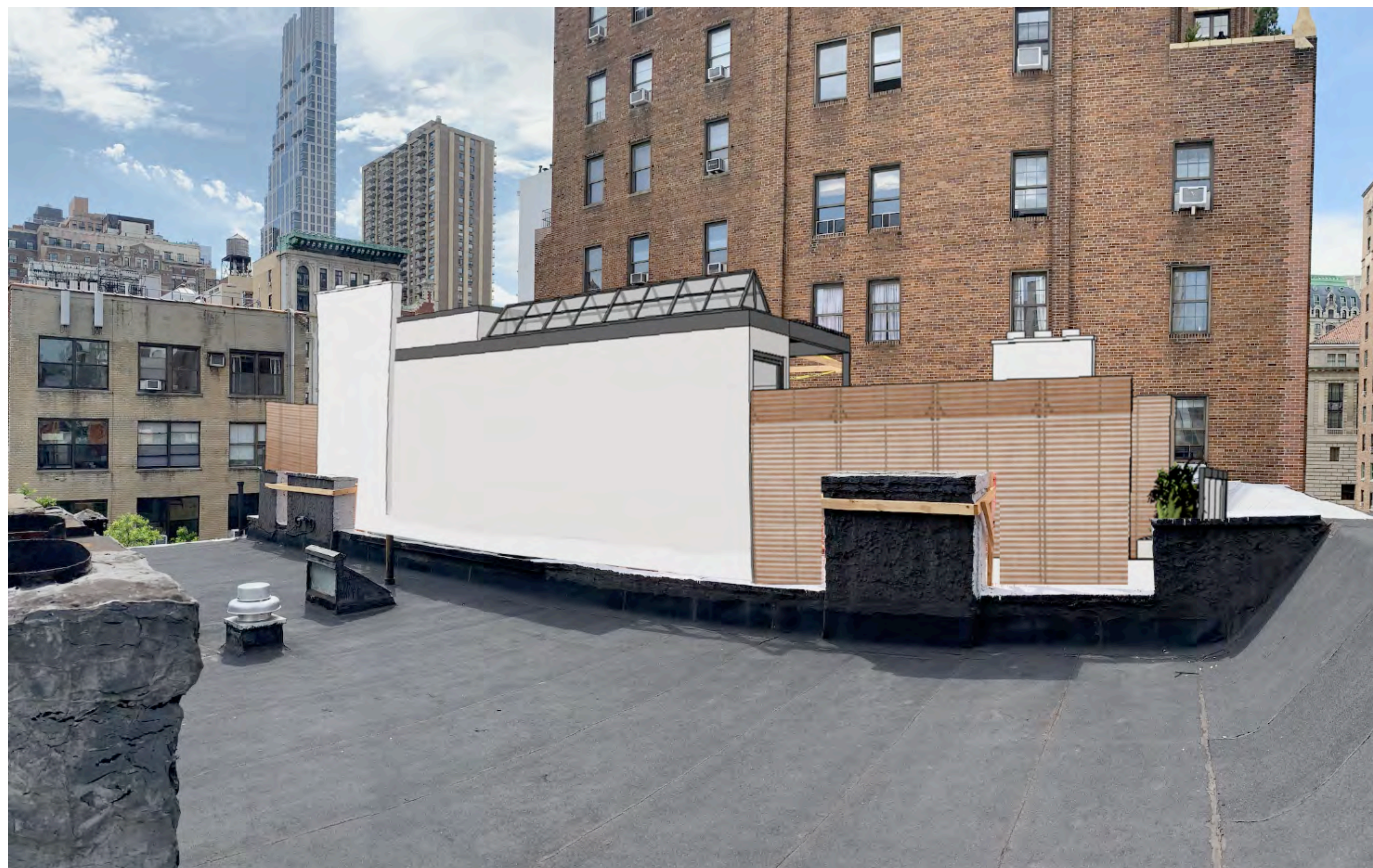
2 VIEW FROM ROOF OF 152 W 73RD ST LOOKING WEST W/ 3D MODEL OVERLAYED IN Scale: NTS
