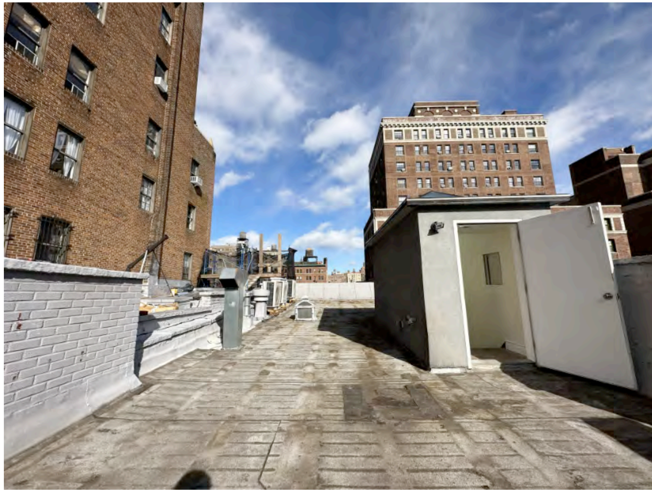
1 PHOTO FROM ROOF LOOKING NORTH Scale: NTS
