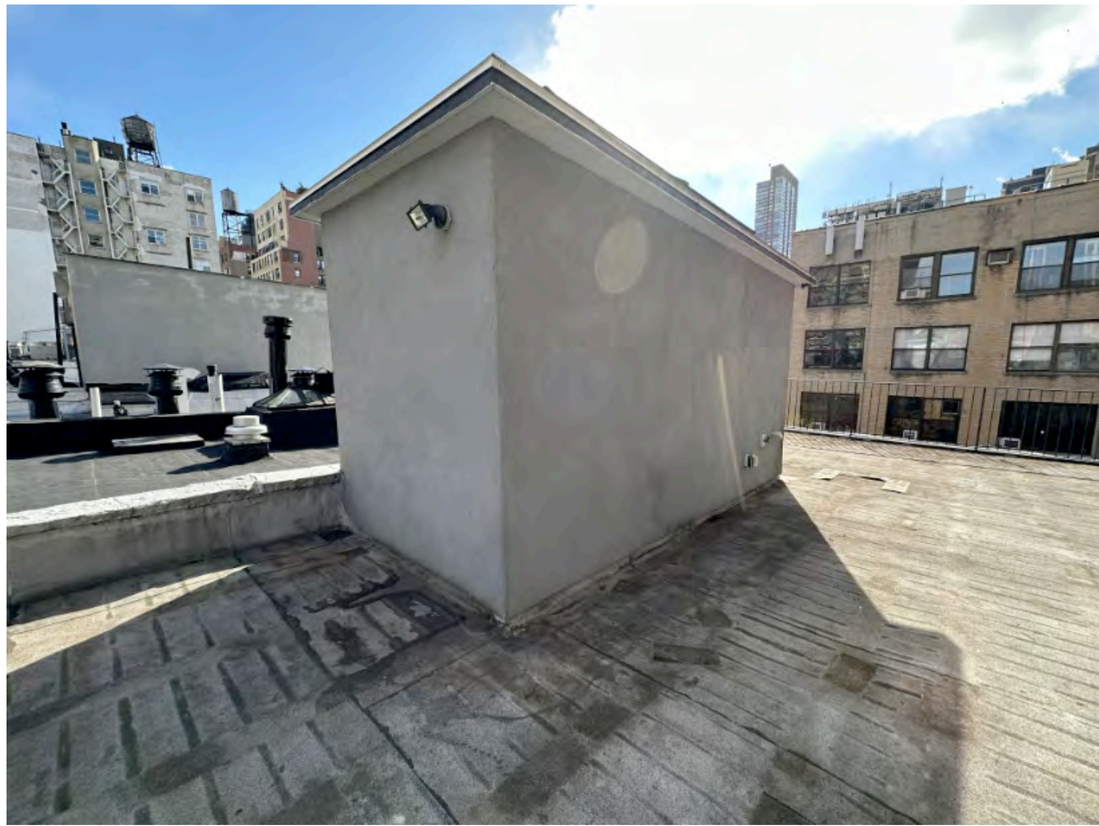
3 PHOTO FROM ROOF LOOKING SOUTH EAST Scale:
