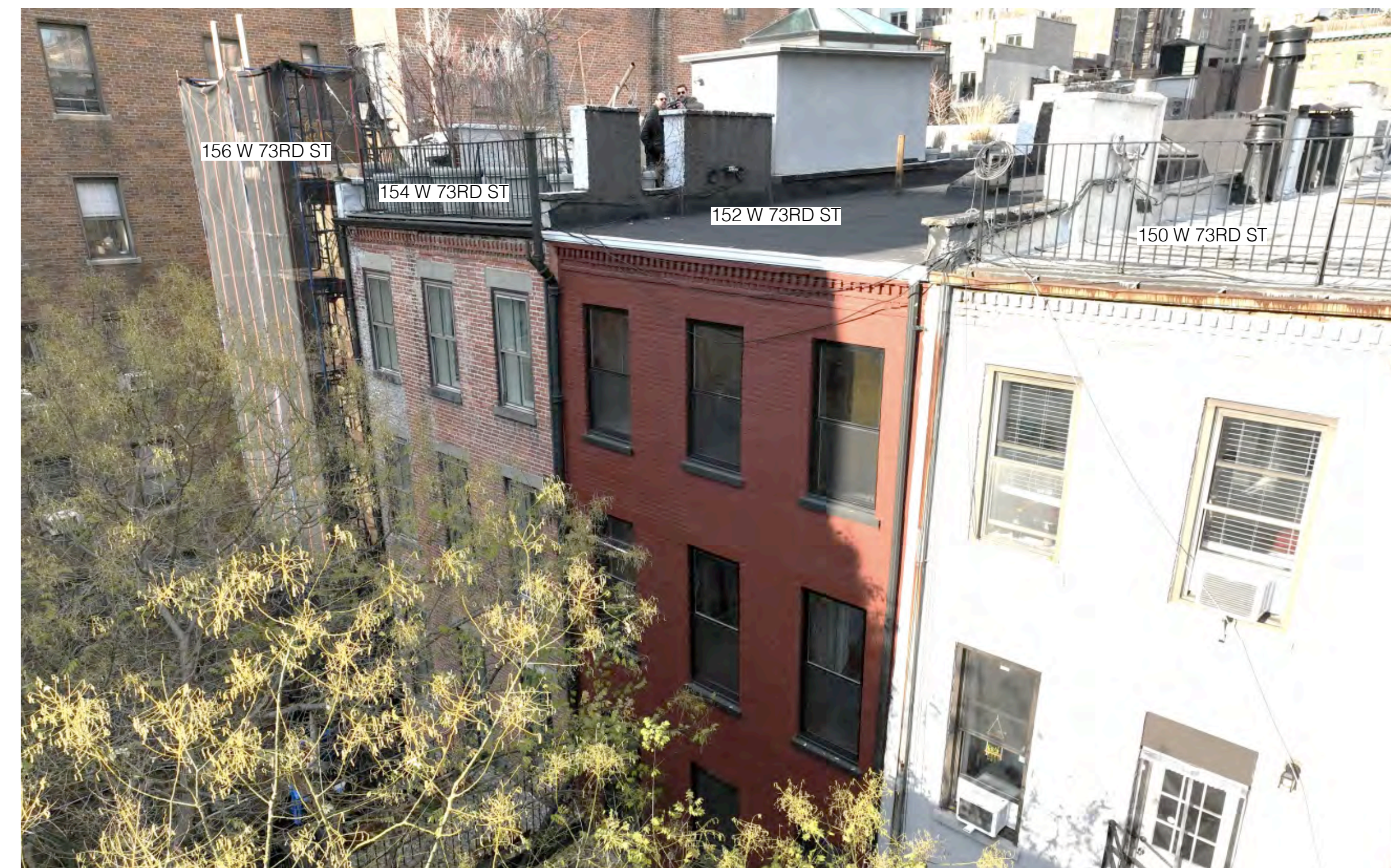
3 EXISTING DRONE PHOTO OF REAR YARD LOOKING NORTHWEST Scale: NTS
