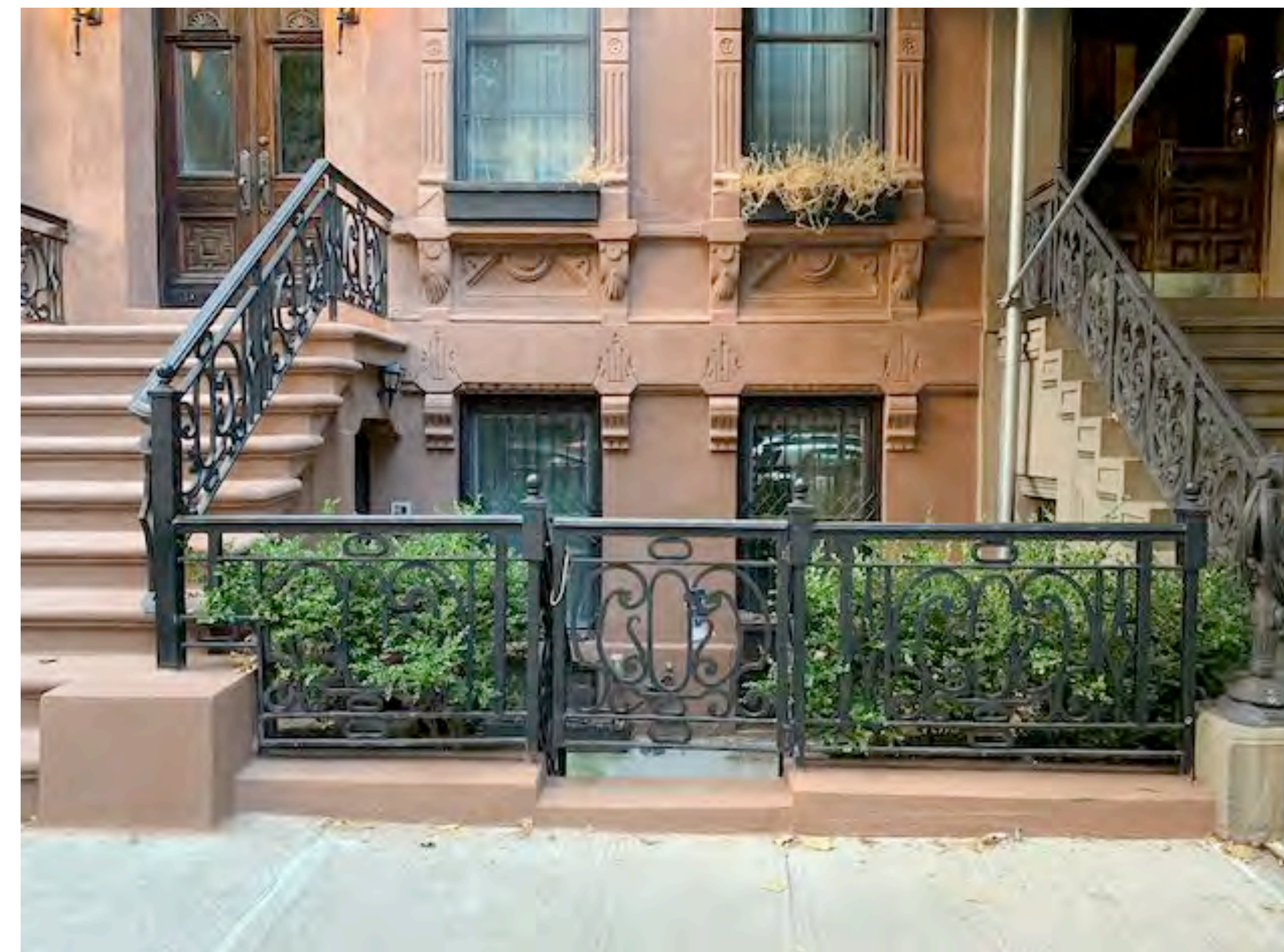
5 CURRENT PHOTO OF EXISTING STOOP 154 WEST 73RD ST. LOOKING SOUTH Scale: NTS
