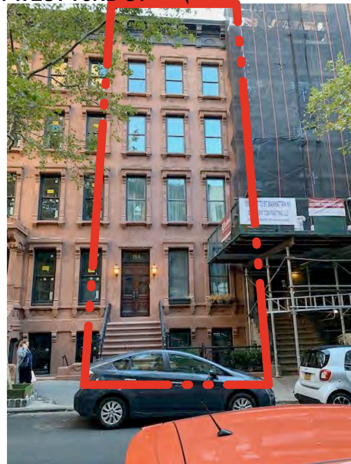
6 CURRENT PHOTO LOOKING SOUTH Scale: NTS
