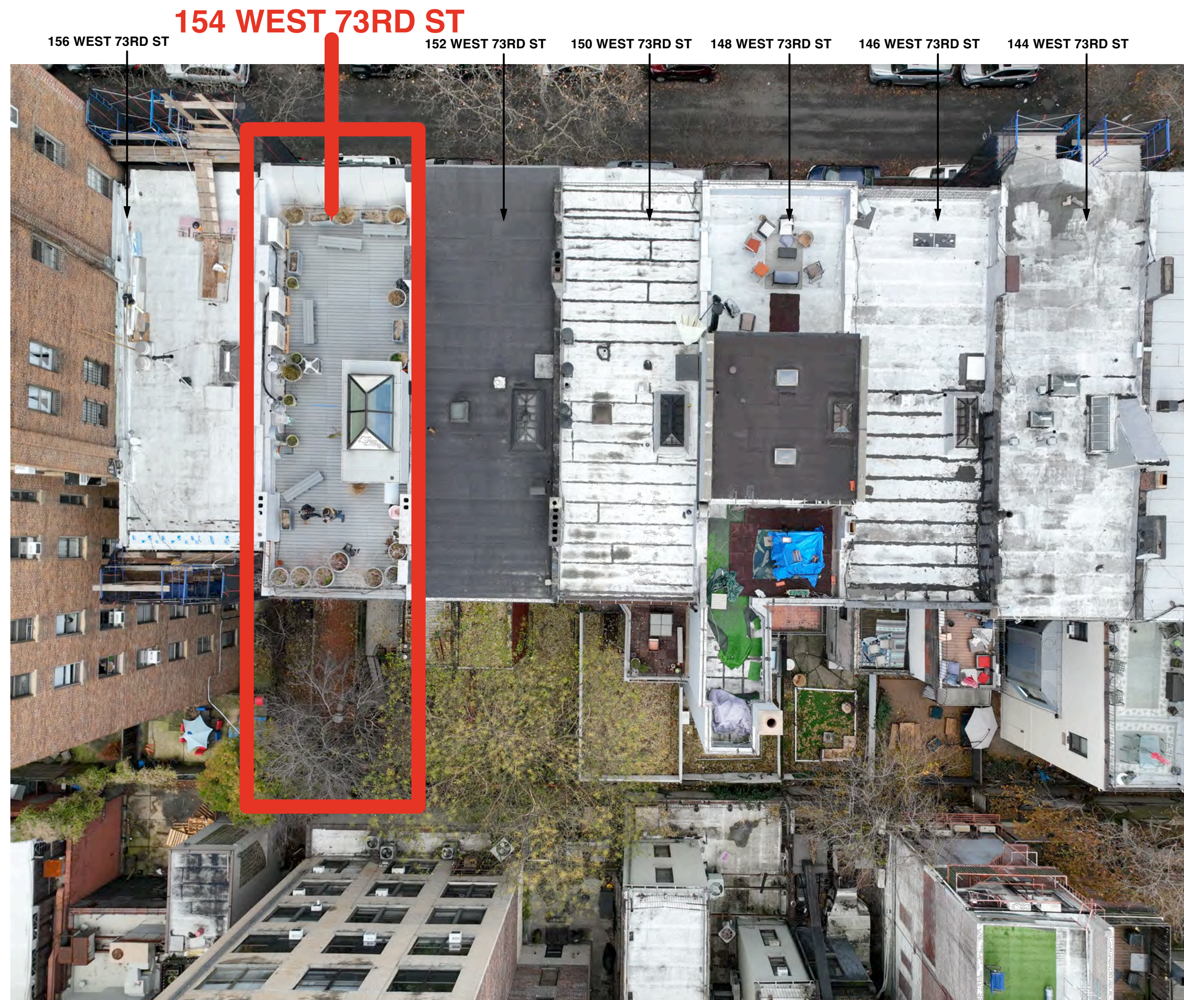
1 OVERHEAD DRONE PHOTO Scale: NTS
