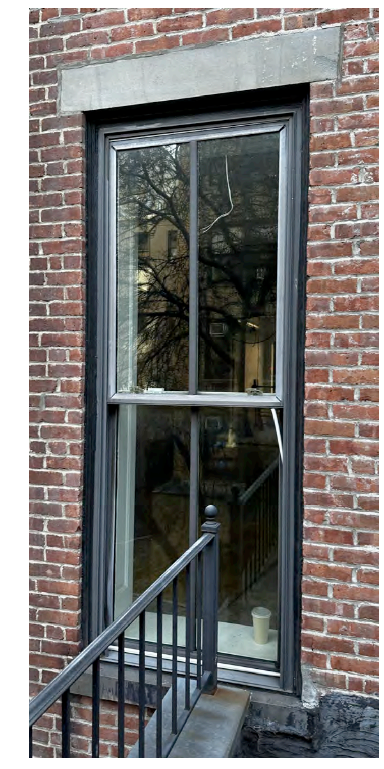
3 PHOTO OF TYP. EXISTING REAR FACADE WINDOW Scale:
