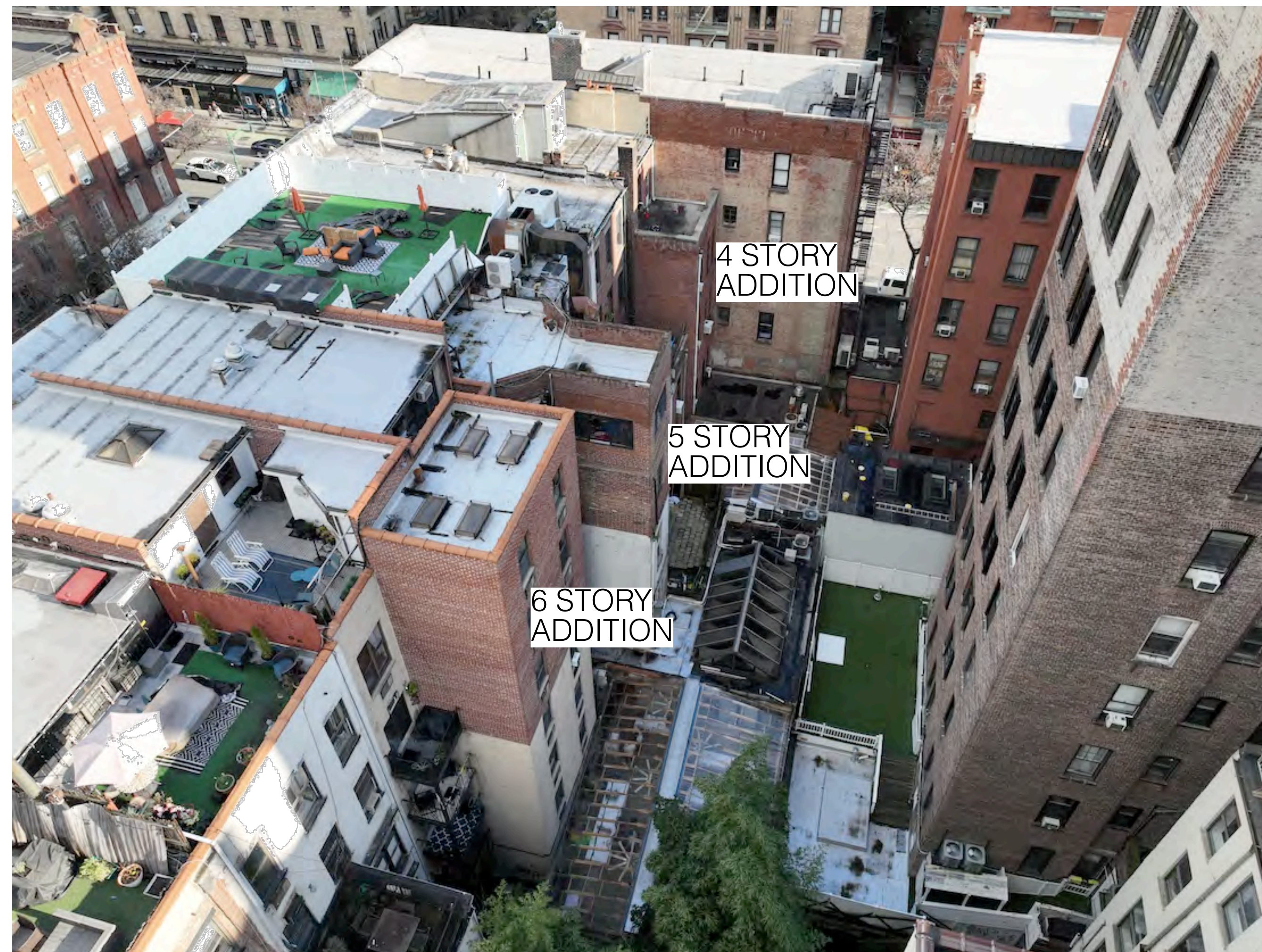
2 DRONE VIEW OF 'DONUT' LOOKING EAST Scale: NTS
