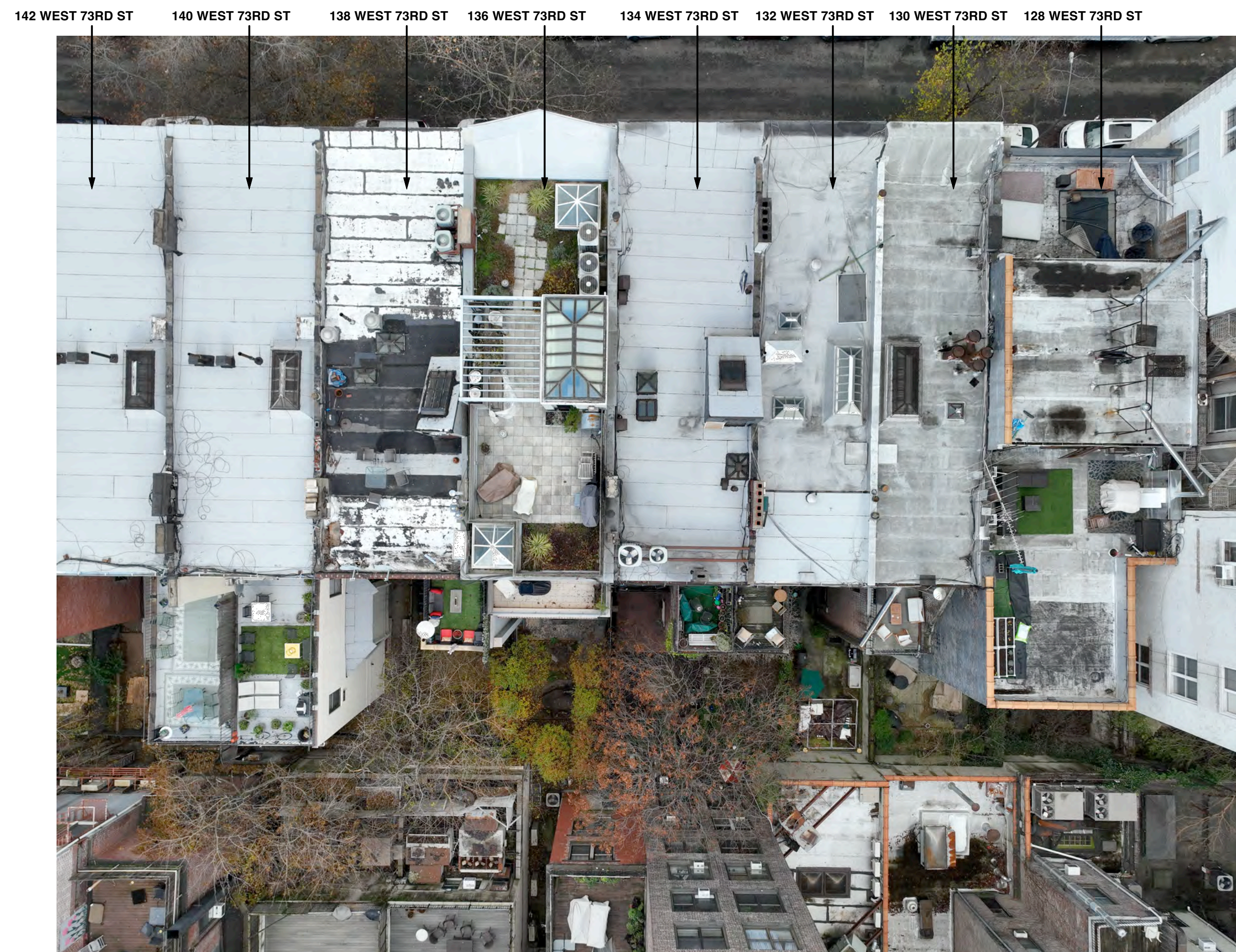
2 OVERHEAD DRONE PHOTO Scale: NTS
