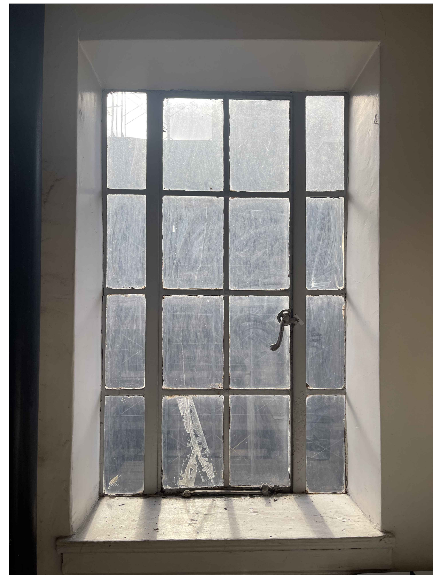
Existing Photograph Types C
