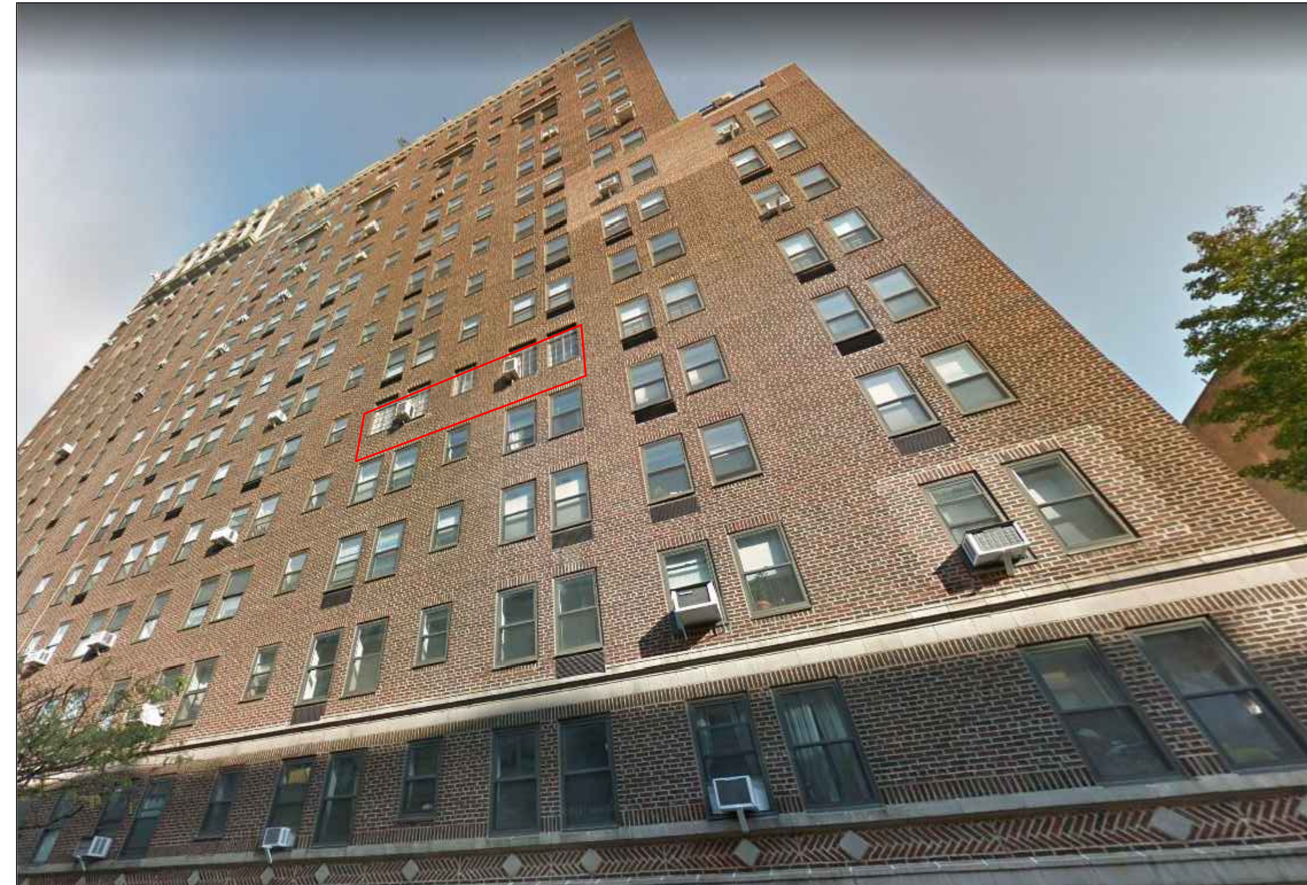
West 95th Street Facade-
