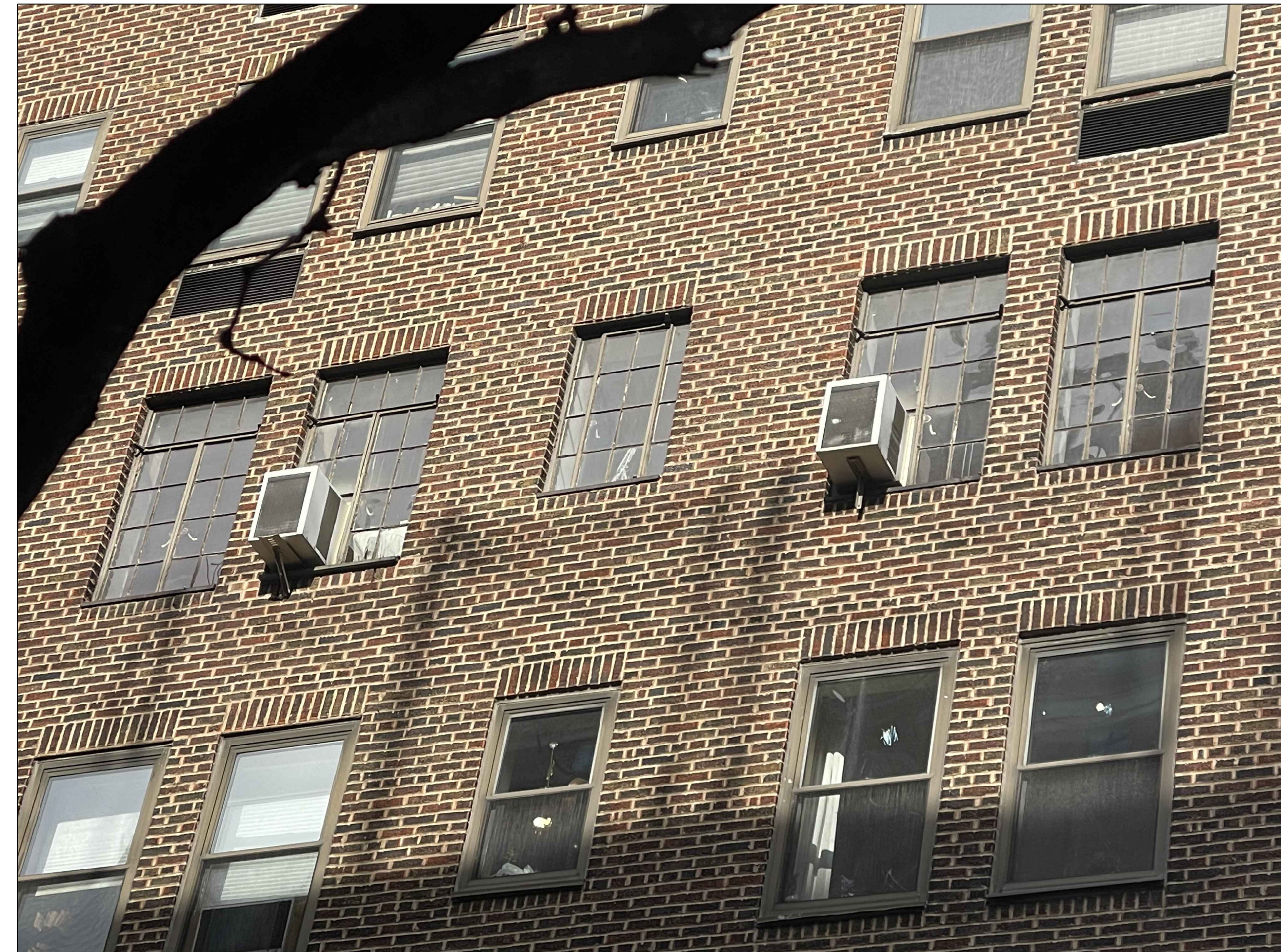
Exterior view of windows in scope of work
