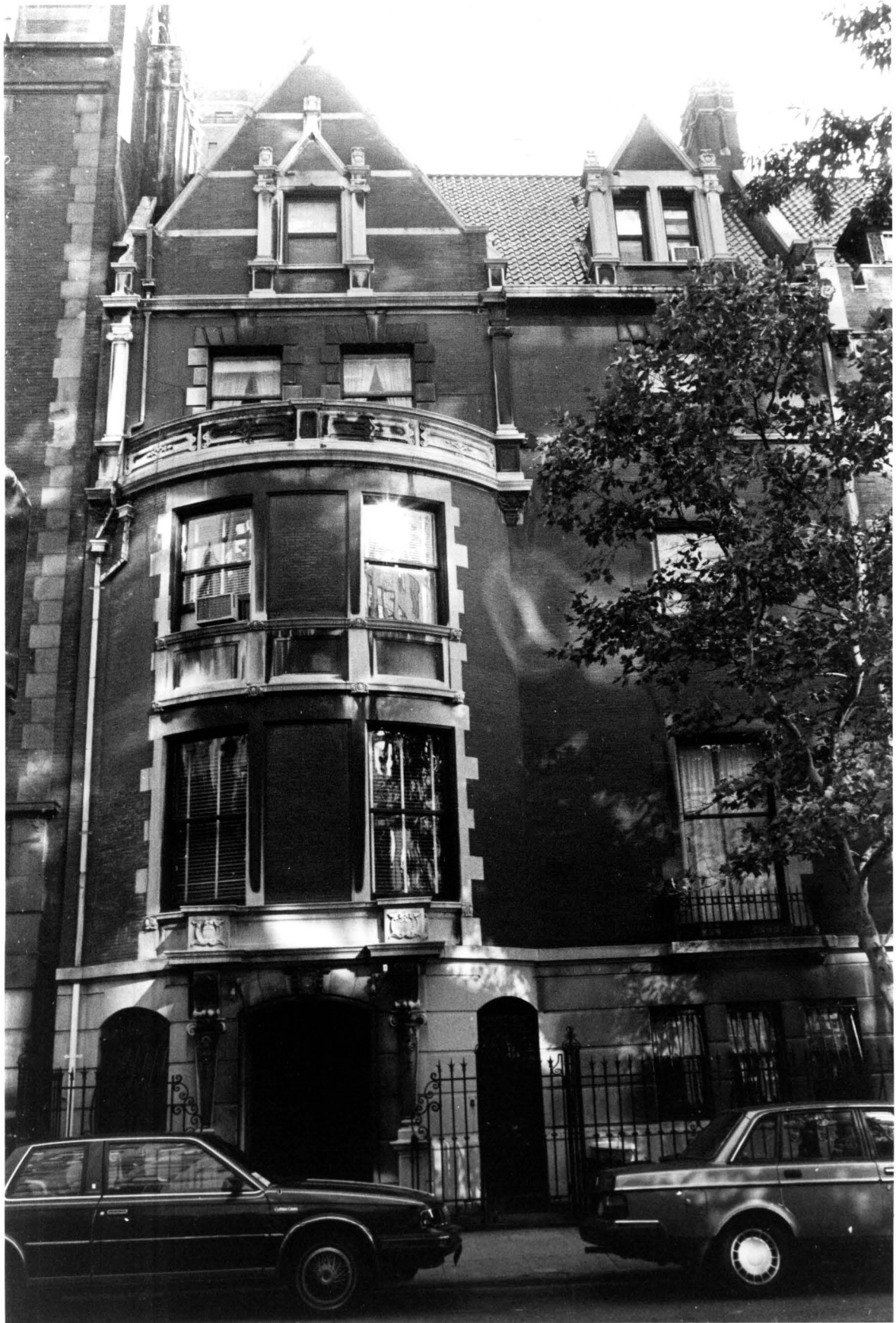
332 West 83rd Street House Architect: Clarence True Built: 1898-99 Photo: Lynne Marthey
