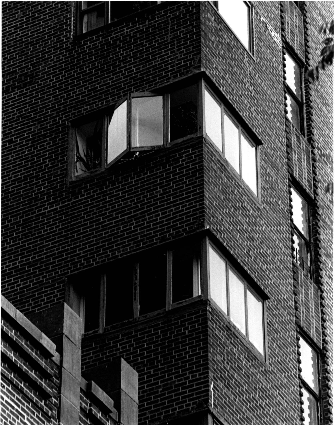
The Master Building 310-312 Riverside Drive; original windows at northwest corner 1928-29; Helmle, Corbett & Harrison with Sugarman & Berger Photo Credit: Carl Forster
