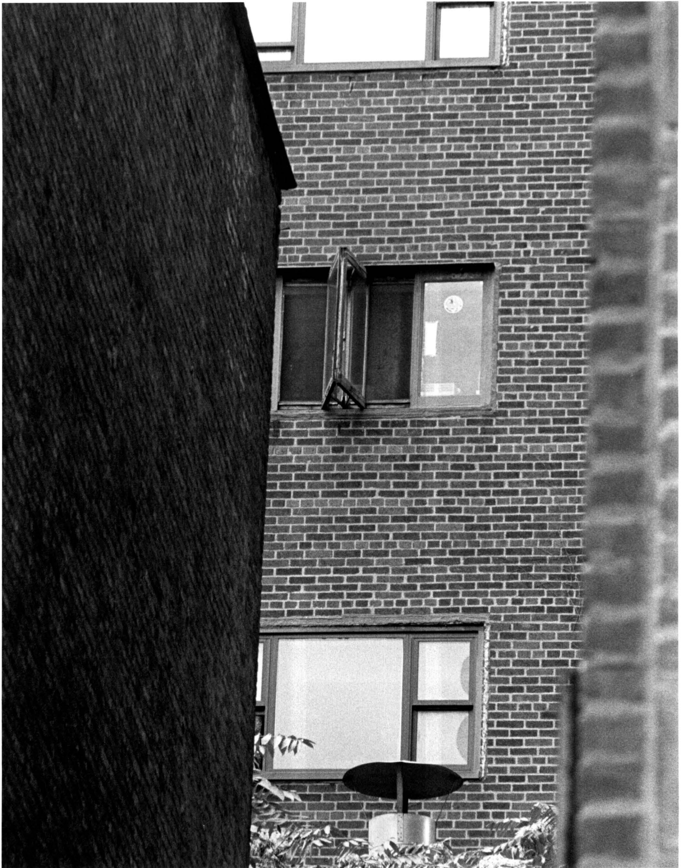
The Master Building 310-312 Riverside Drive; original windows at northeast corner 1928-29; Helmle, Corbett & Harrison with Sugarman & Berger Photo Credit: Carl Forster
