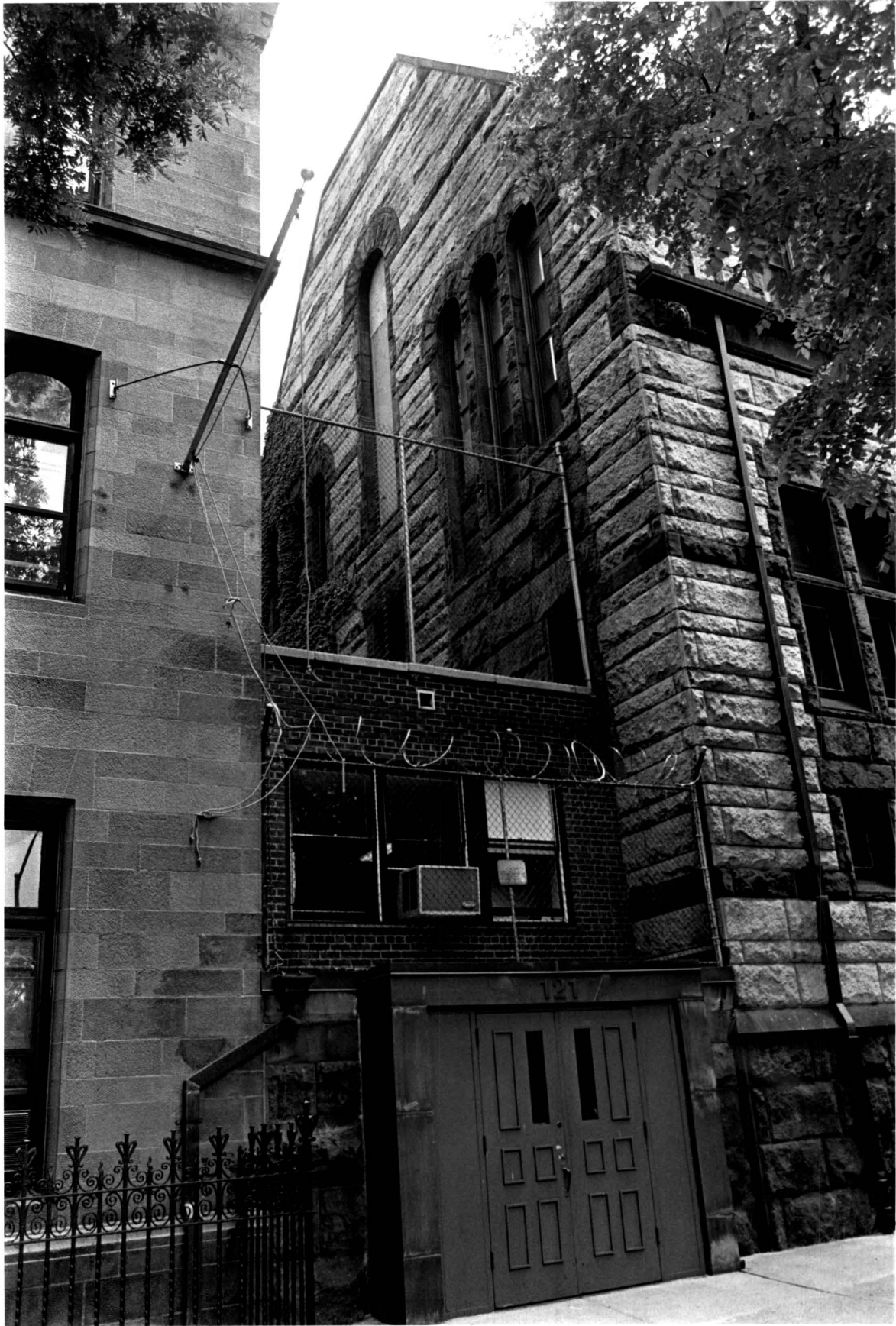
121 West 91st Street Structure joining Trinity School and the Former St. Agnes Parish House, not part of Landmark Site.
