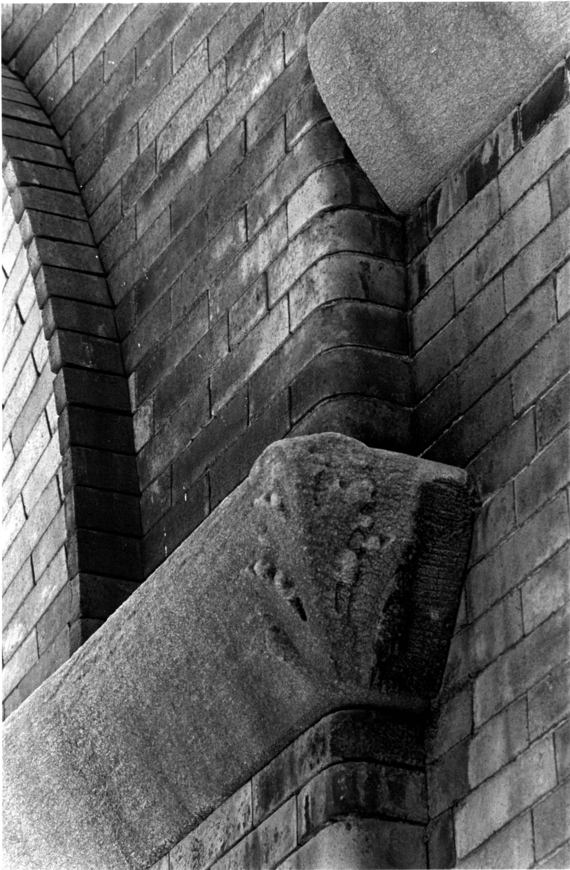
Claremont Stables (now Claremont Riding Academy) Detail of an Impost Block
