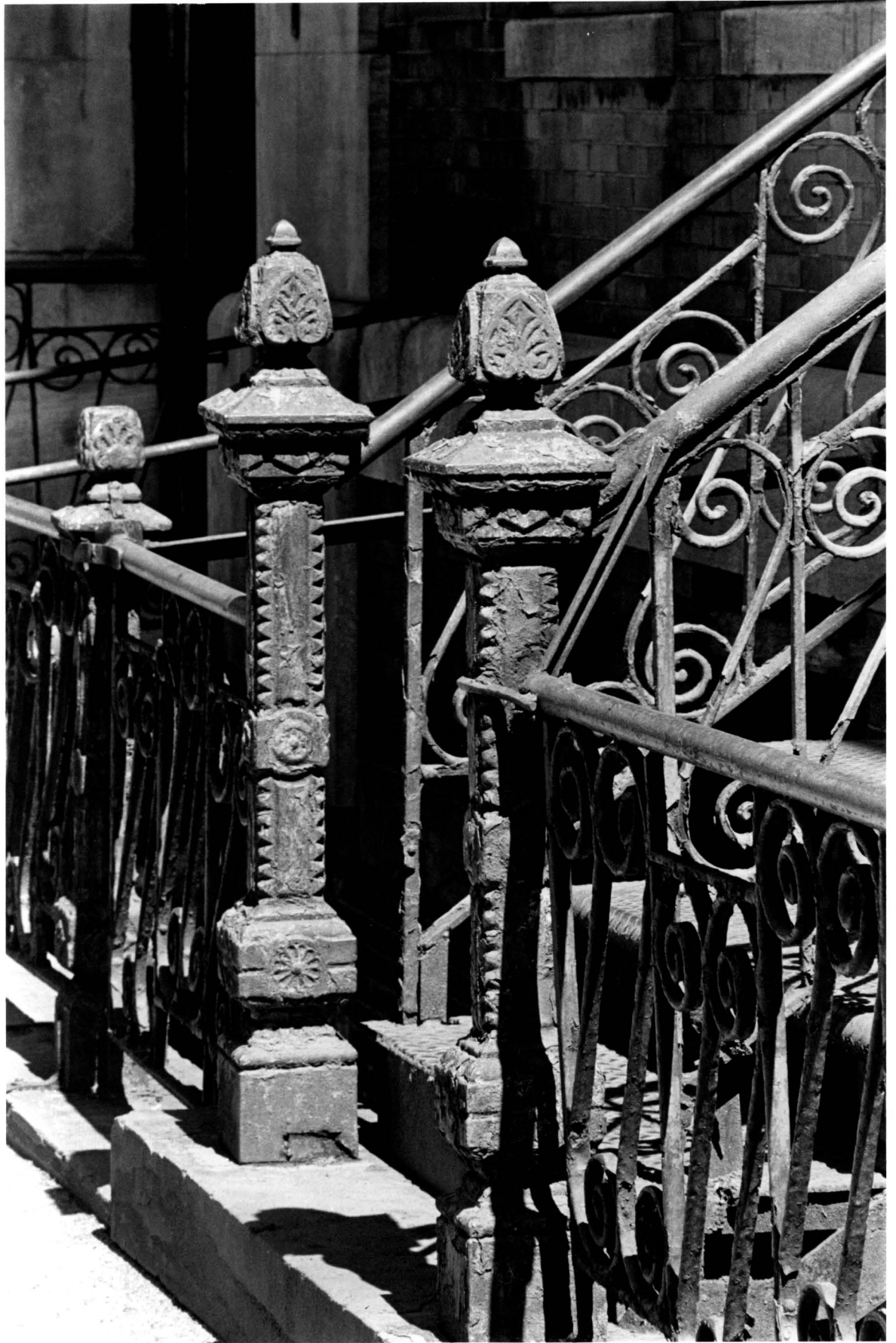
Claremont Stables (now Claremont Riding Academy) Detail of iron fence
