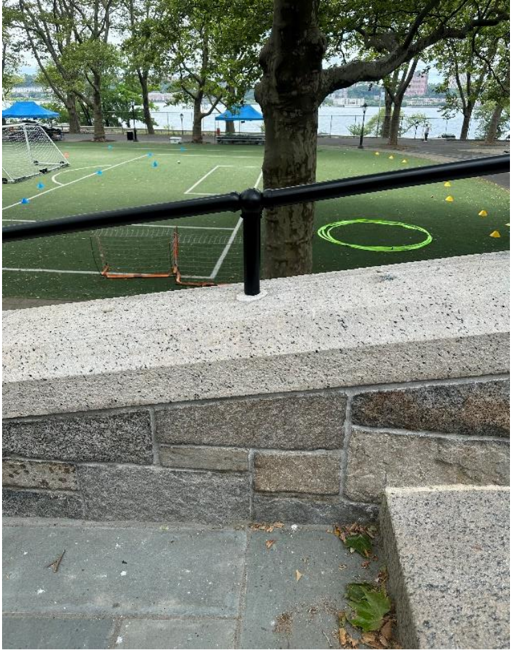
New Custom Guardrail replicates the guardrail at the adjacent retaining wall
