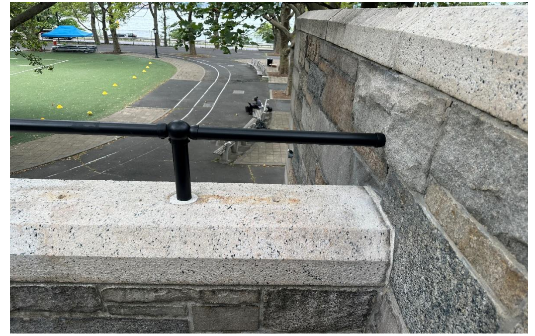
Guardrail recently installed at identical stair at 102 nd Street
