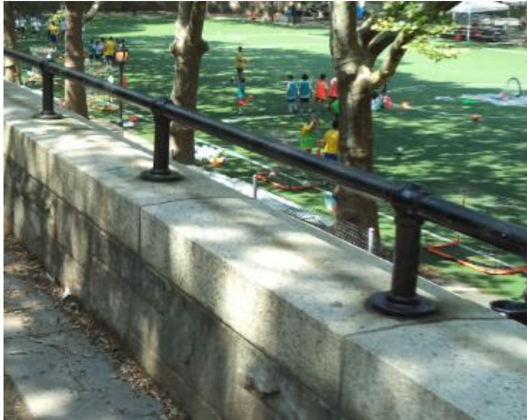
Existing Historic Guardrail on the retaining wall at 102 nd Street
