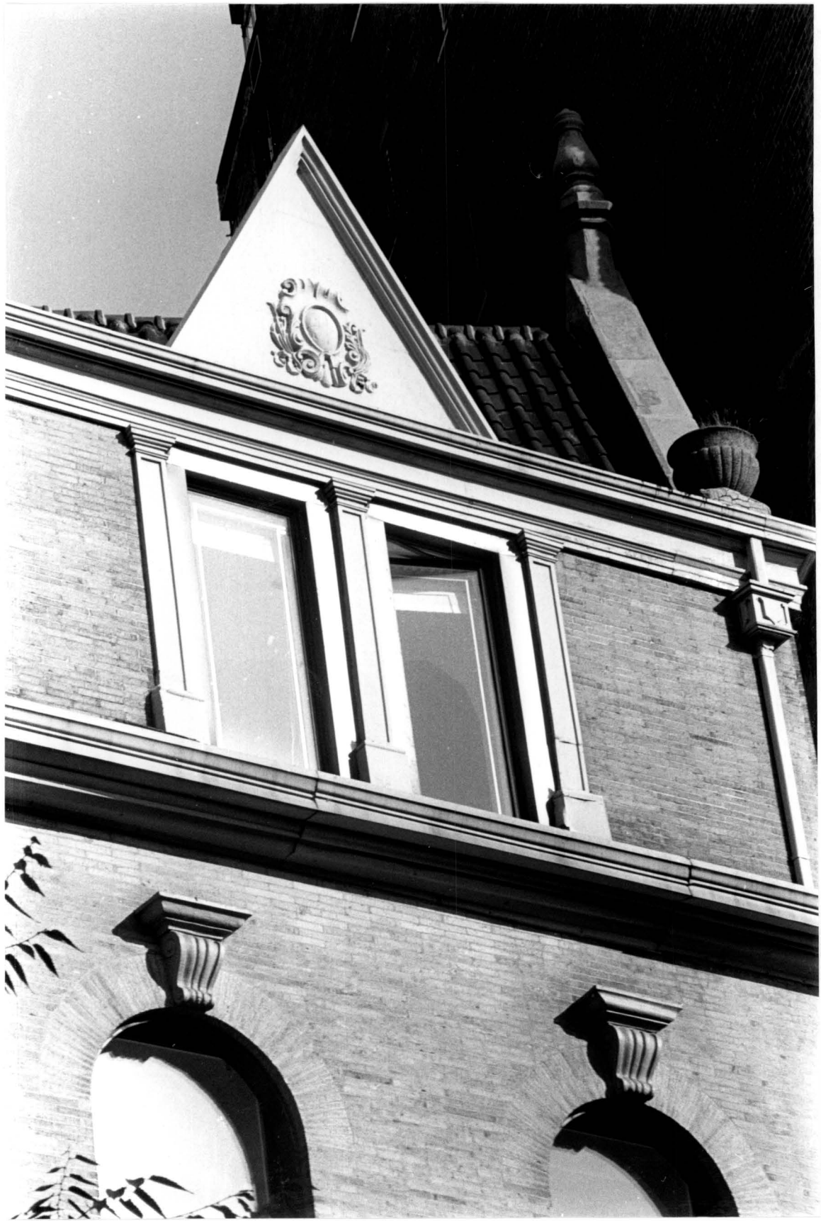
103 Riverside Drive House Dormer Detail on West Facade
