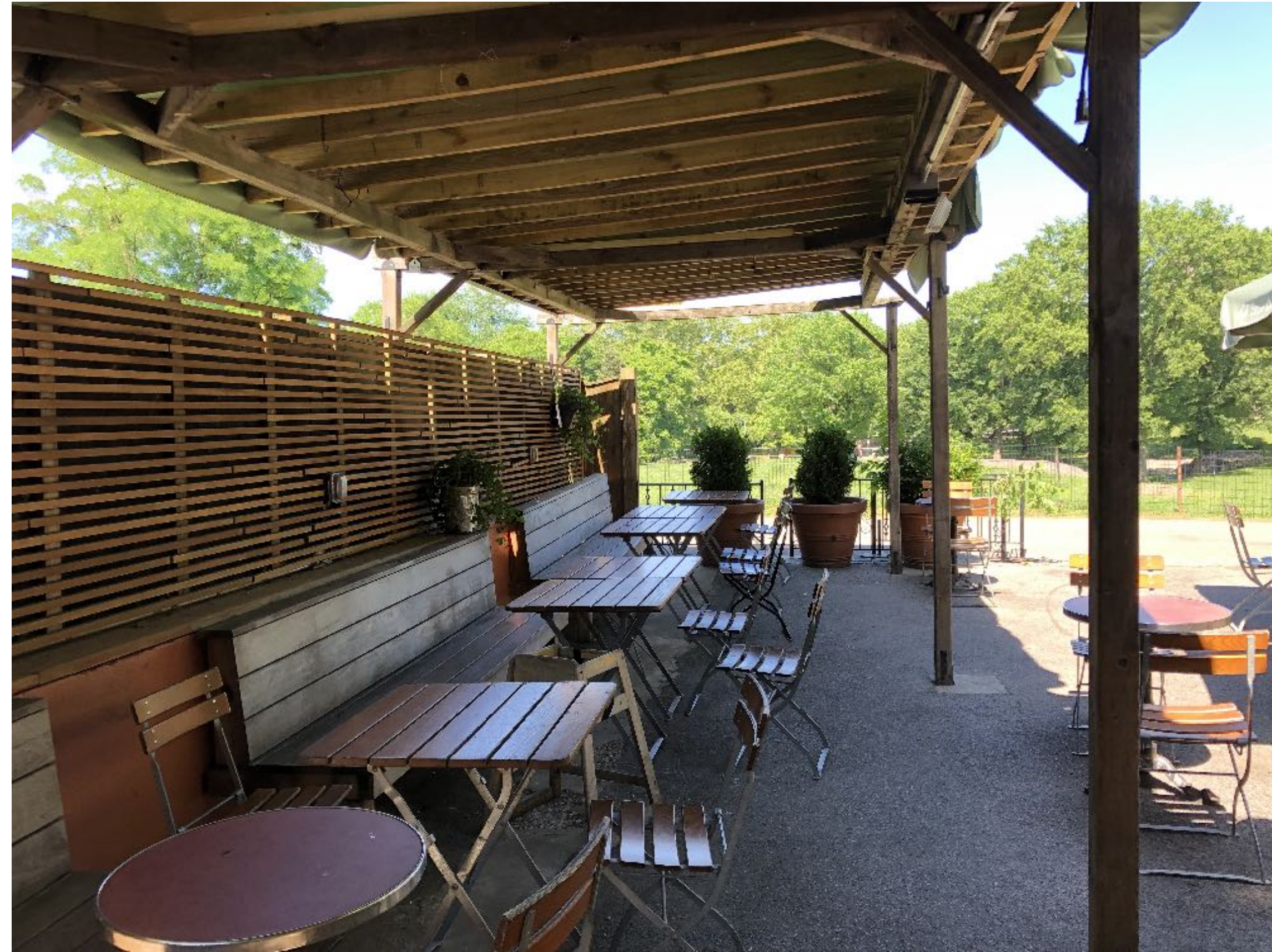
A EXISTING CONDITIONS PHOTO_PERGOLA
