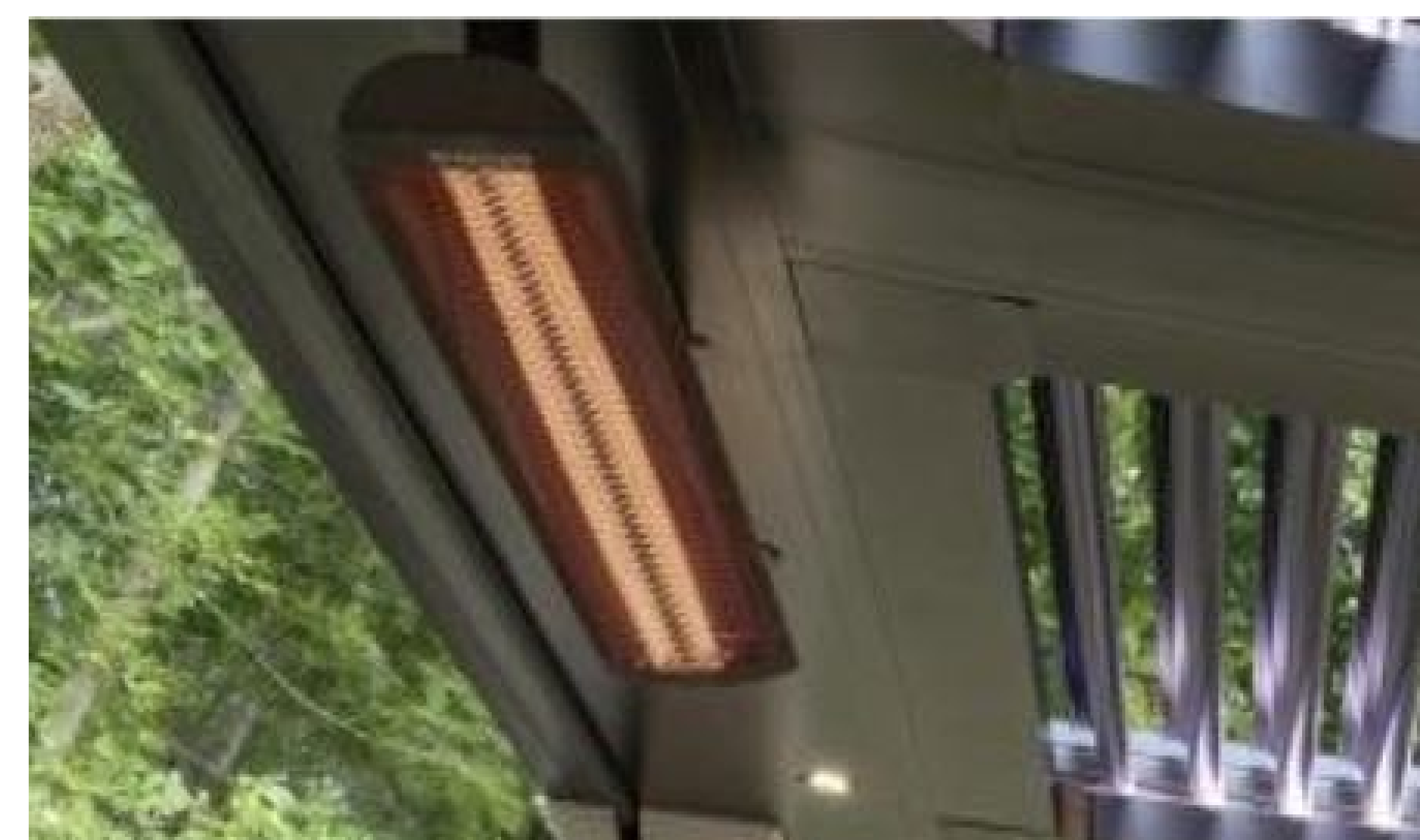
E CEILING MOUNTED HEATERS TO PERGOLA BEAM
