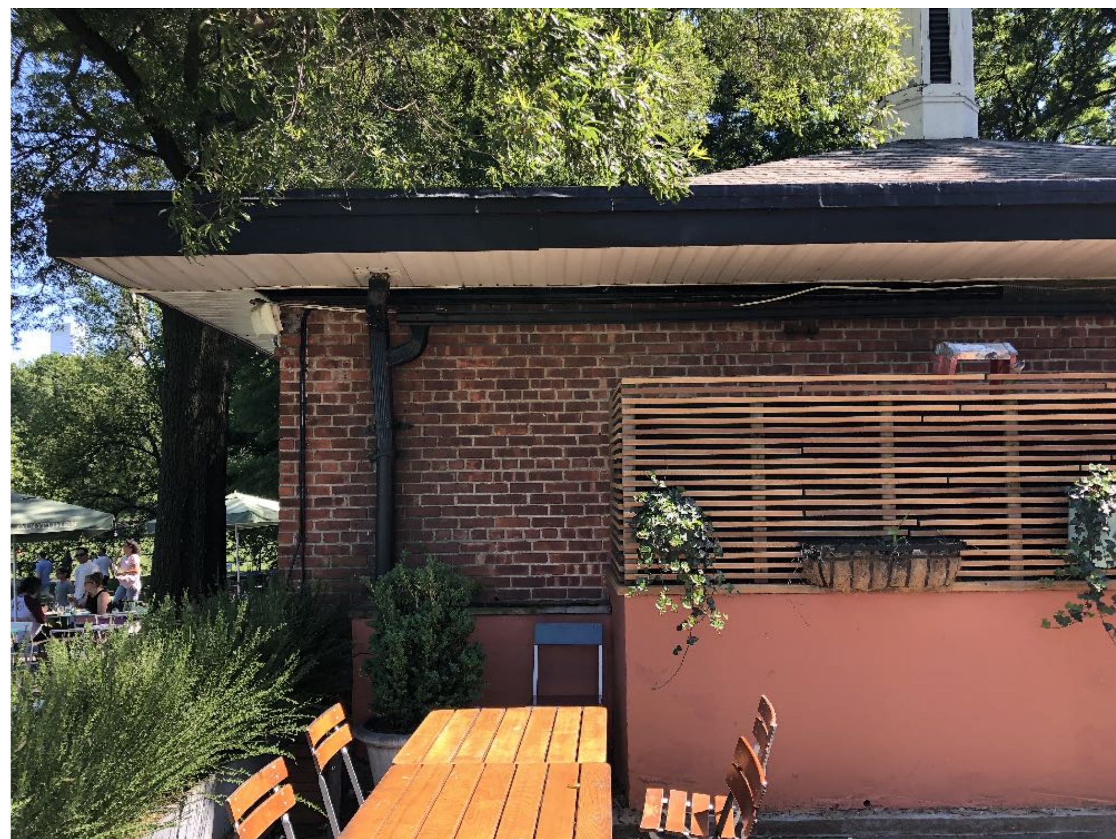
D EXISTING CONDITIONS PHOTO TRASH ALLEY
