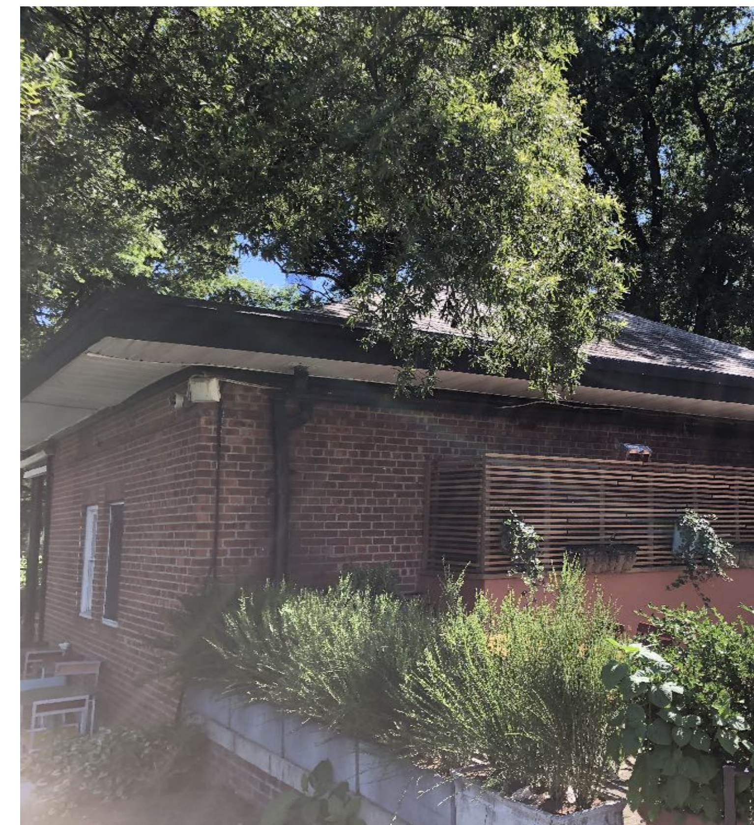
F EXISTING CONDITIONS PHOTO EXISTING RETAINING WALL
