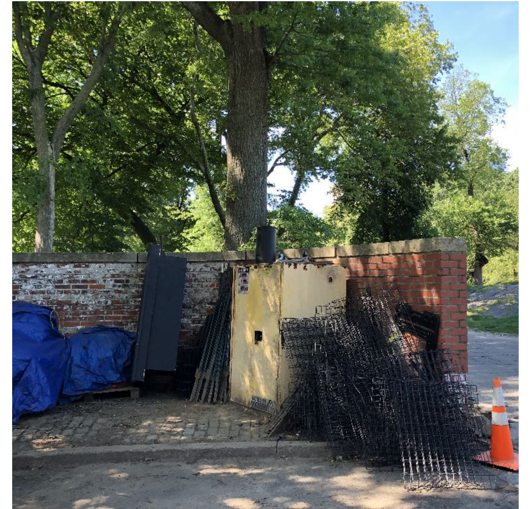
C EXISTING CONDITIONS PHOTO EXISTING BRICK WALL
