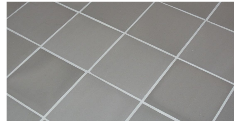
F QUARRY TILE (SERVICE AREA PAVING)
