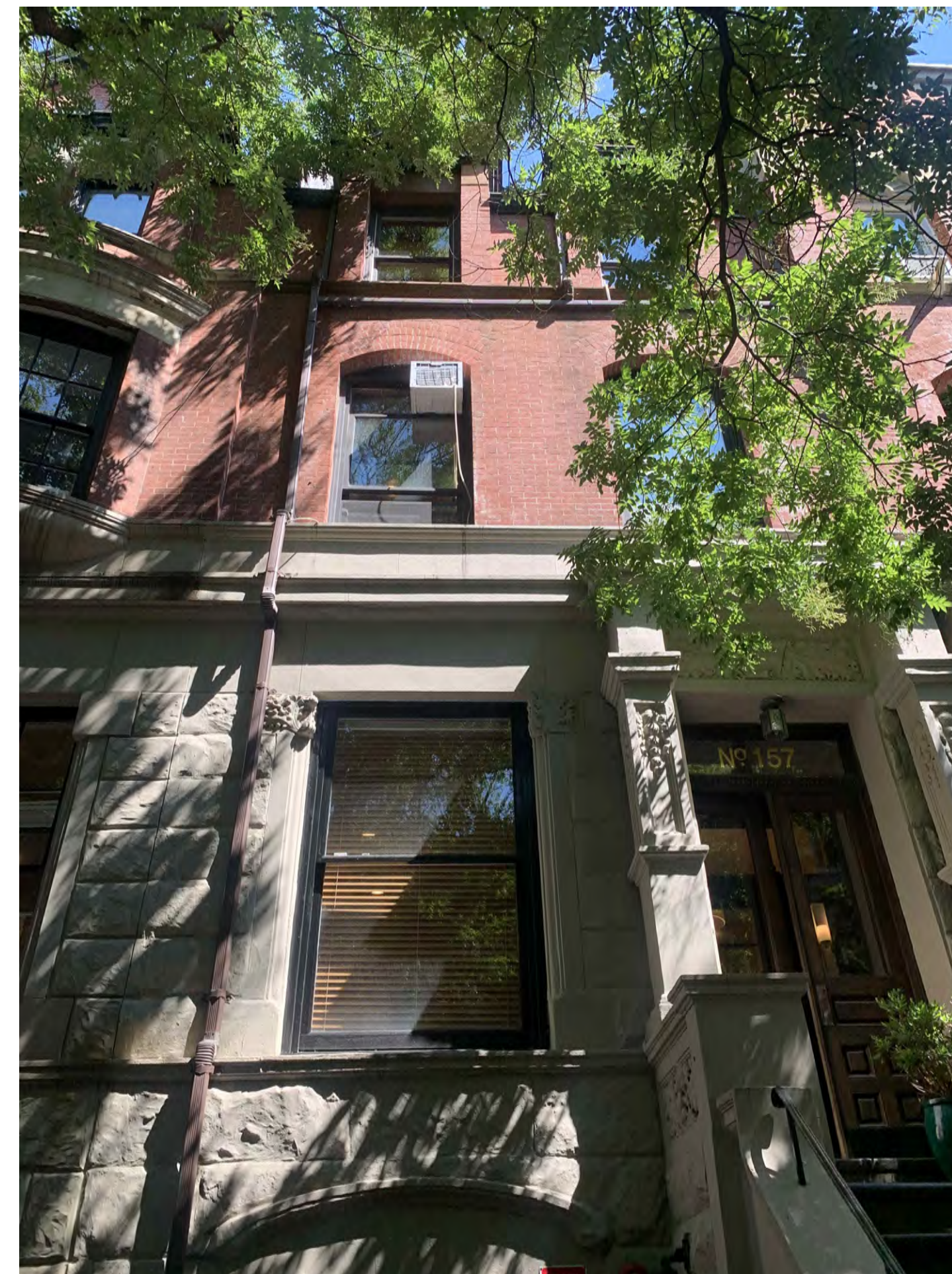
2 2023 EXISTING CONDITIONS PHOTO SCALE: 1/4" = 1'-0"
