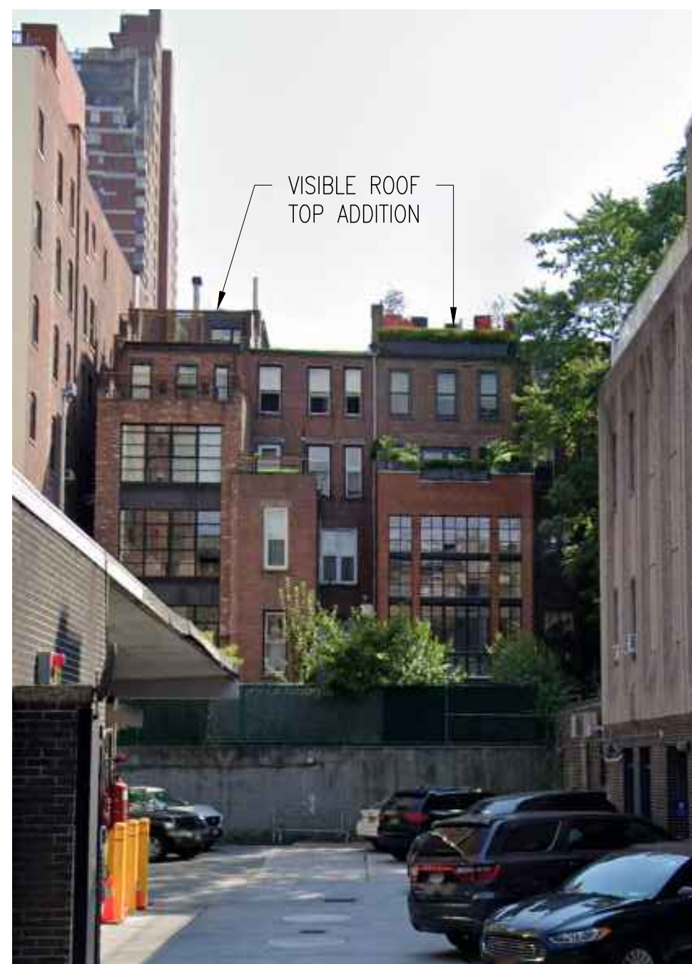
117 & 121 WEST 81st STREET (VISIBLE FROM REAR)
