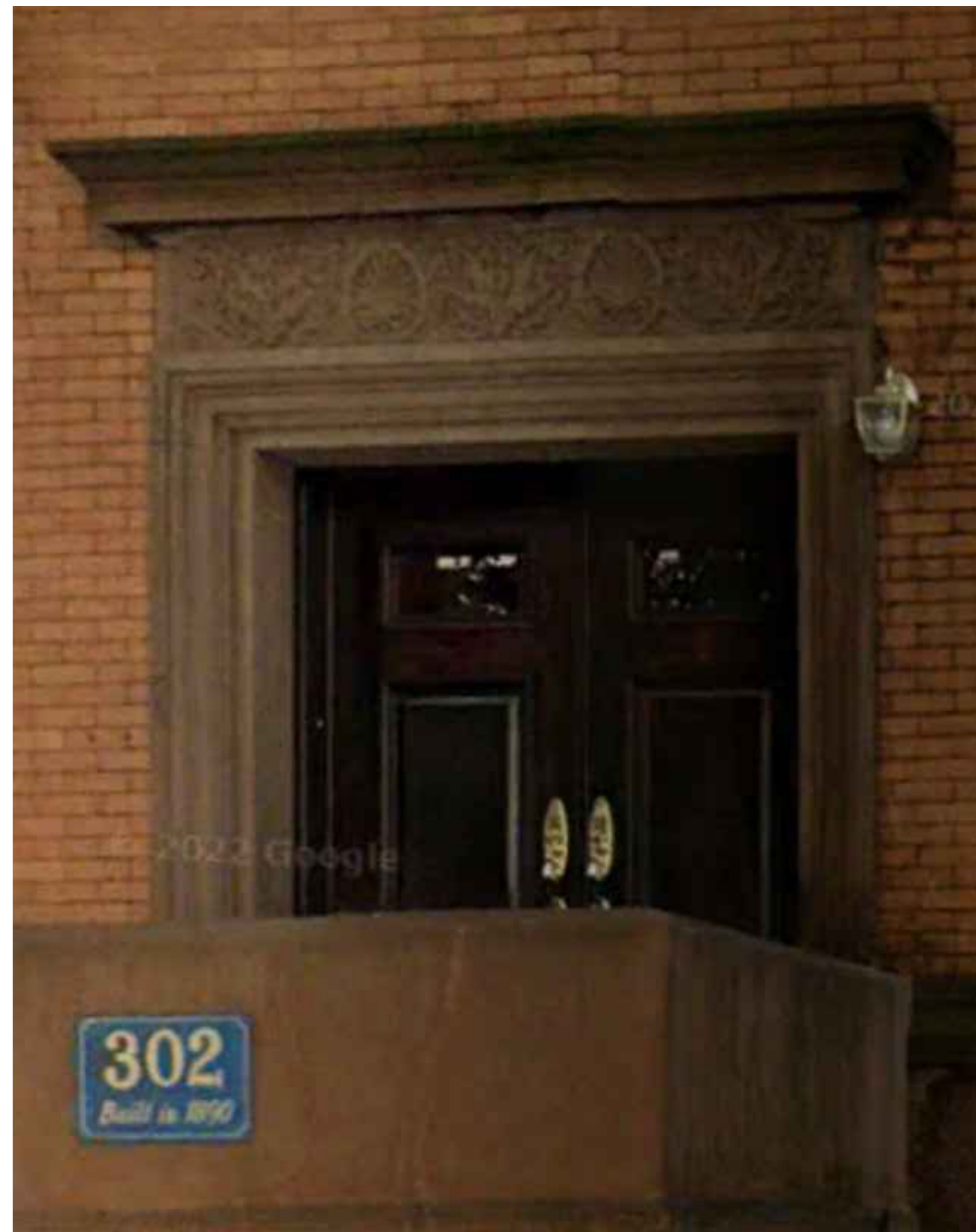
1- DOOR SURROUND @ 302 W 77TH STREET
