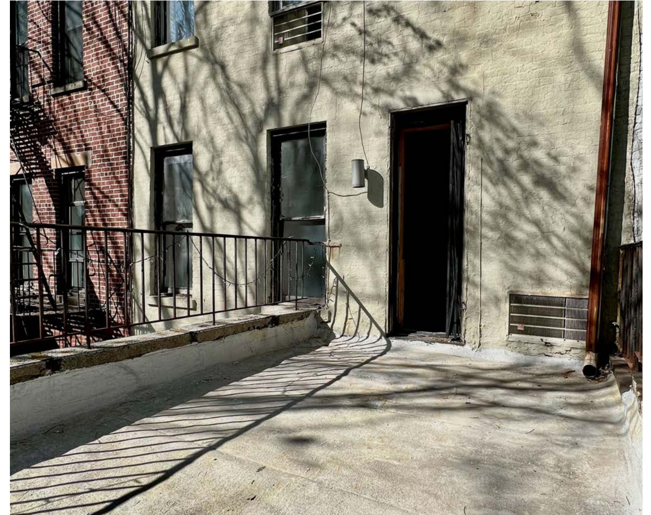
Door out to roof of existing ell
