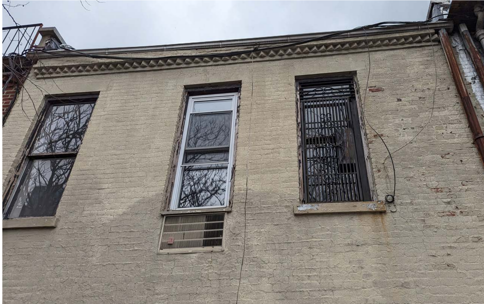
Top floor of rear elevation
