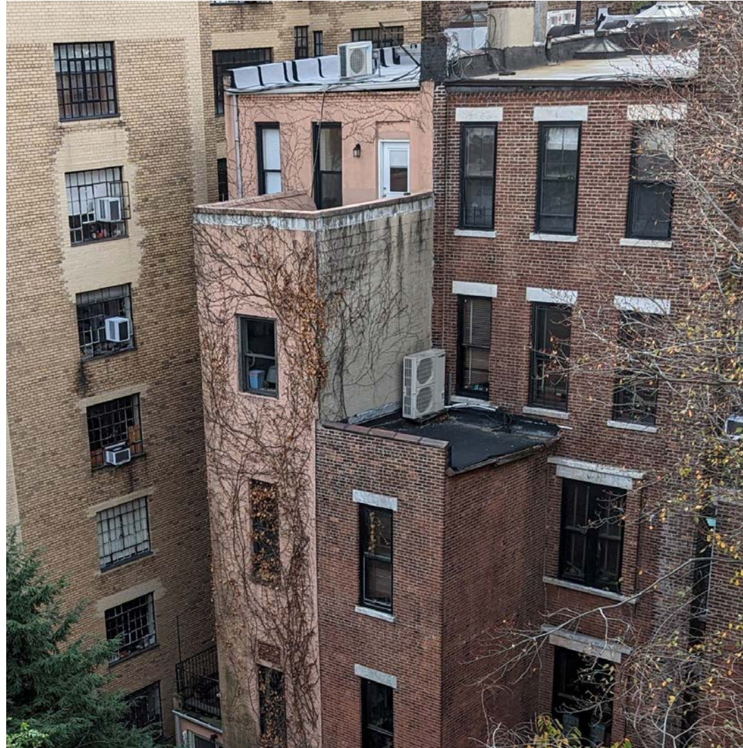
Ell enlargement at 41 West 90th Street
