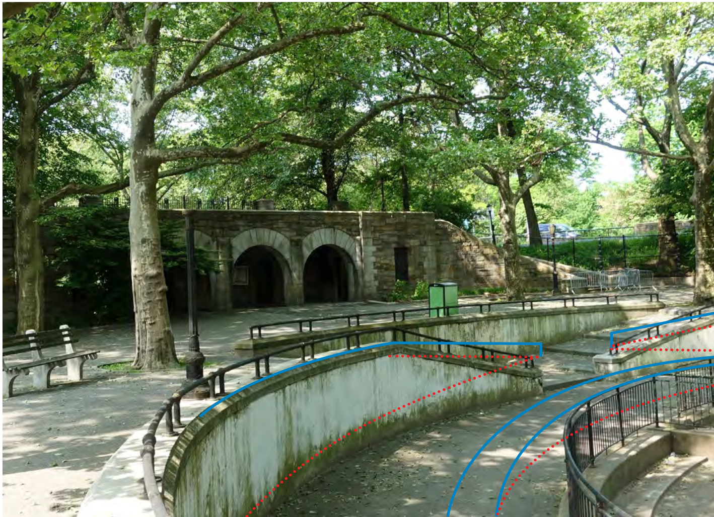
Existing Southern View
