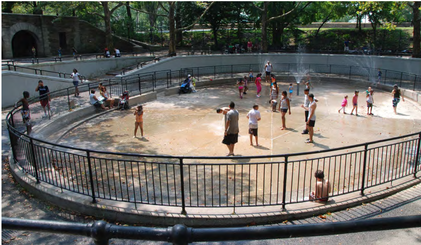
1 - Existing Water Play Area
