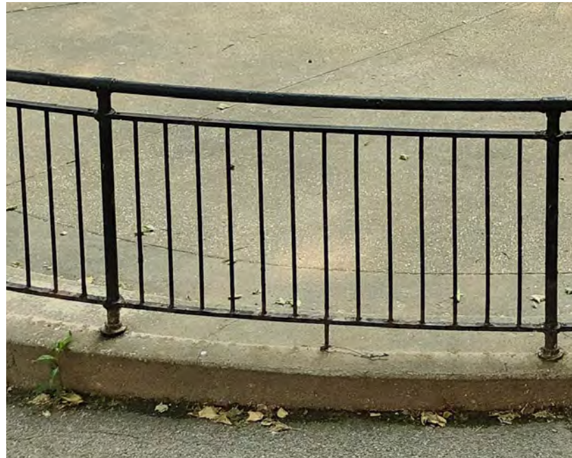
Existing 42" ht Fence on Wall at Water Play Area
