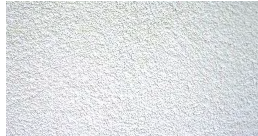
Sand Texture in a Medium Density Appearance, Painted White, For Inner Face of New and Parapet Wall
