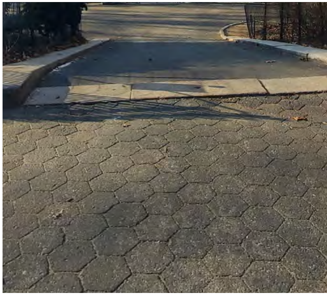
Asphalt Block Hex Pavers to match Existing at Riverside Drive
