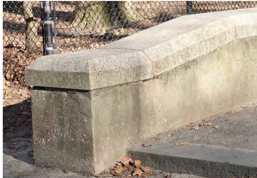
Replace-in-Kind Wall Coping as required
