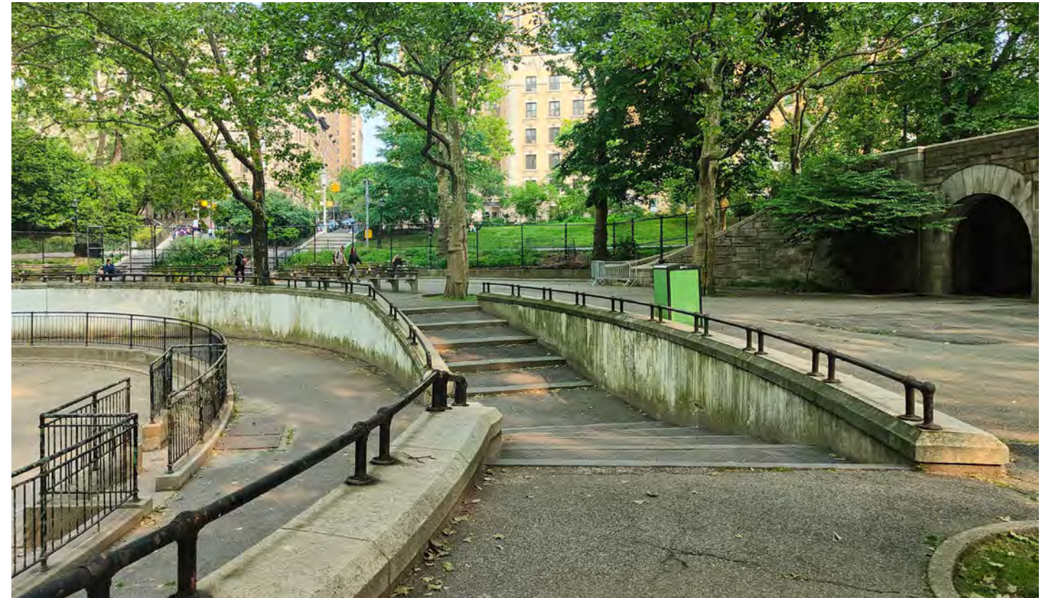
2 - View of Ramp Steps with Bluestone Treads, Granite Stone Coping and Railing
