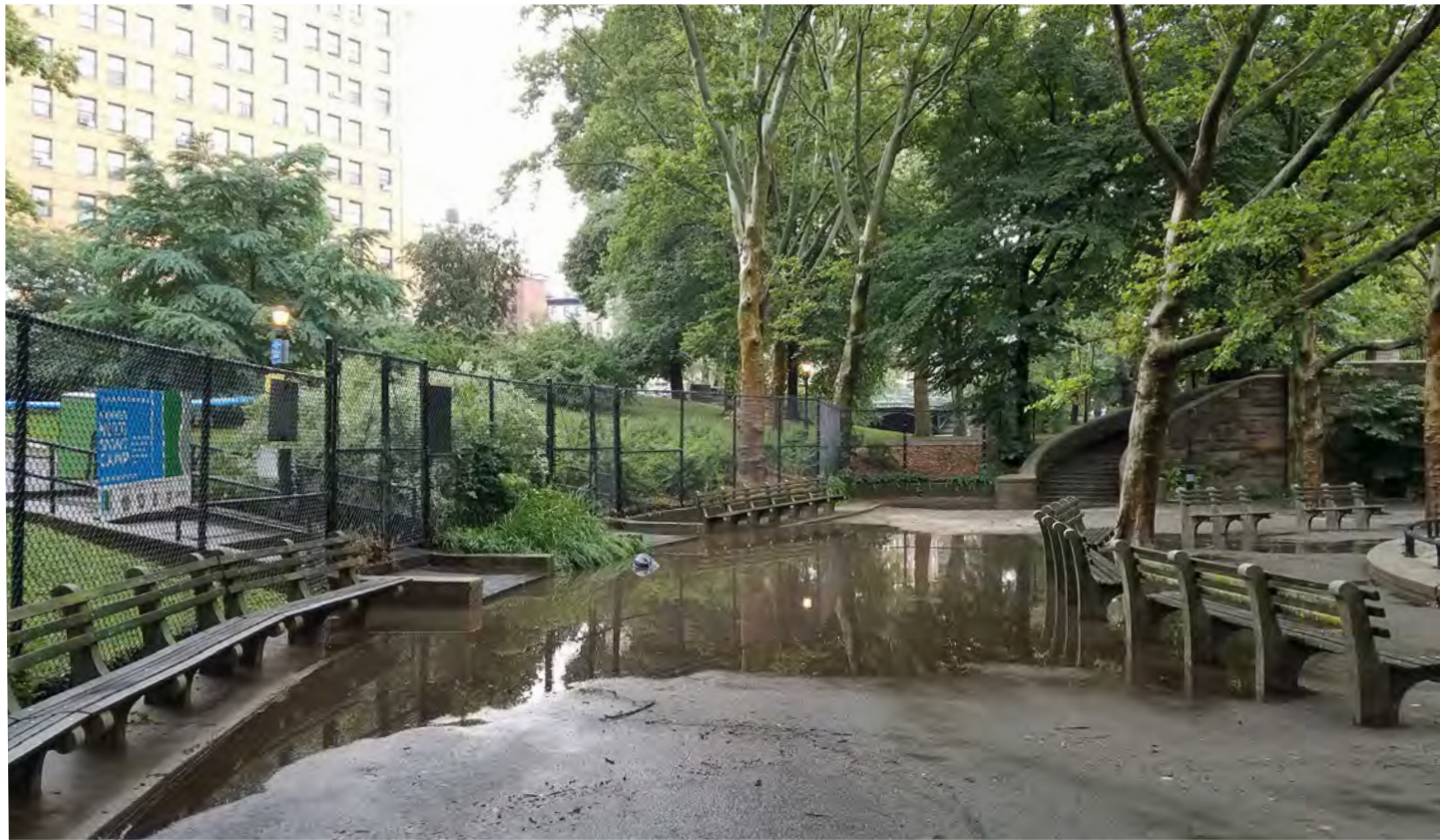
1 - Typical Flooding at Middle Terrace Entrance
