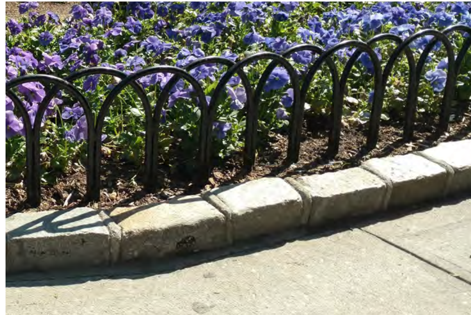
Wicket Steel Fence with Granite Block Edging, 12in high with 2in reveal
