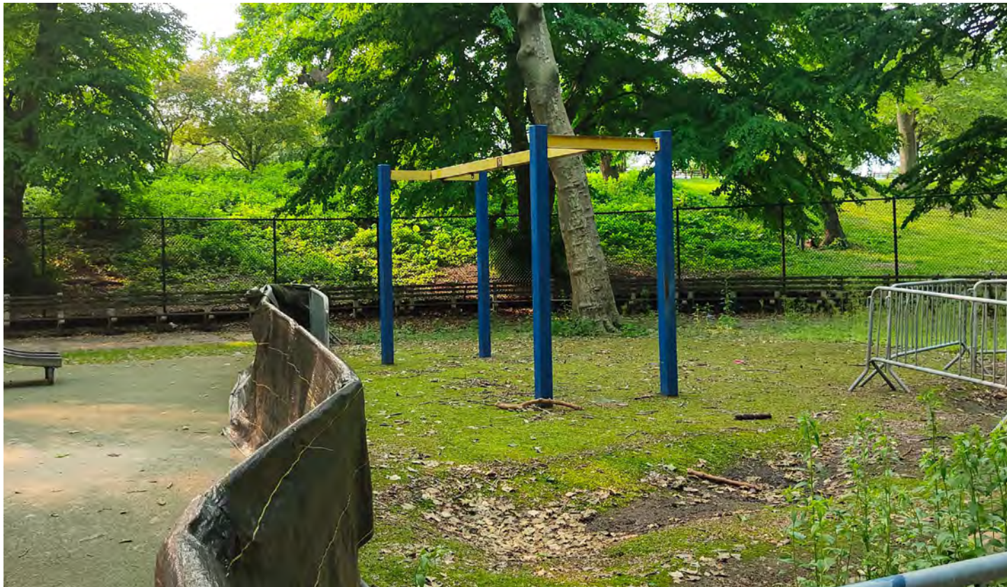
1 - Existing defunct gymnastic hoops in the area of sinkhole Area Currently Closed
