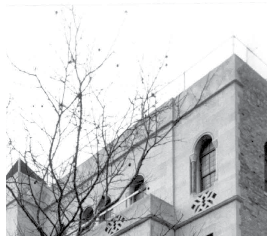
Enlargement of Designation Photo Showing Existing Fence
