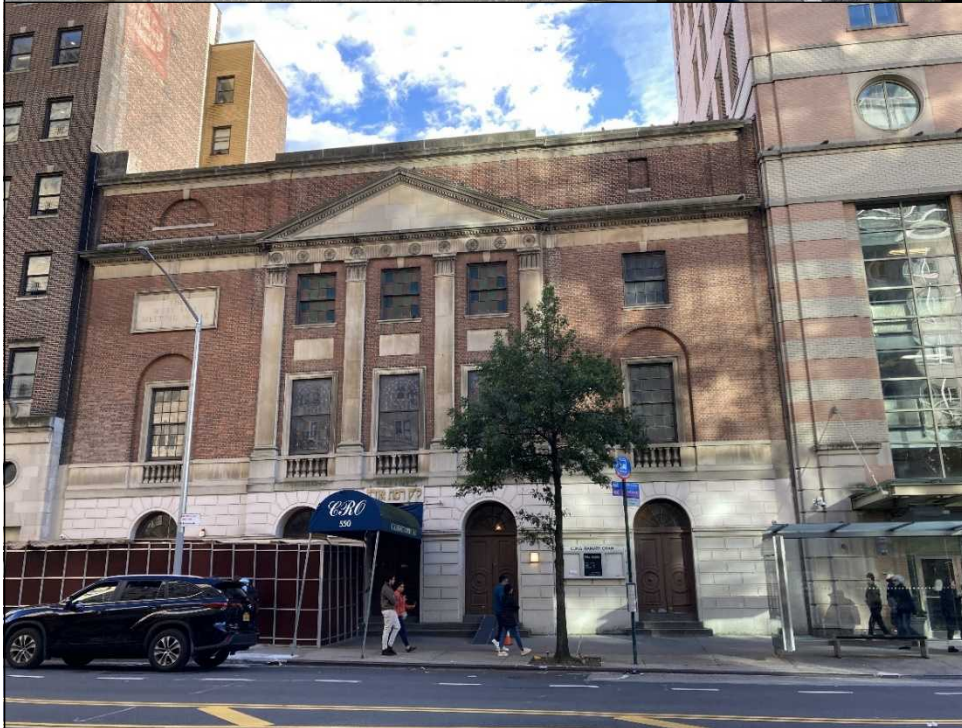
24. View southwest toward the Project Site (not visible) overlooking the West Side Unitarian Church - Congregation Ramath Orah (15NR00056)
