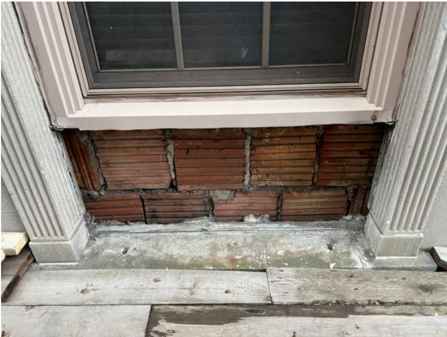
Probe/removals at existing spandrel panel
