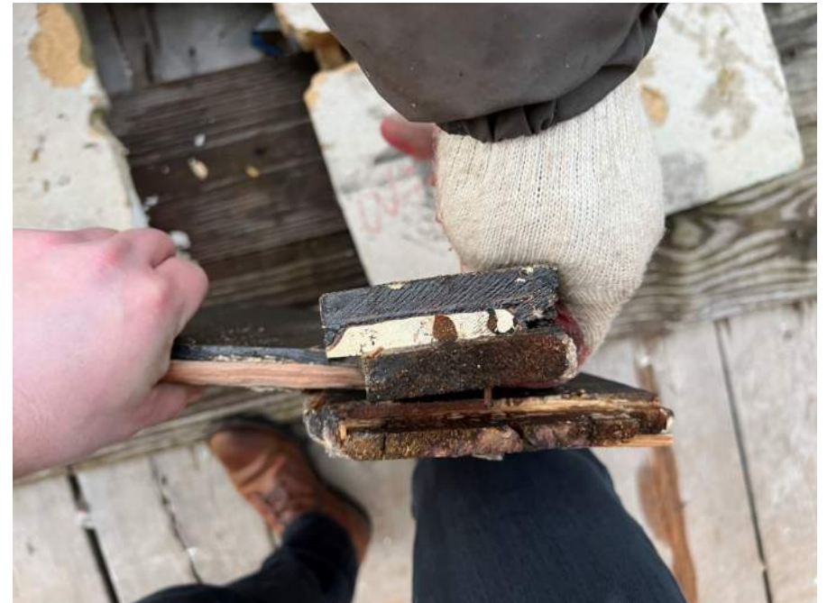
Probe/removals at existing spandrel panel
