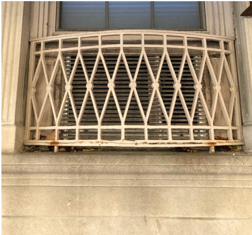
Existing modified spandrel panel – note the louver stops roughly 6" short of the jamb at either side, leaving remnants of the original spandrel panels
