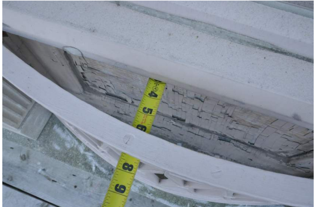
Existing spandrel panel – paint failure
