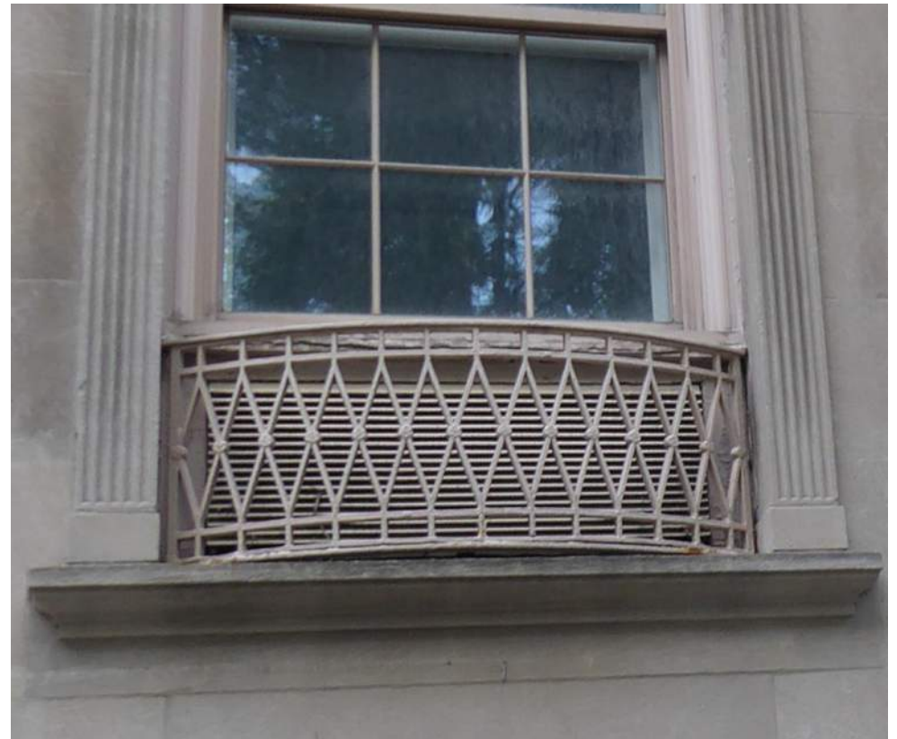
Existing modified spandrel panel – note louver encompasses nearly the entire width of the opening; this is the general intent for future louver installations
