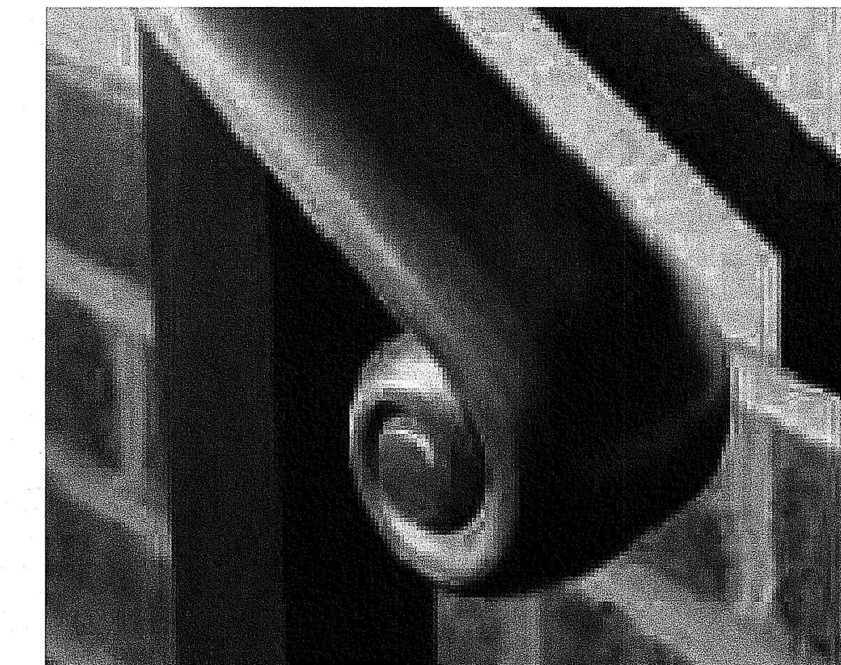
C2 PROPOSED HANDRAIL END FITTING A-420 N.T.S.
