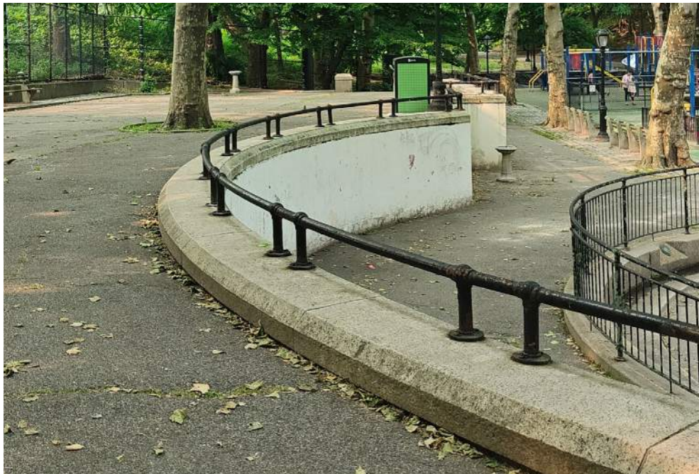
Raise Existing 12” ht Pipe Railing on Existing 12” ht Parapet wall to compliant height
