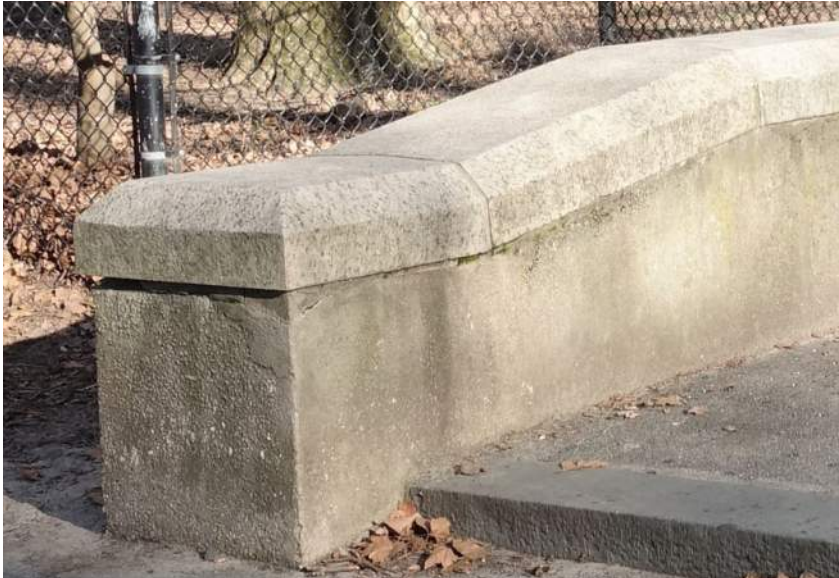
Replace-in-Kind Wall Coping as required
