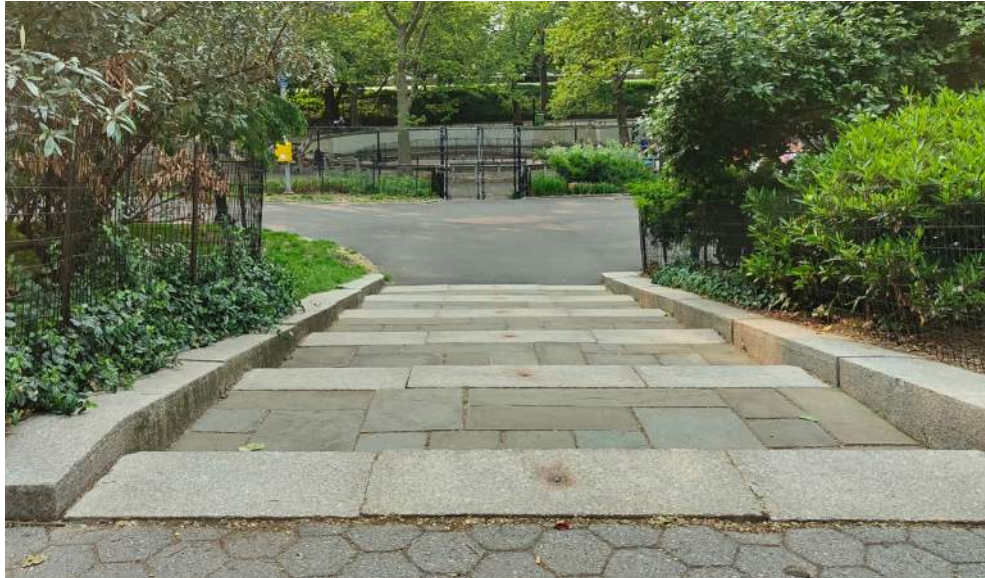
Replace Granite Curb, Bluestone Paver Landings and Granite Stair Treads at Riverside Dr Entry
