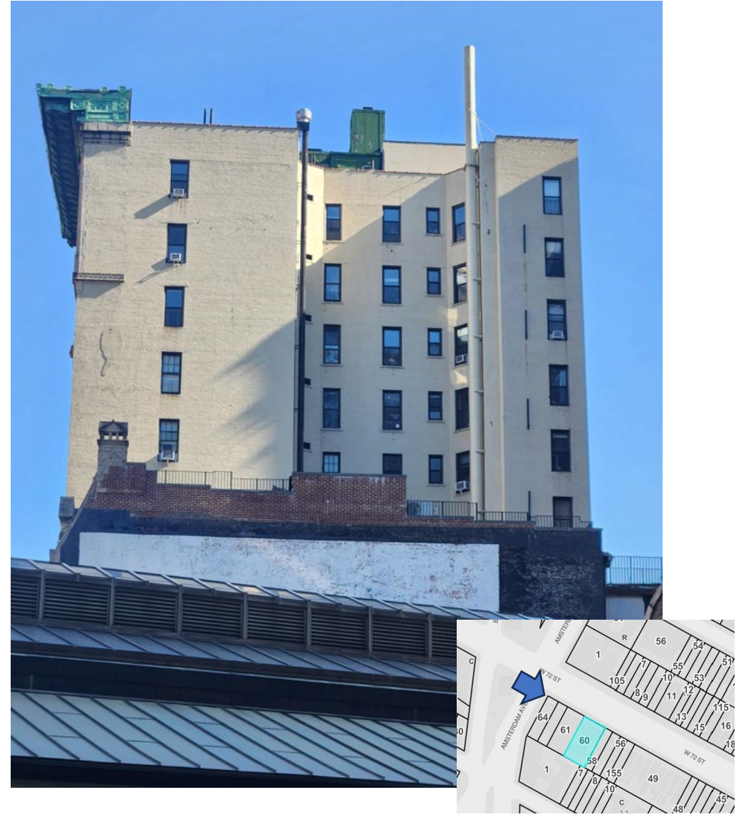
Proposed View of West Facade via Broadway - 2024
