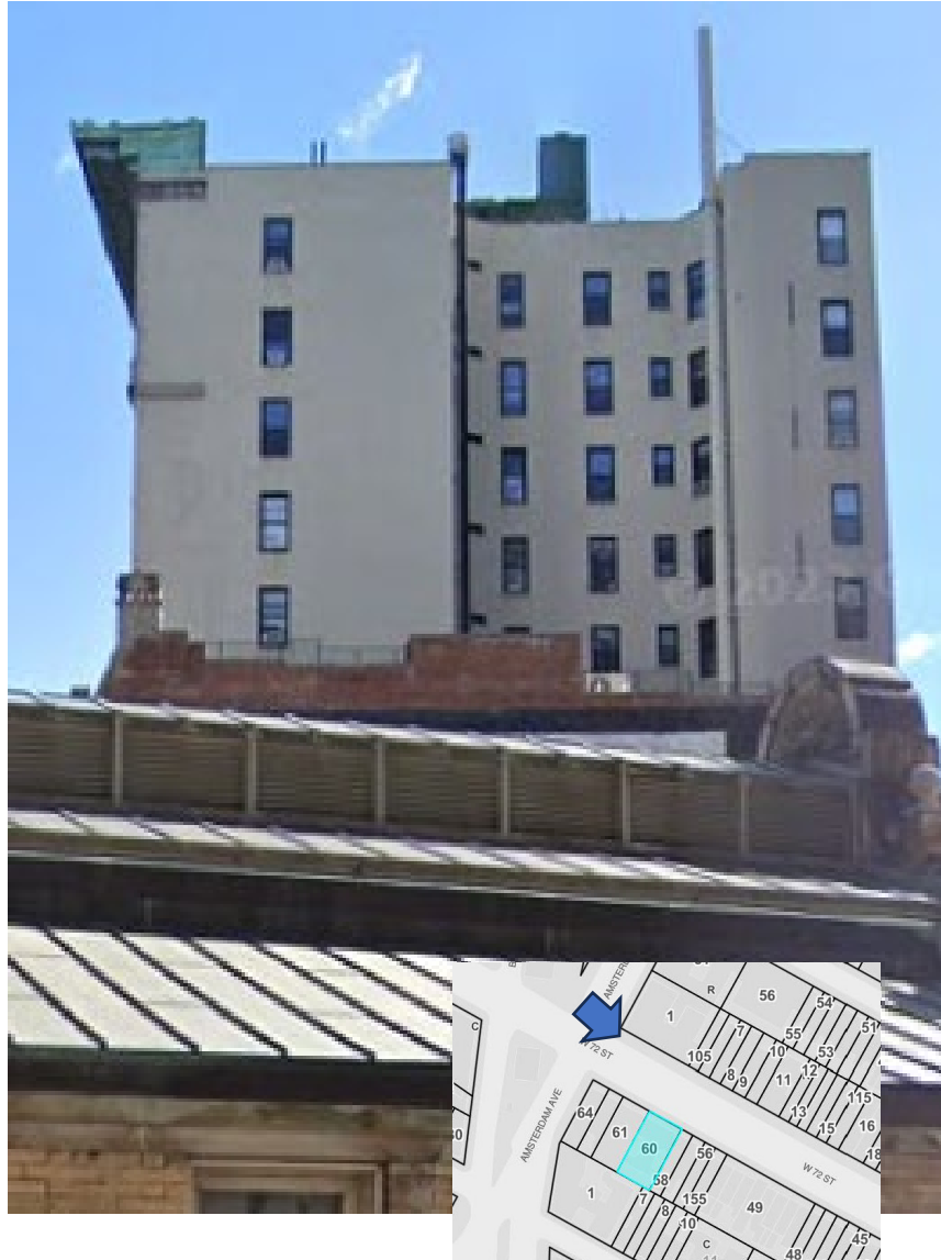
Previous View of West Facade via Broadway - 2022
