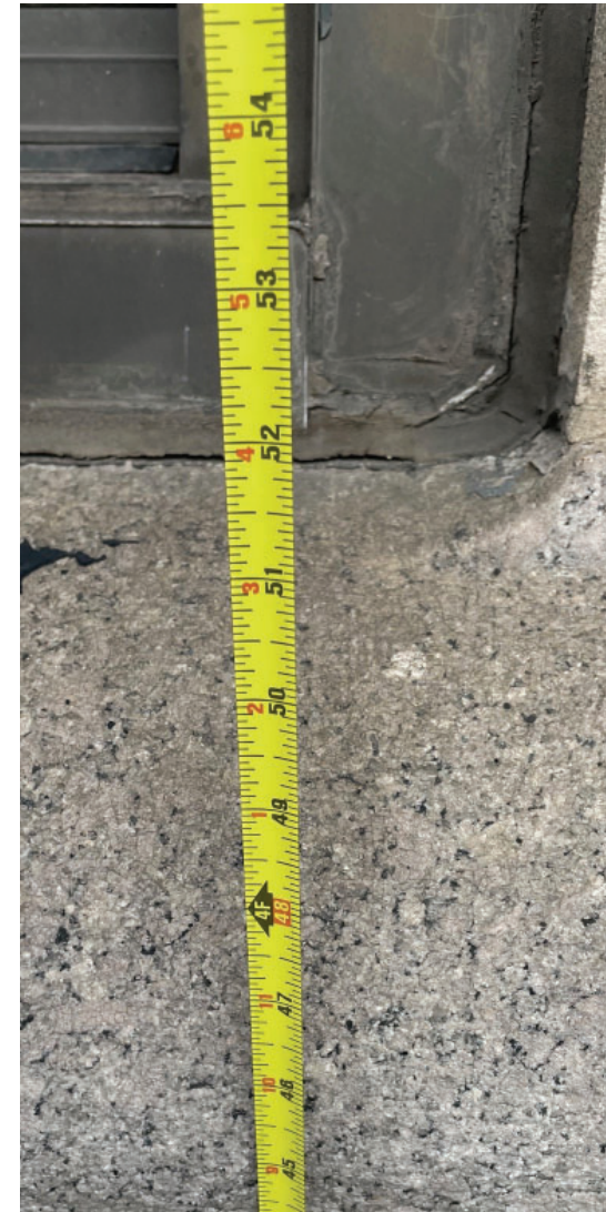
SILL HEIGHT EXISTING TO REMAIN 4'-4" ABOVE GRADE
