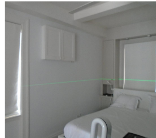
Existing Window Condition - Interior View ㉕
