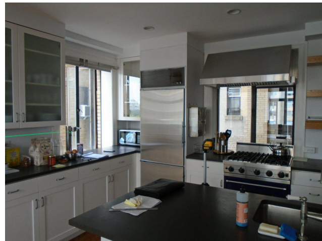
Existing Window Condition - Interior View ㉒ ㉓
