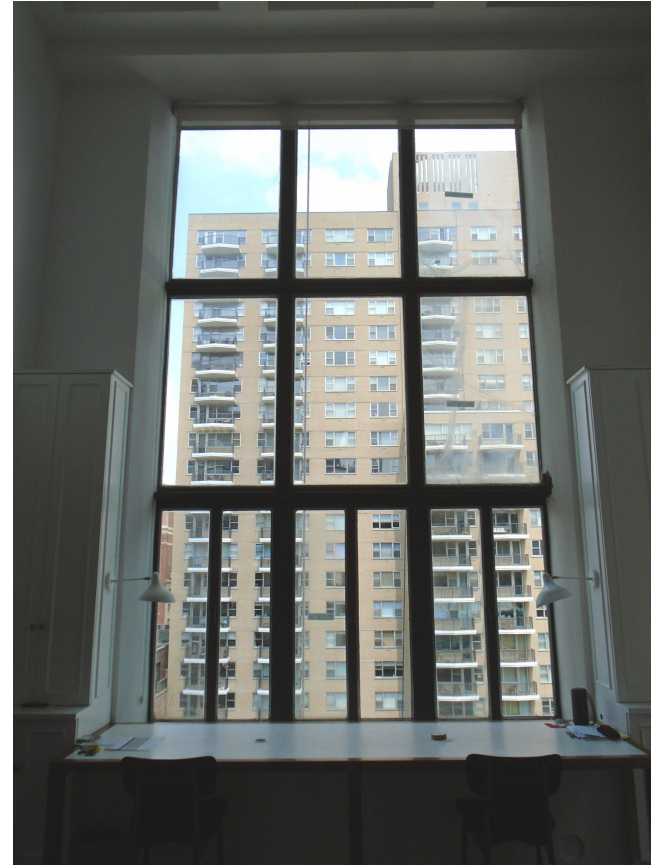
Existing Window Condition - Interior View ⑩ — ⑱
