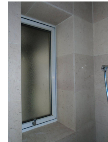
Existing Window Condition - Interior View ㉗
