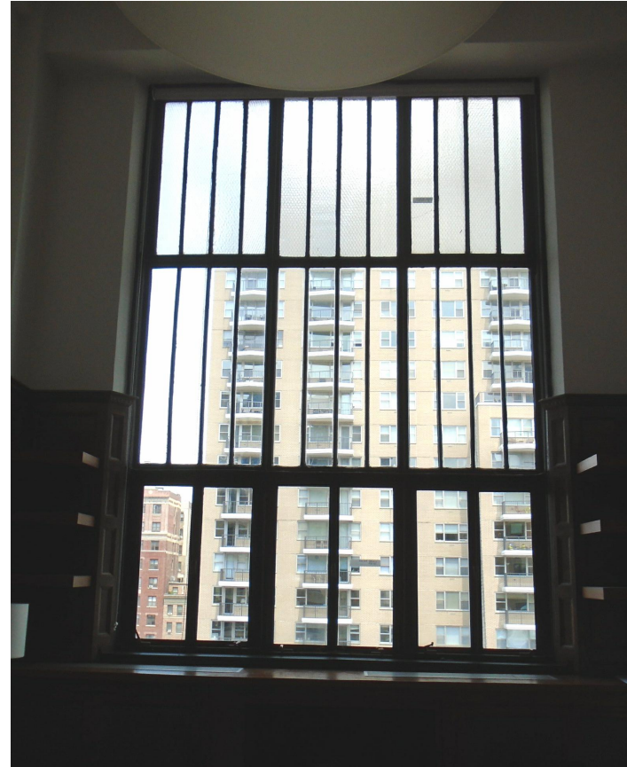
Existing Window Condition - Interior View ① — ⑨
