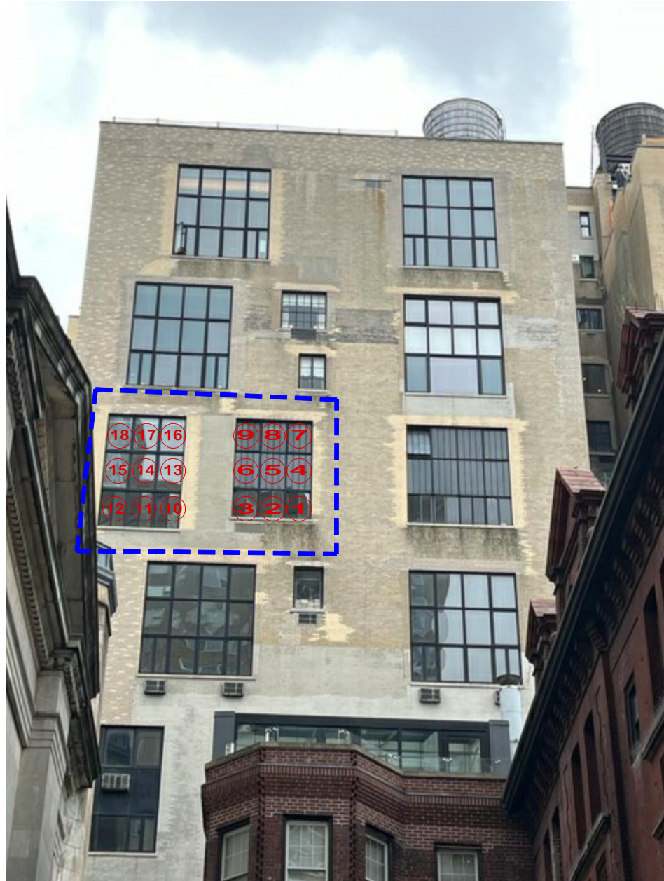
1 West 67th Street - Partial North Facade (Looking South from 68th Street)
