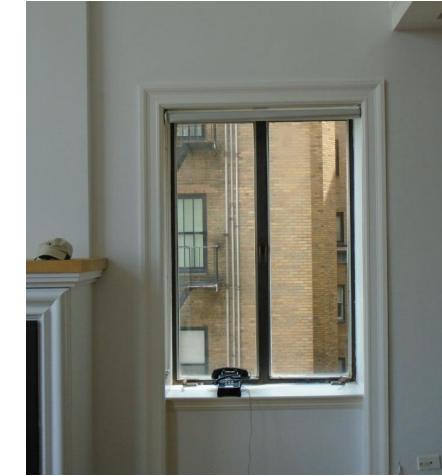
Existing Window Condition - Interior View ⑳
