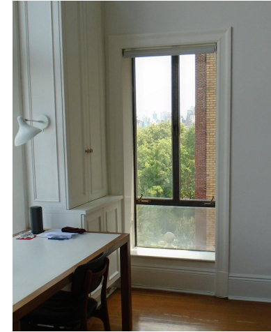
Existing Window Condition - Interior View ⑲
