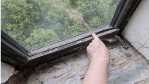
Photo 8: The gasketing and glass stop at the window sash frame of window #6 was visibly loose and able to be removed by hand.
