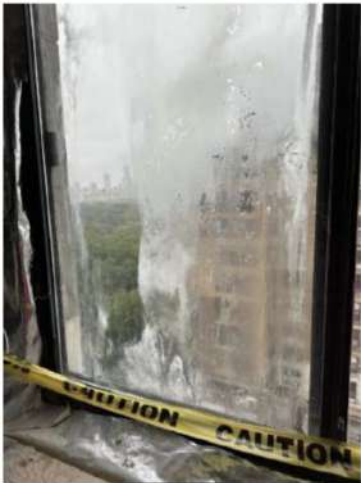
Photo 8: The gasketing and glass stop at the window sash frame of window #6 was visibly loose and able to be removed by hand.
