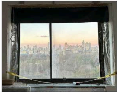
VIEW FROM INTERIOR WINDOW TYPE "A": EXIST. WINDOW PHOTO NTS 1
