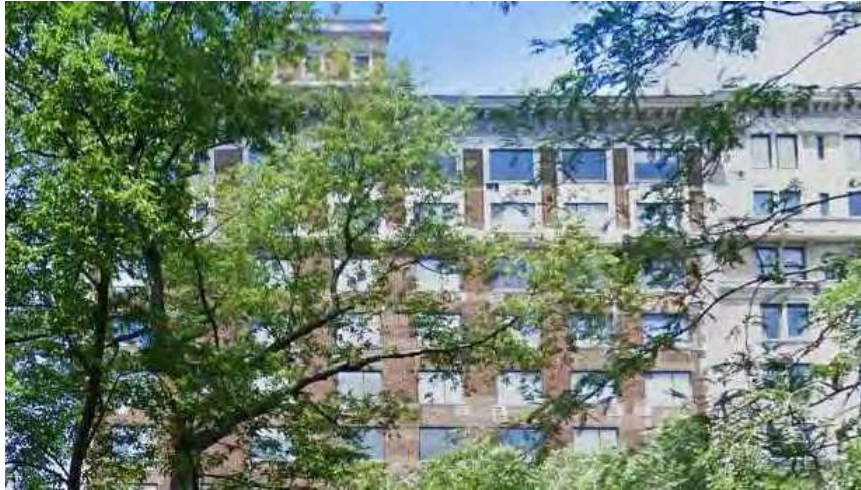
CPW Facade from Central Park
