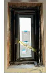
VIEW FROM INTERIOR WINDOW TYPE "D": EXIST. WINDOW PHOTO NTS 16
