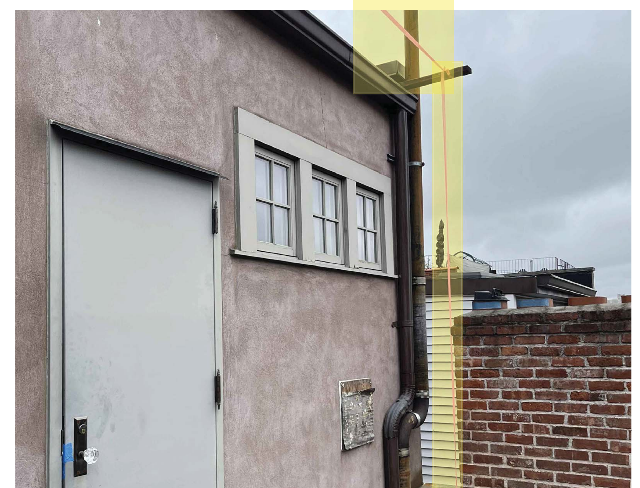
PENTHOUSE MOCKUP SOUTHWEST CORNER VIEW
