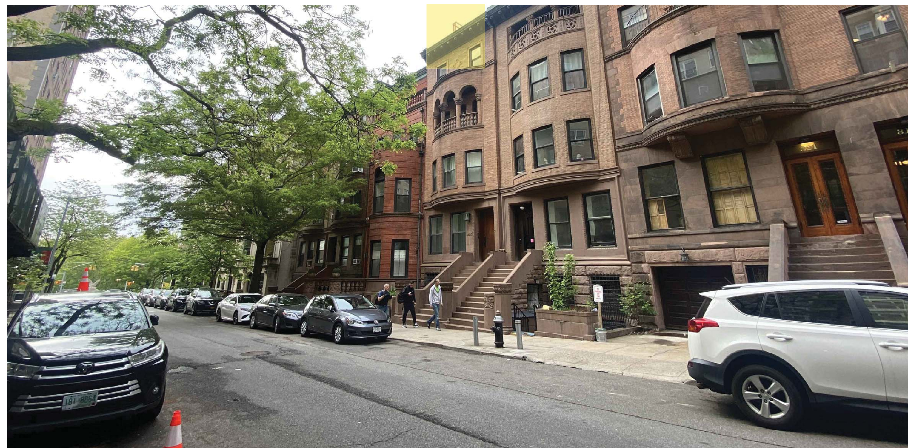
327 WEST 76TH STREET - LOOKING WEST
