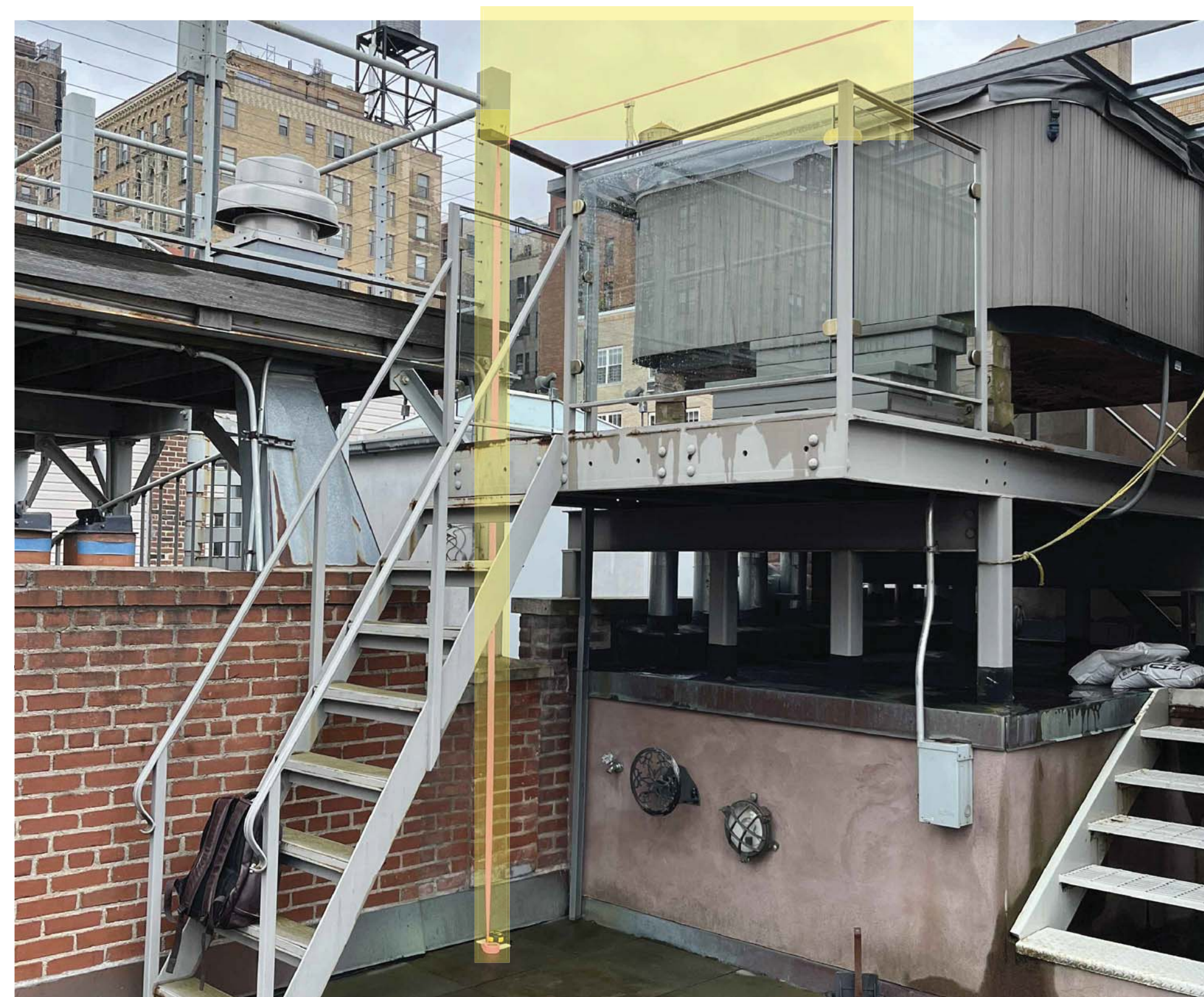
PENTHOUSE MOCKUP SOUTHEAST CORNER VIEW
