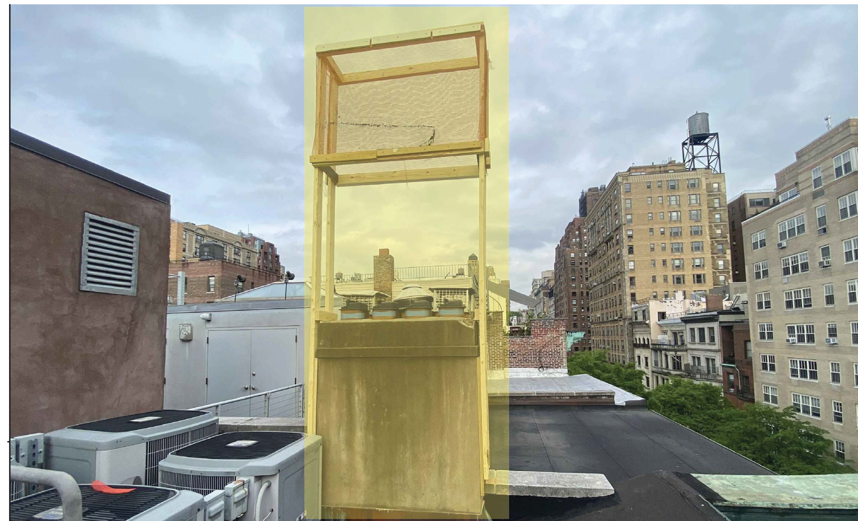
SOUTH PENTHOUSE LOOKING EAST
