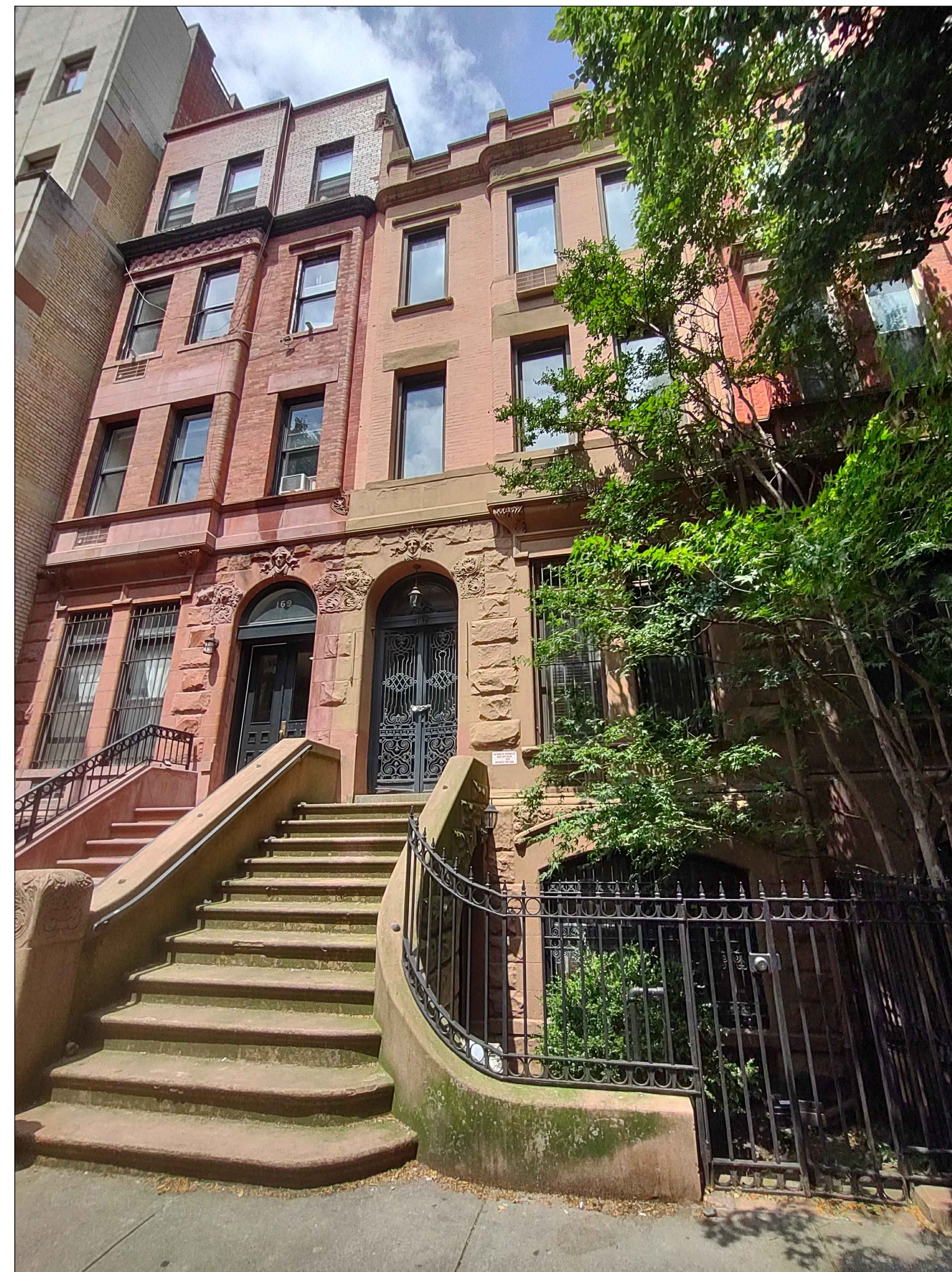
EXISTING SOUTH FACADE
