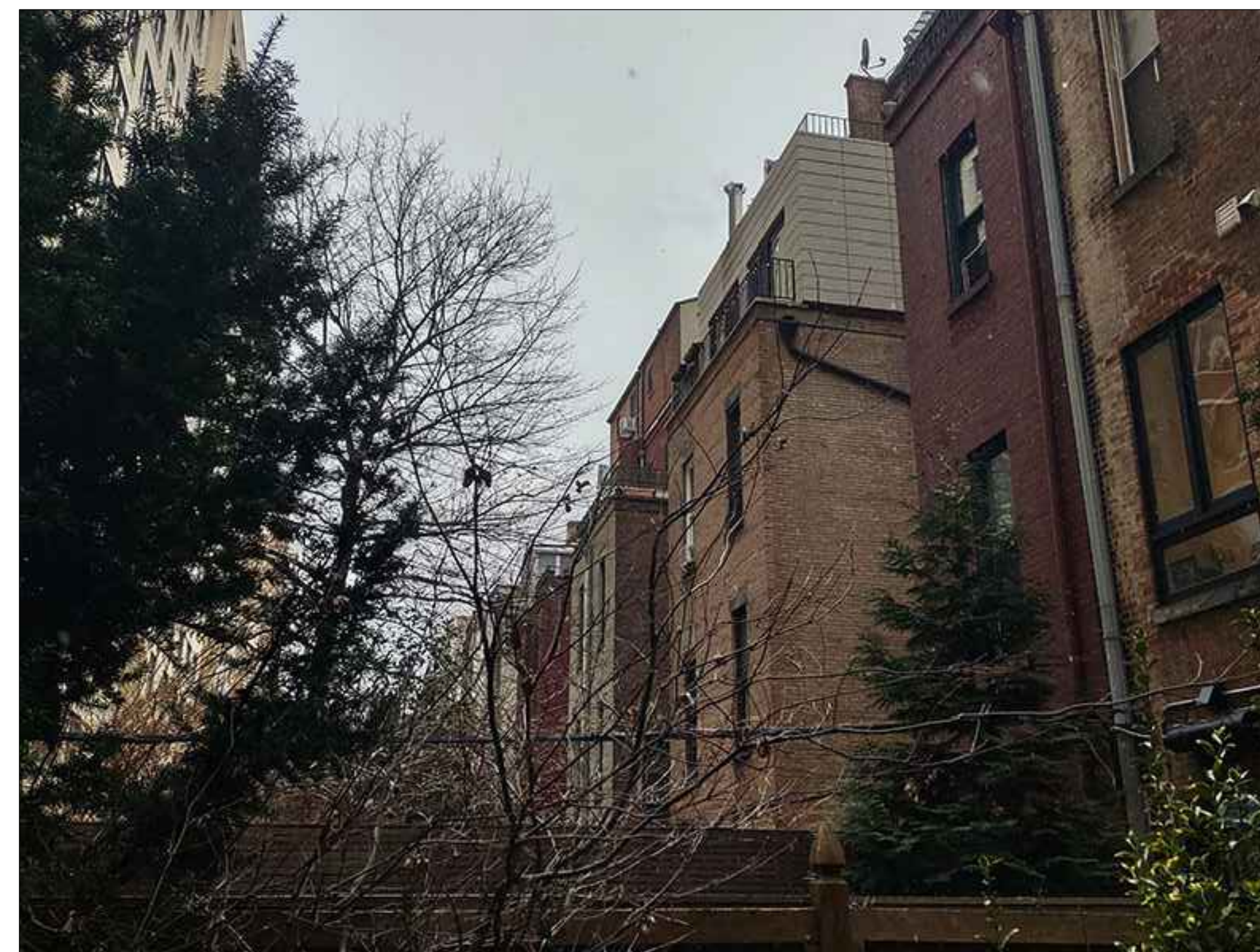
INTERIOR LOT CONDITIONS LOOKING EAST
