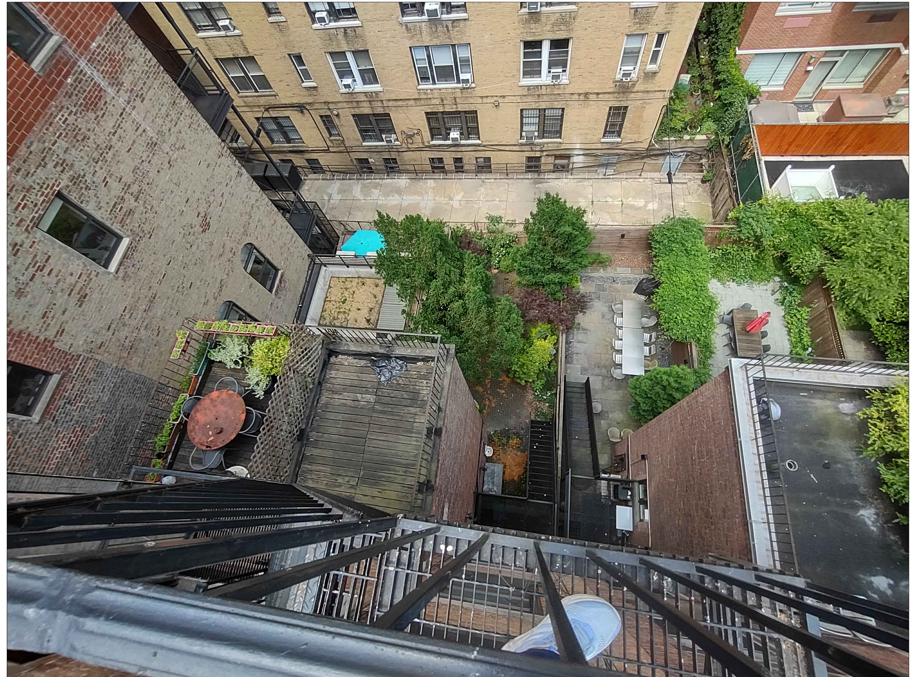
INTERIOR BLOCK CONDITION @ 165 & 167 W. 85TH ST
