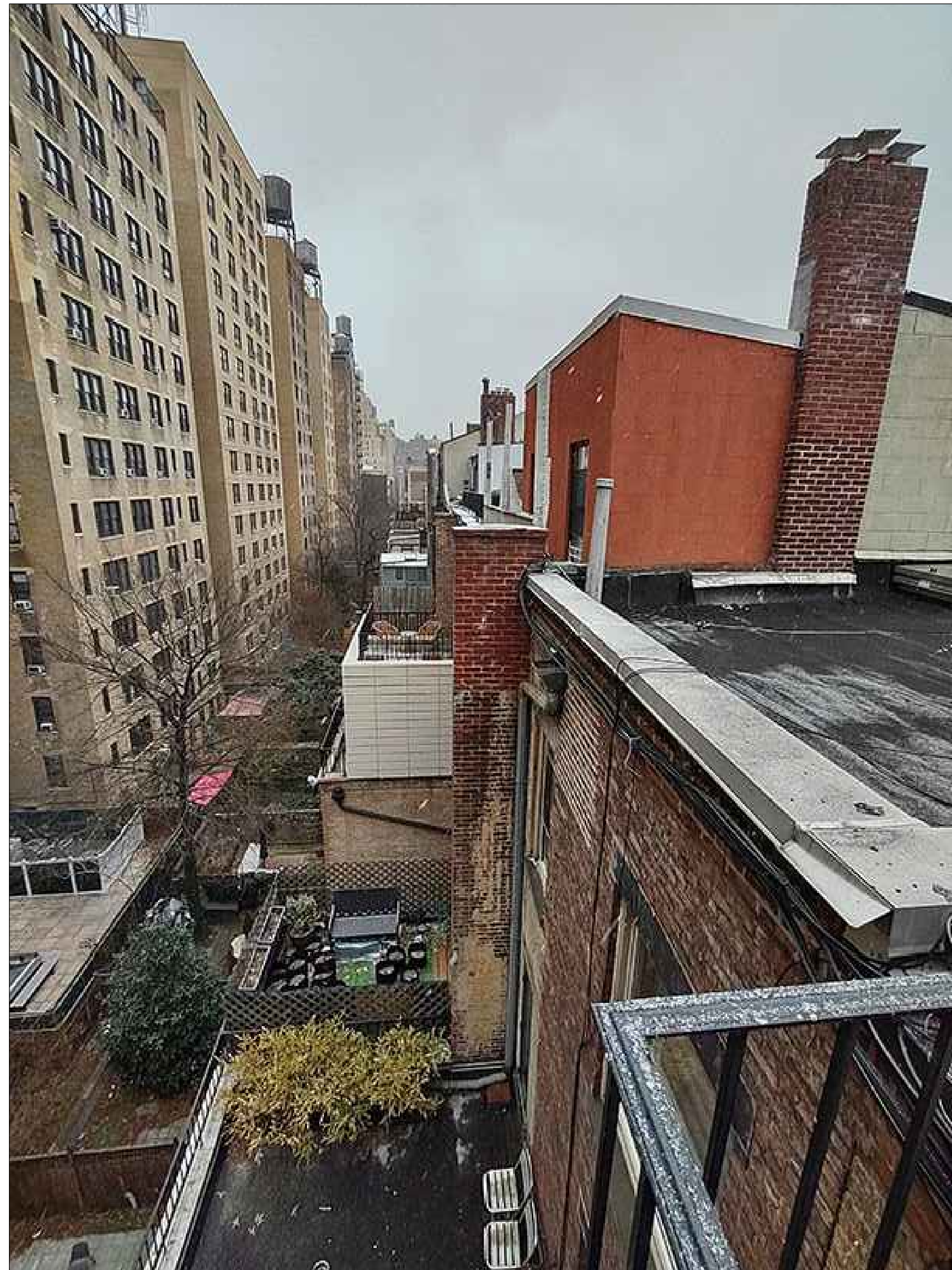
INTERIOR BLOCK CONDITIONS LOOKING EAST
