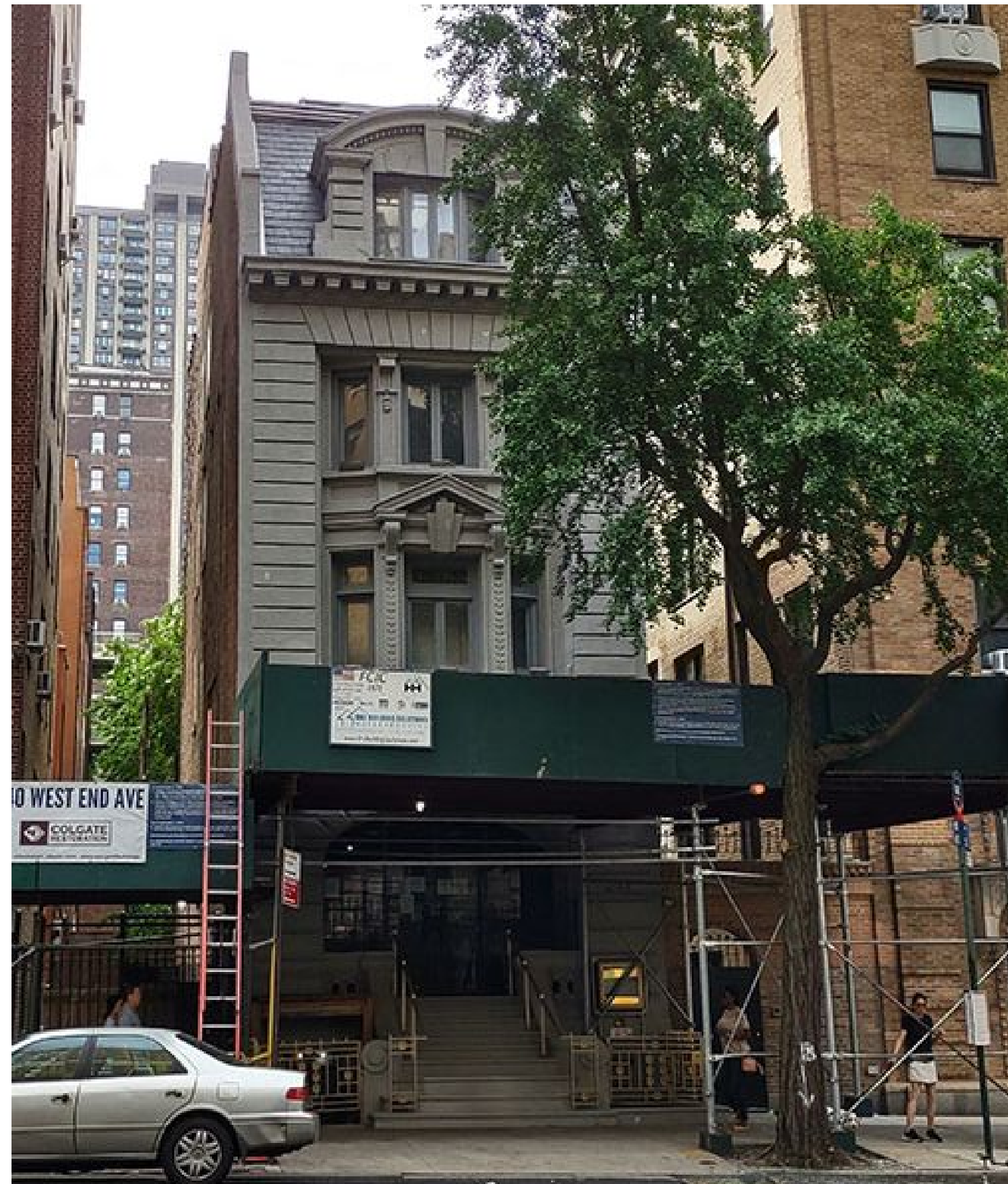
EXISTING FRONT FACADE
