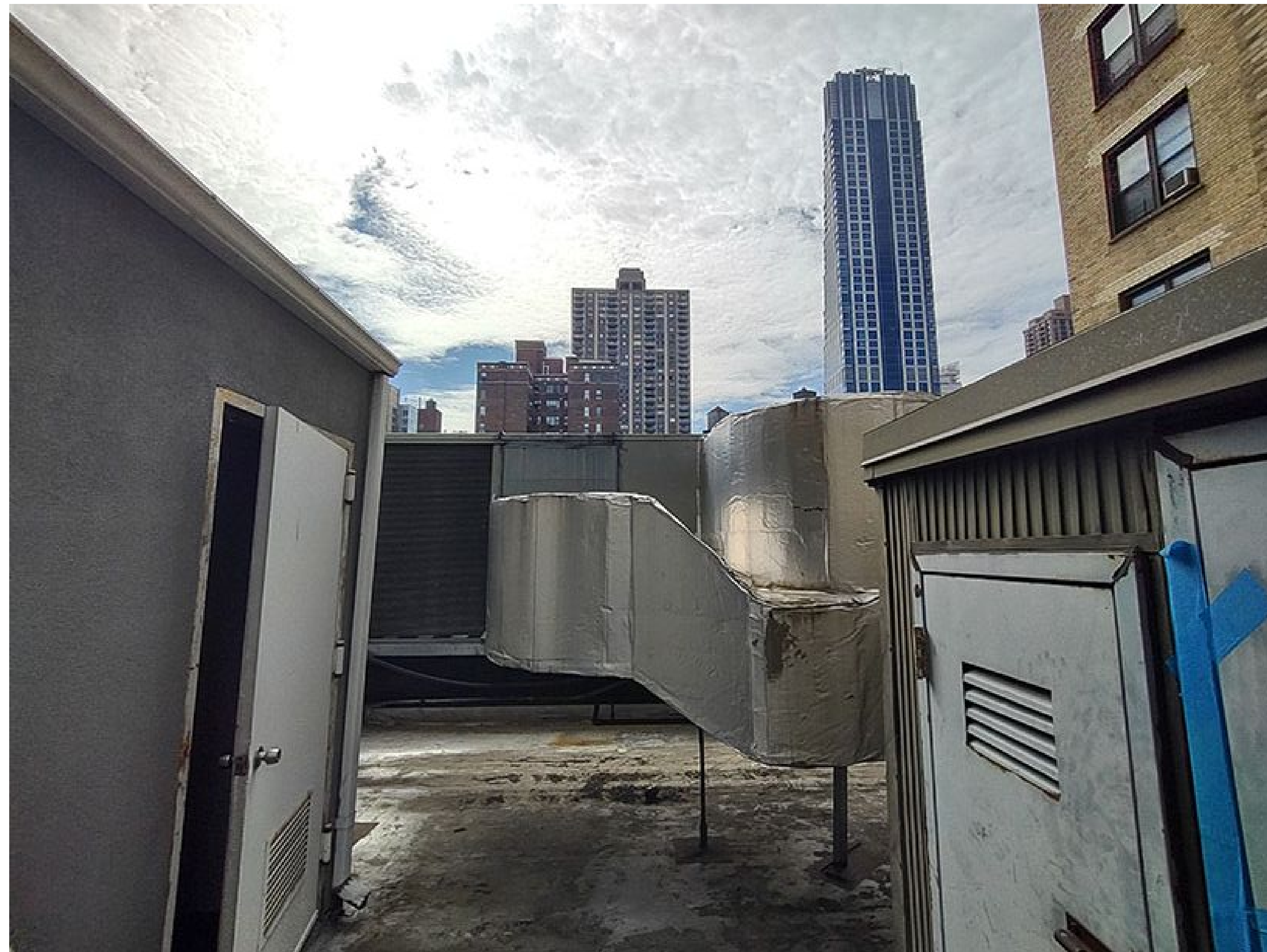
EXISTING CONDITIONS AT ROOF LOOKING WEST
