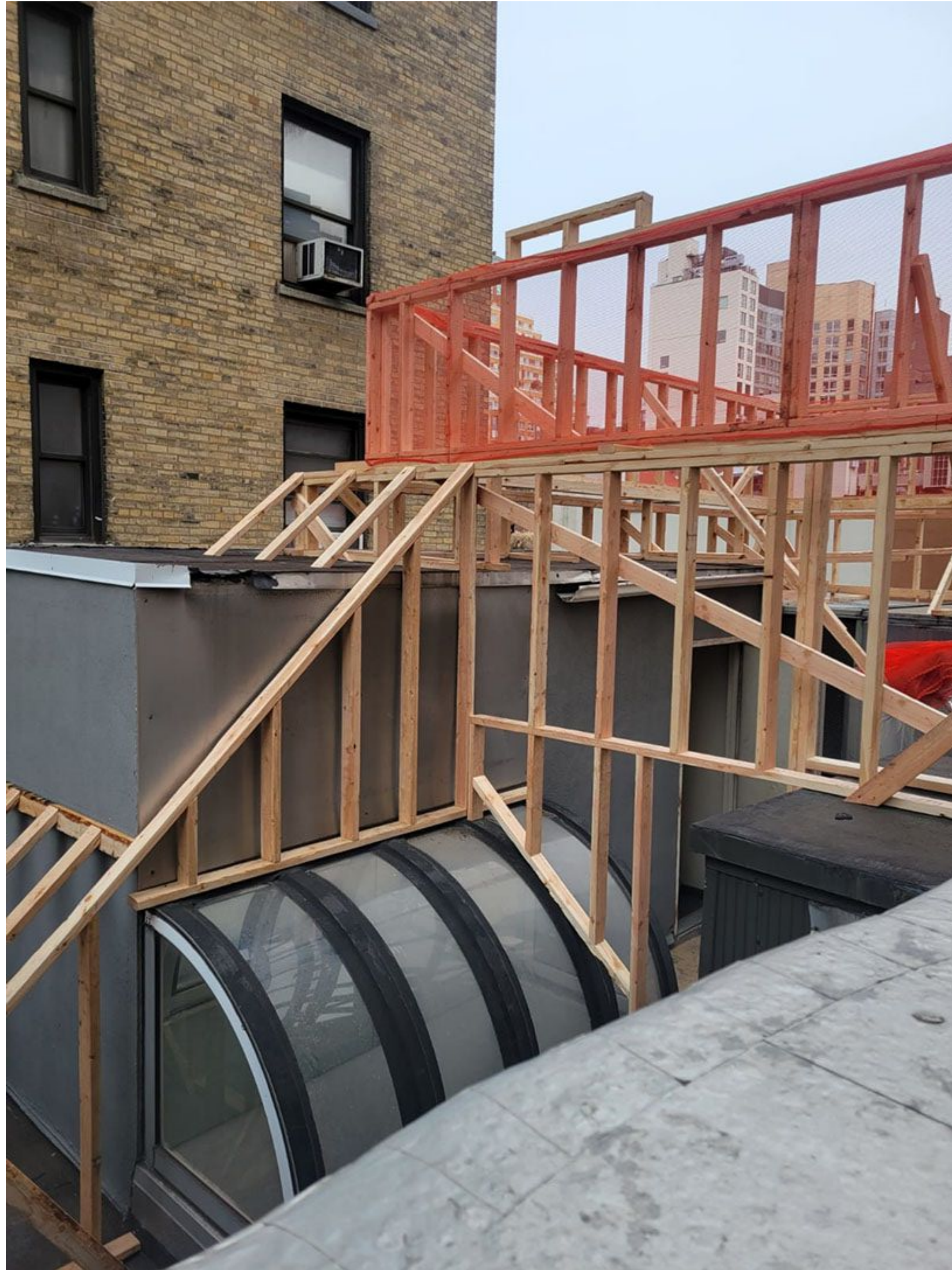
ROOFTOP MOCKUP LOOKING EAST
