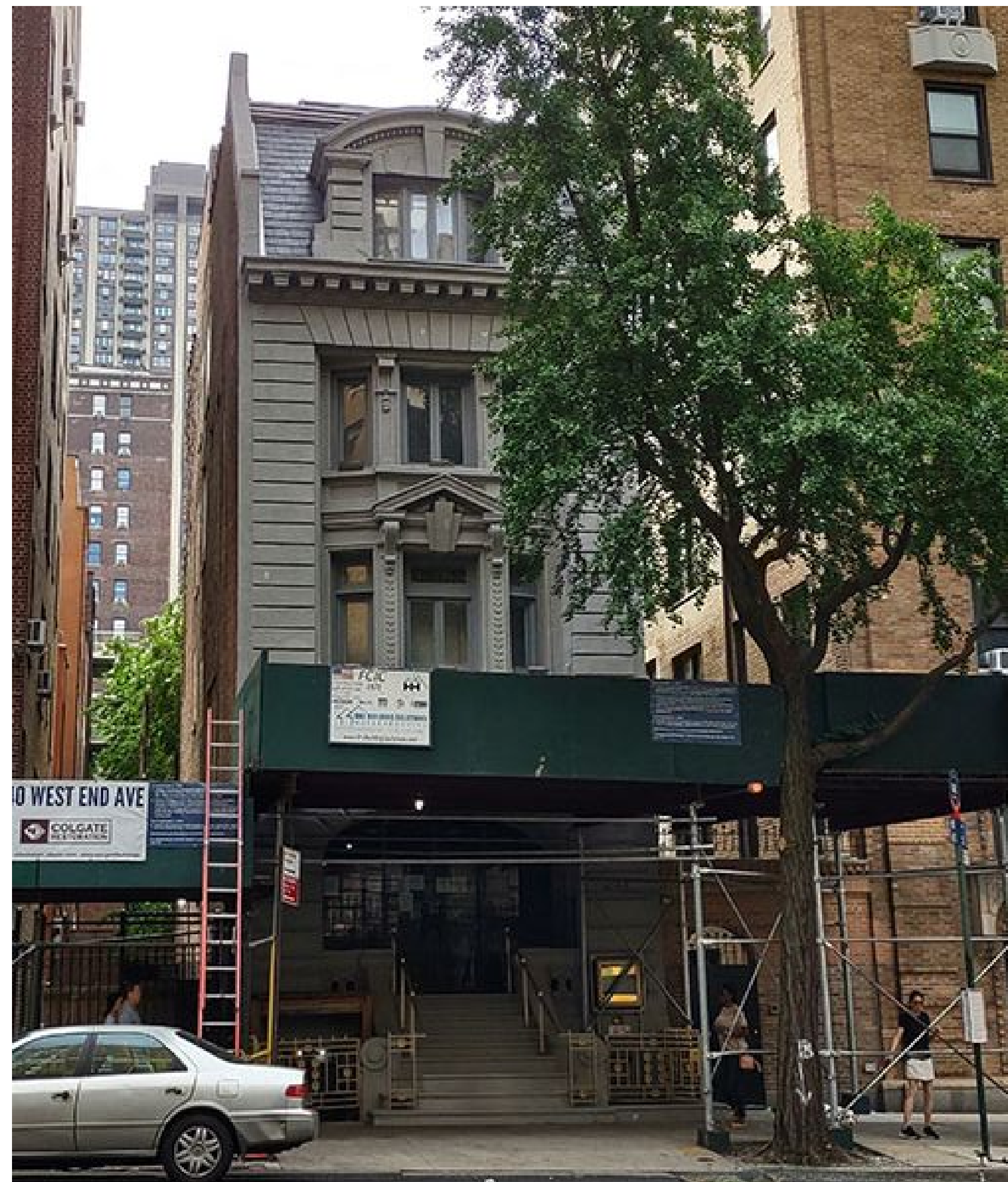
EXISTING FRONT FACADE
