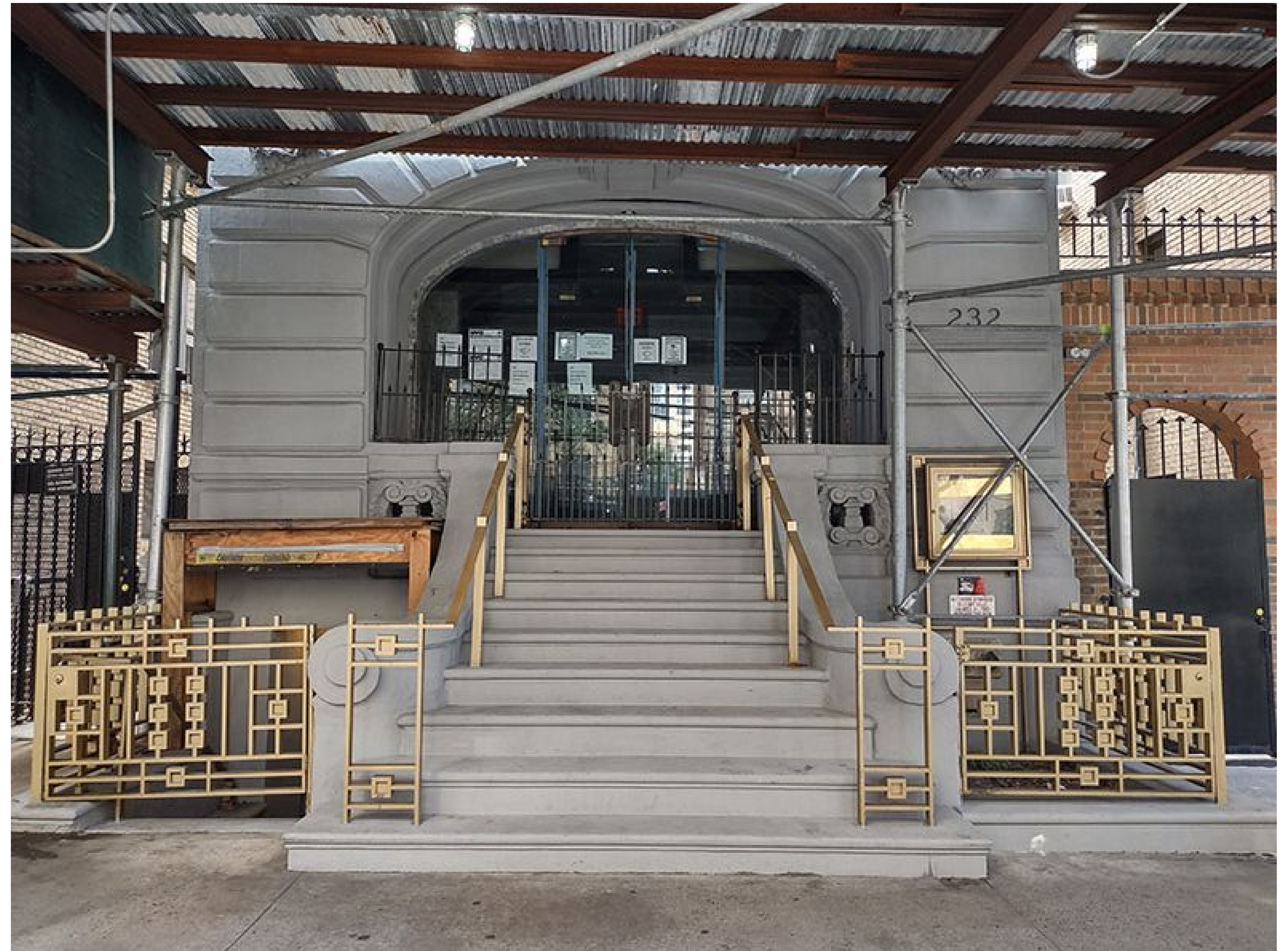
EXISTING FRONT ENTRANCE CLOSE-UP
