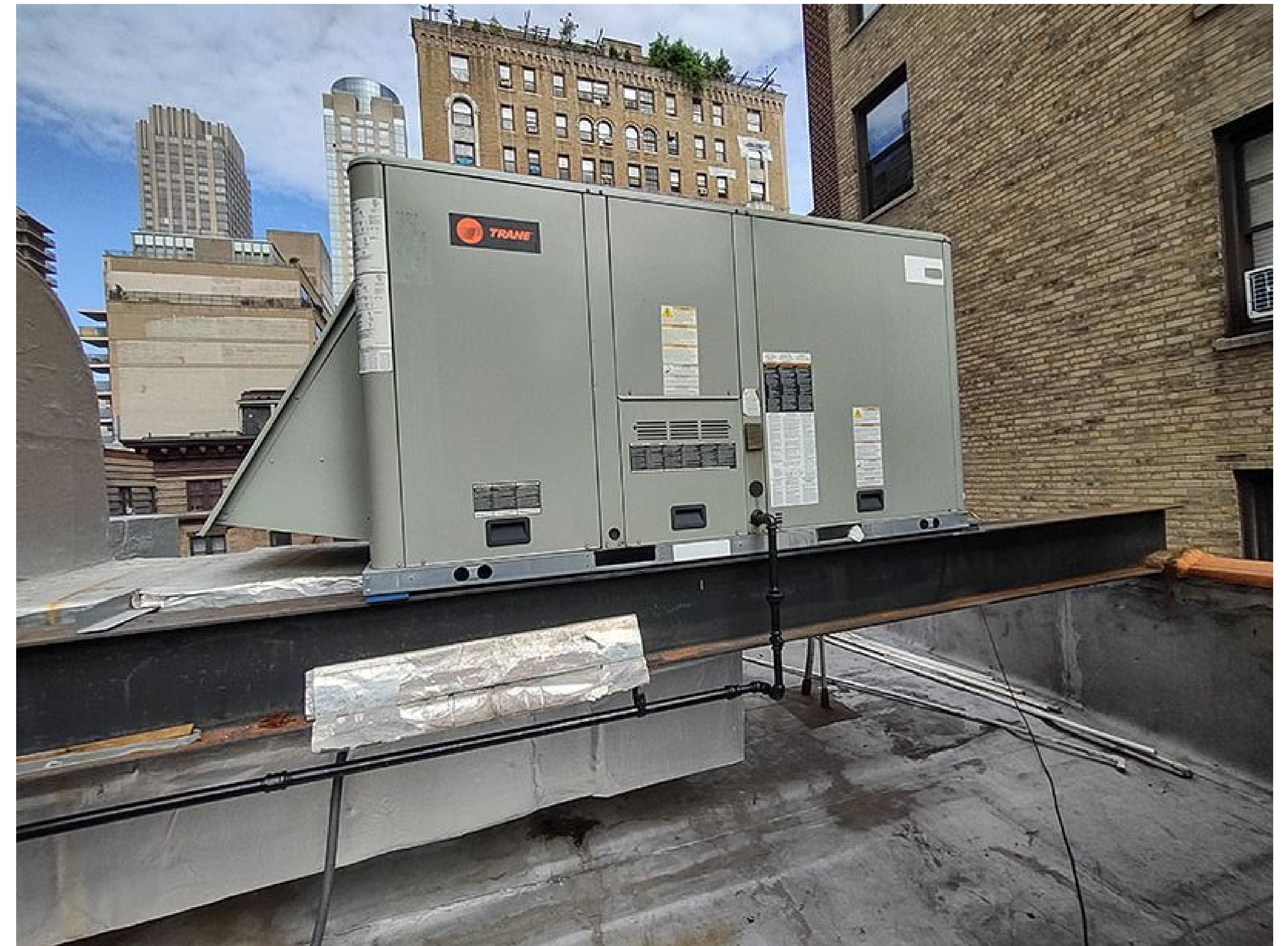
EXISTING CONDITIONS AT ROOD LOOKING EAST
