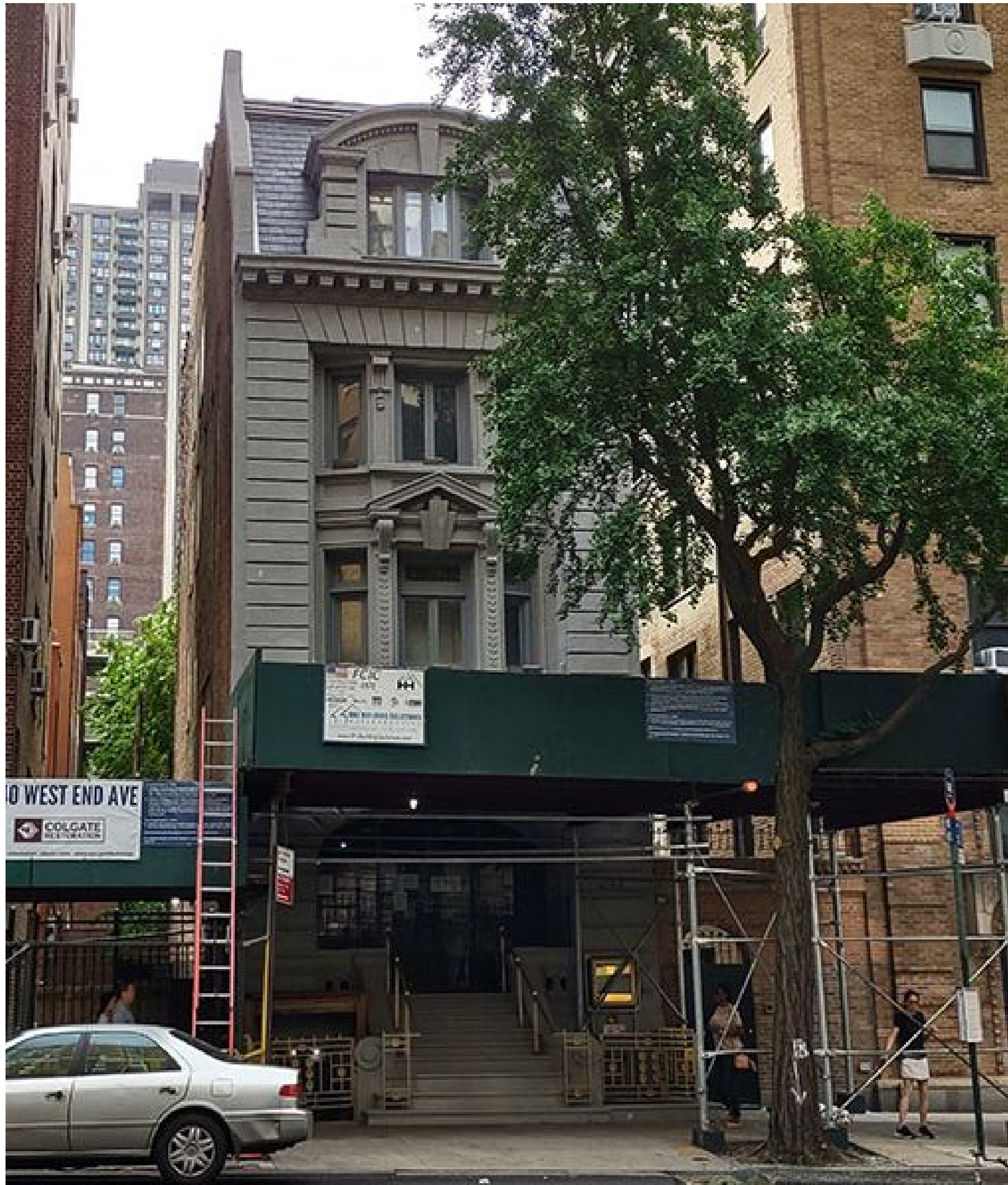
EXISTING FRONT FACADE
