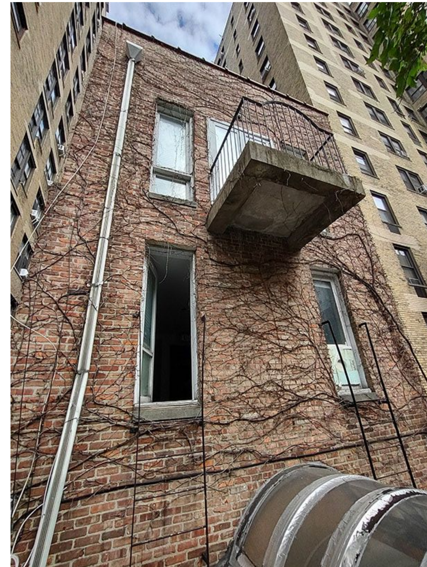
EXISTING REAR FACADE
