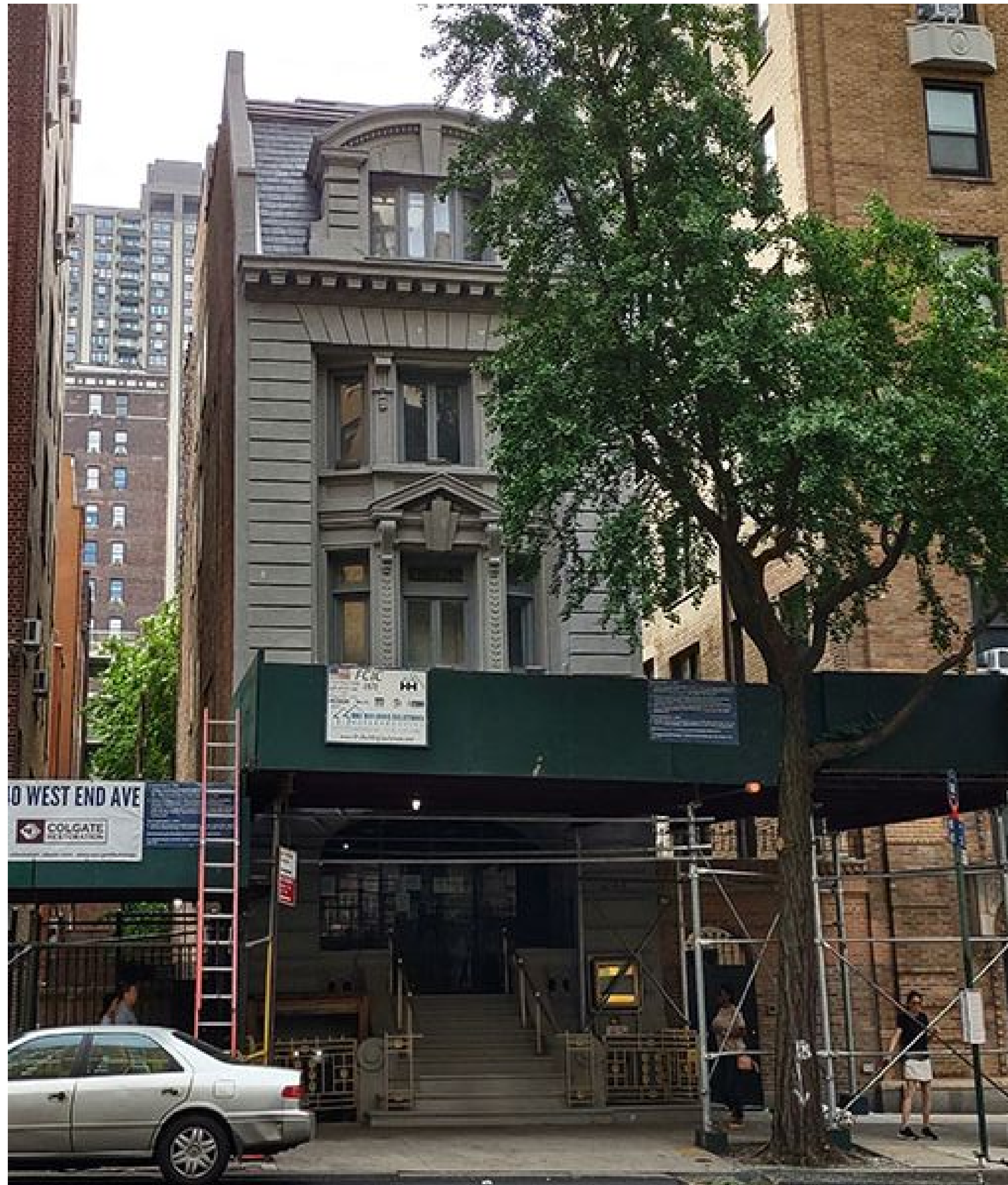
EXISTING FRONT FACADE
