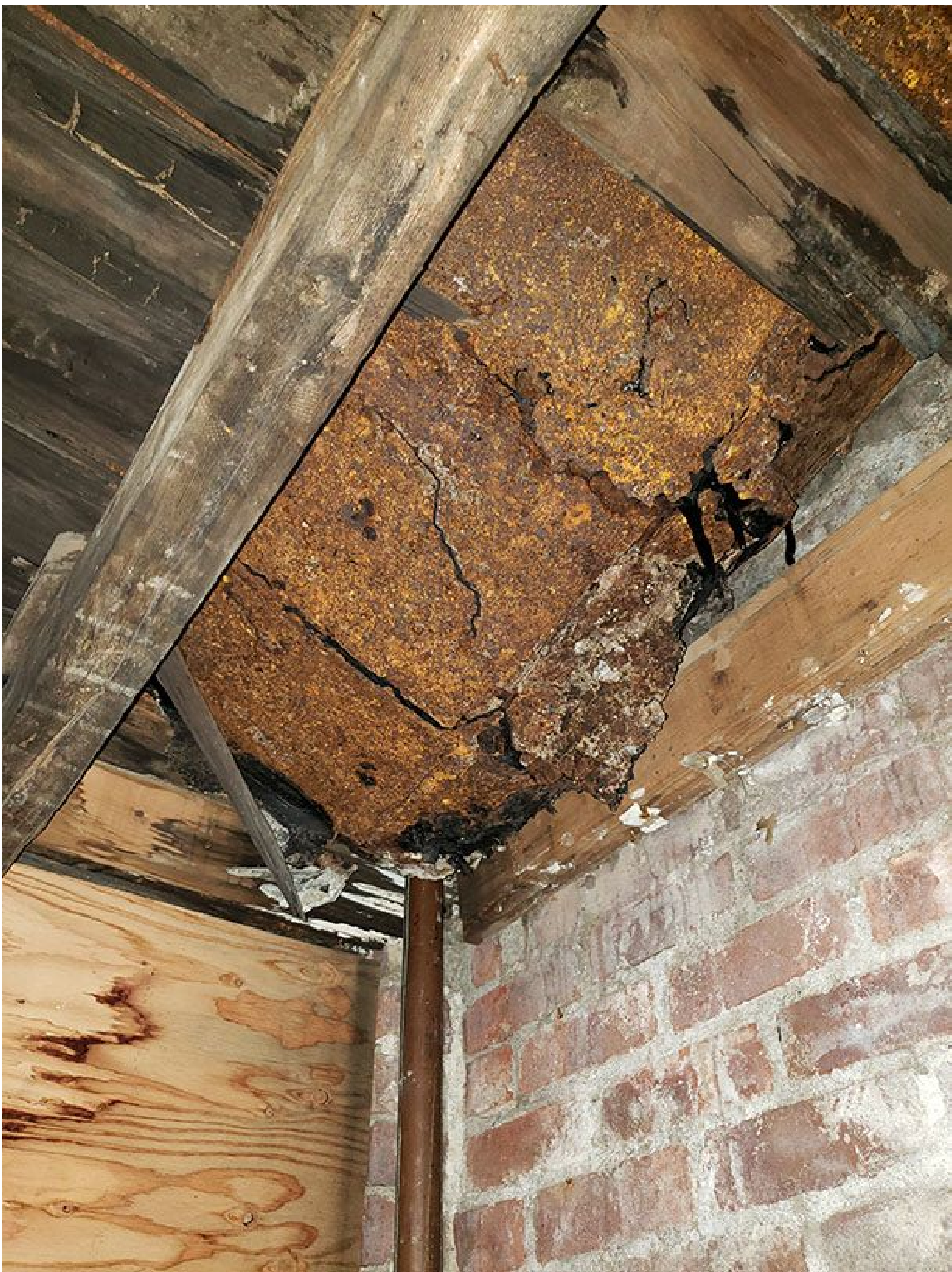
EXTERIOR LOAD BEARING WALL
