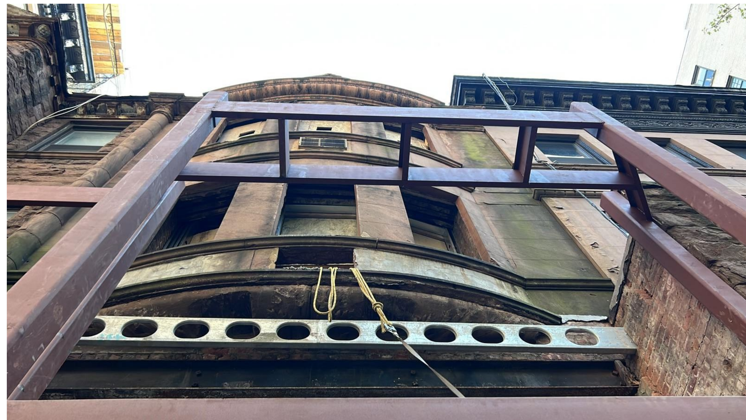
STEEL FRAME @ FRONT FACADE
