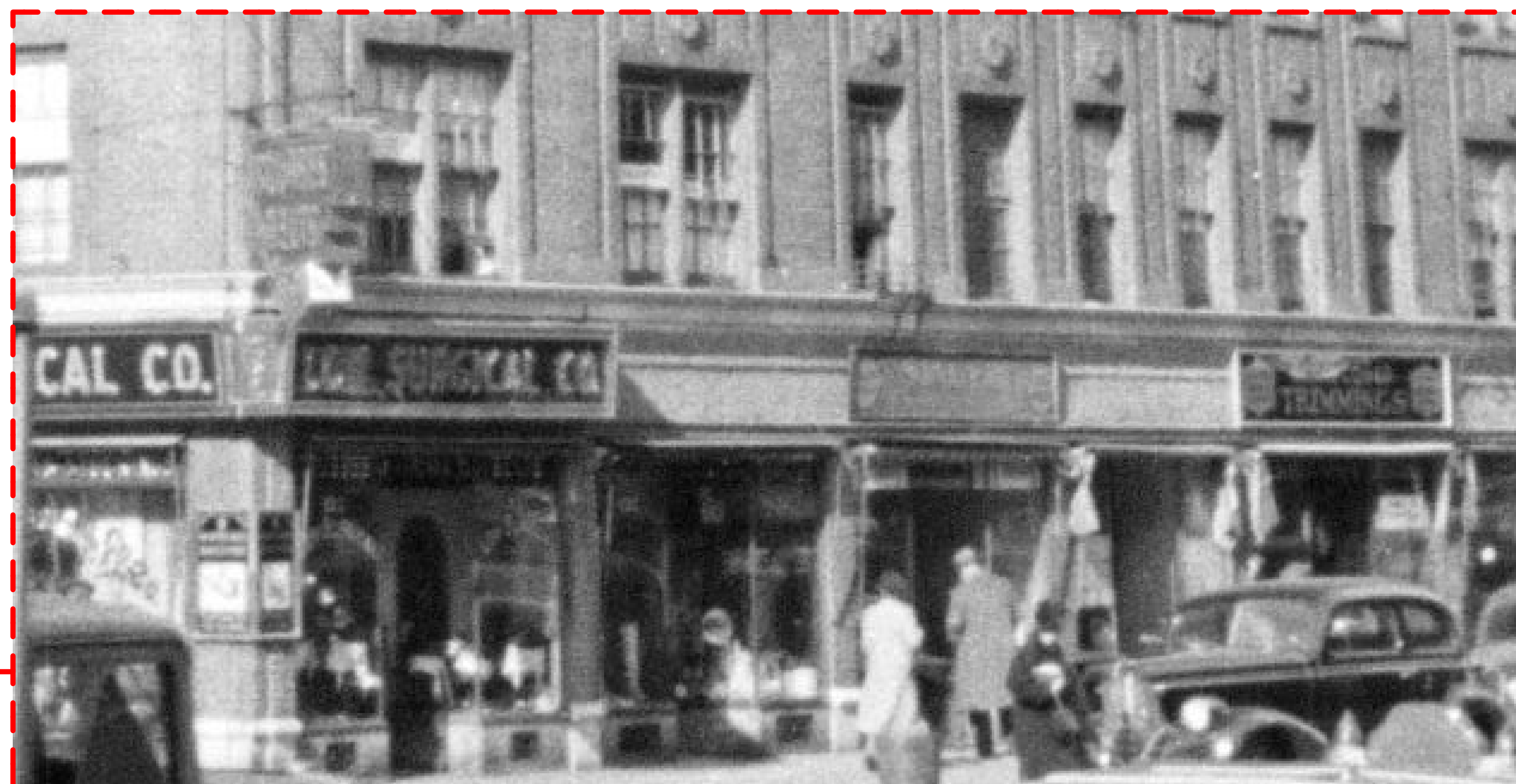
520-528 AMSTERDAM AVENUE-1940's TAX PHOTO (MUNICIPAL ARCHIVE)
